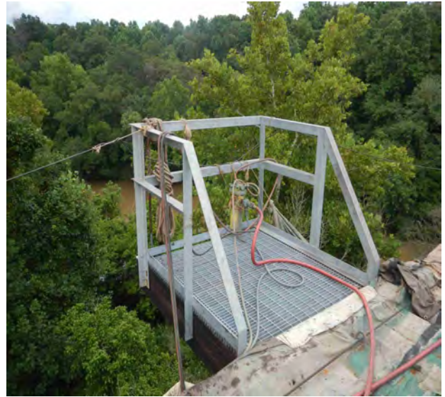
Bridge 19.30 Section 2 Typical Refuge Platform
