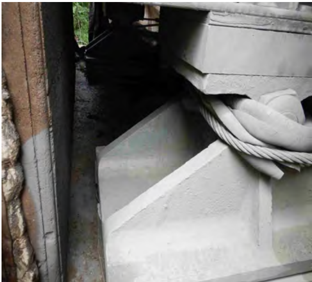
Bridge 19.30 Section 3 Abutment Bearings
