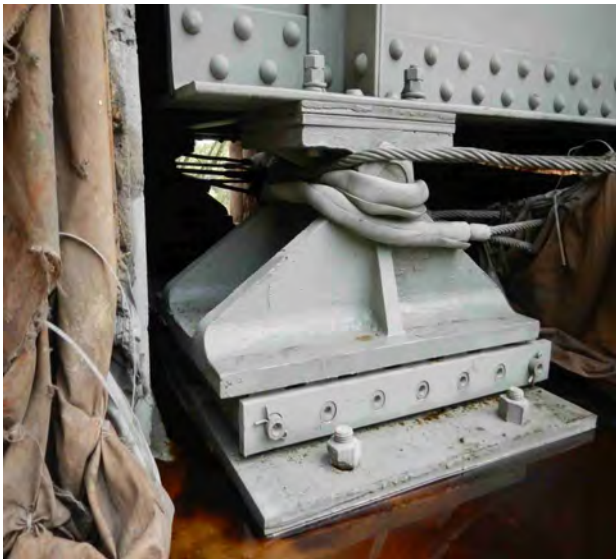
Bridge 19.30 Section 1 Typical Abutment Bearing
