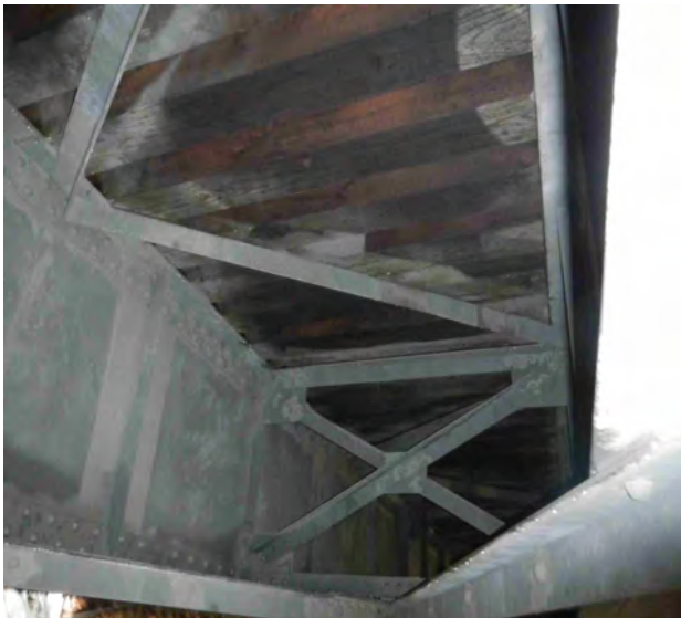
Bridge 19.30 Section 2 View of Stringer Top Lateral Bracing
