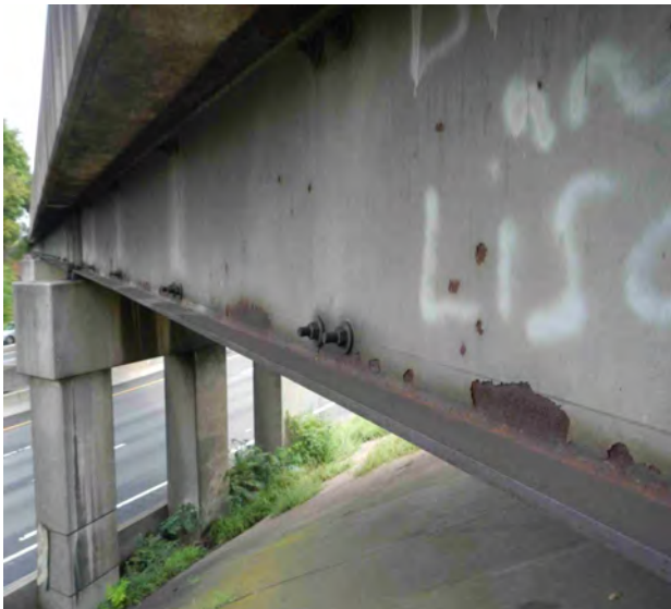
Bridge 21.50 Minor Corrosion to Beam Web at Bottom Flange Angle
