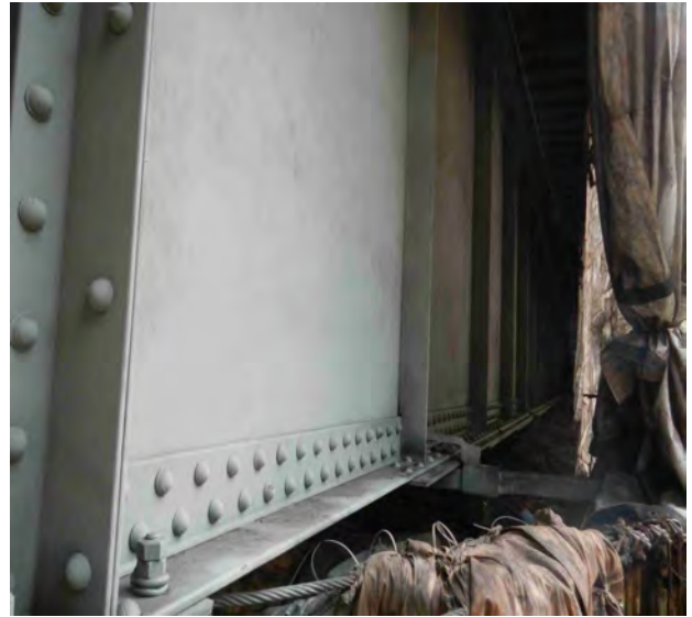
Bridge 19.30 Section 1 - New Paint on Girder
