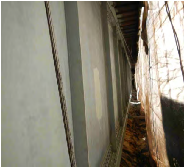
Bridge 19.30 Section 3 - New Paint on Girder
