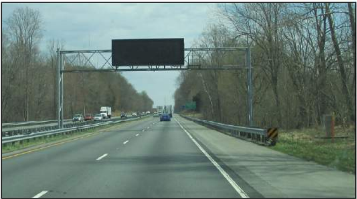
TYPICAL DMS INSTALLATION ON TRUSS STRUCTURE
