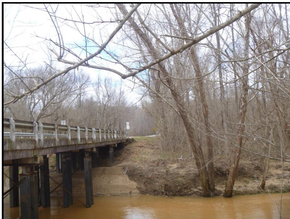
Figure 16. Bridge No. 106, facing Northwest
