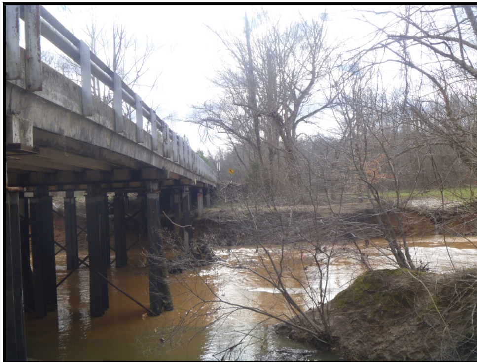
Figure 15. Bridge No. 106, facing Southeast
