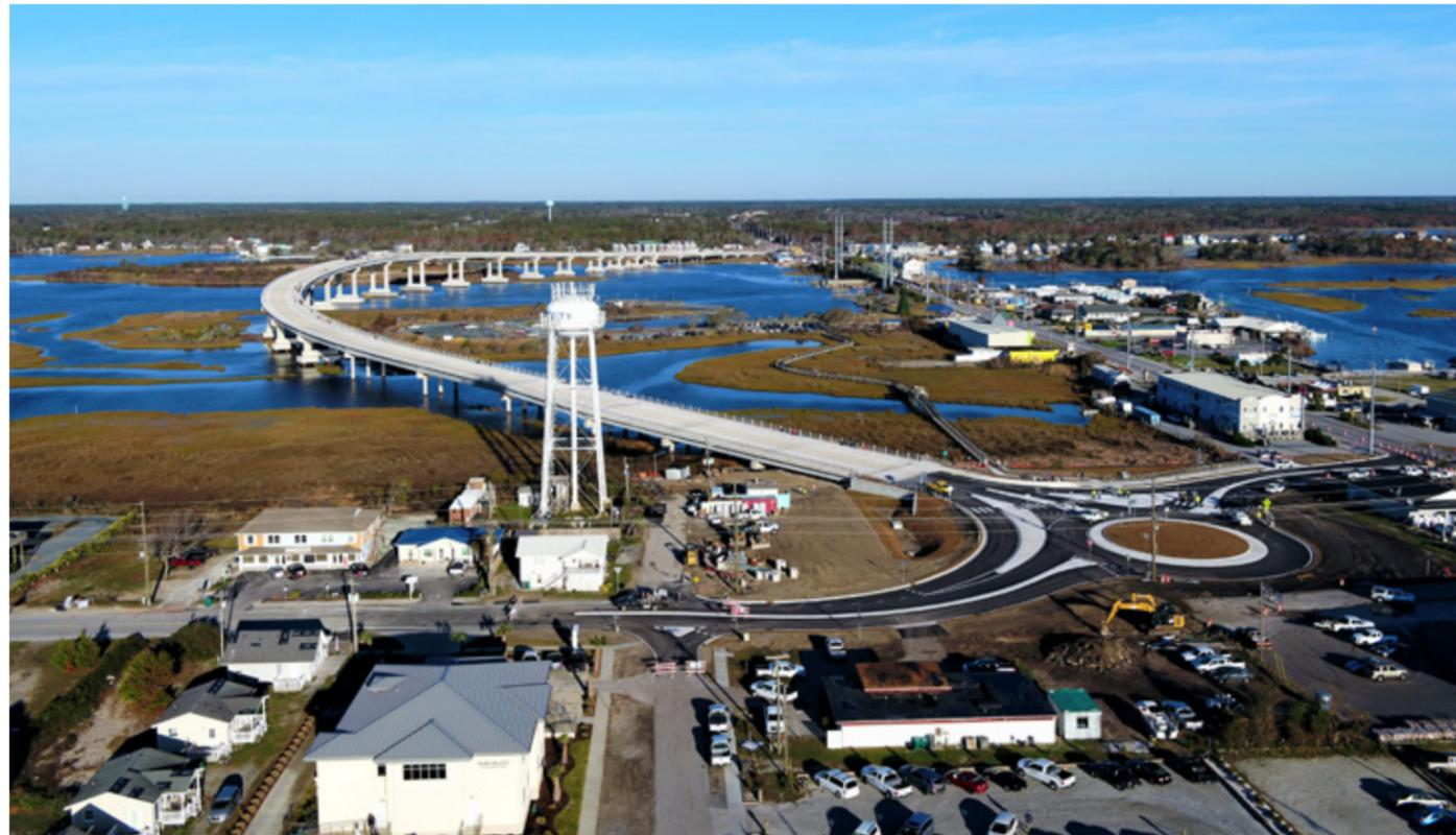
The Surf City Topsail Island Bridge Connector replaced the aging, 1950s-era steel truss drawbridge that served as a critical link between Surf City and Topsail Island. The 0.7-mile replacement bridge eliminates the chronic traffic delays from the drawbridge. It also includes roundabouts for better vehicle flow and pedestrian movement. The new bridge includes a 10-foot, multi-use path that creates a safe pedestrian route, connects the mainland to the beach, sidewalks and a park, and completes
