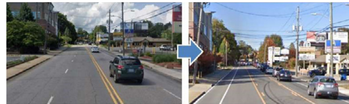
Before and After Streetview Images on Merrimon
