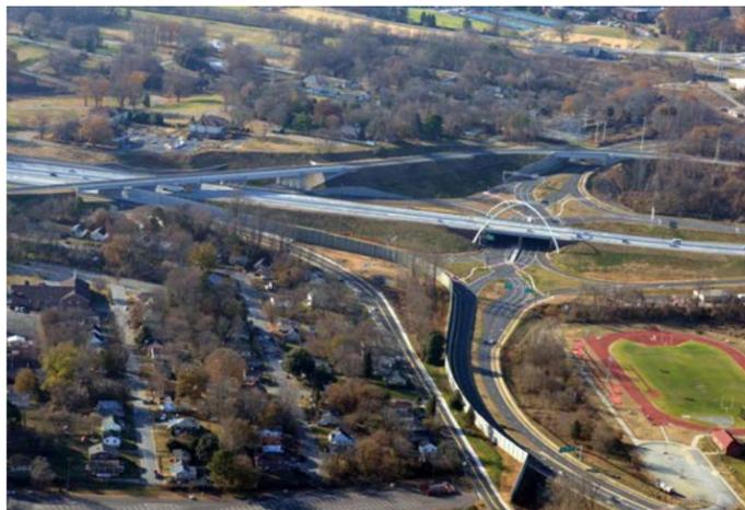
The Salem Creek Connector project is a new, 1.1-mile, four-lane median divided road with sidewalk and greenway connections connecting Martin Luther King Jr. Drive to Rams Drive at the Piedmont Triad Research Park in Winston-Salem. It opened in April 2018. This new road adds nine bridges over parts of Salem Creek and U.S. 52. Also, a new interchange was built at U.S. 52. The current interchange at Rams Drive will be removed.
