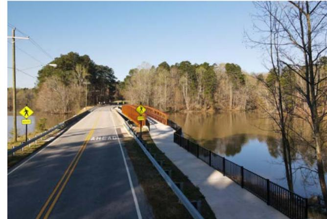
The East Fork Road Pedestrian Bridge and Sidewalk in Jamestown was completed in July 2020. The project consisted of a 200-foot pedestrian bridge and 1,266 feet of sidewalk to complete a safe pedestrian and bicyclist access to Jamestown Park and the Bicentennial Greenway. The bridge is 10 feet wide to allow for significant space for bicyclists and pedestrians to easily space out and share the facility.
