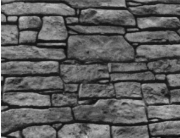
All texture is to be in addition to the nominal thickness of each element within tolerances. Relief of any texture is not to exceed a maximum depth of 2 inch.
