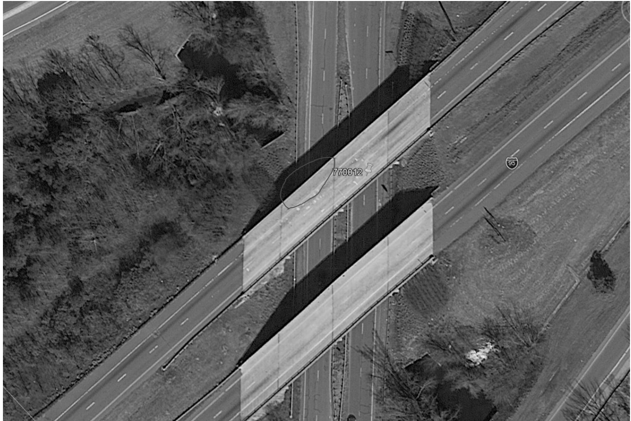
Figure 2: Beam 1 of Span 2 Location
