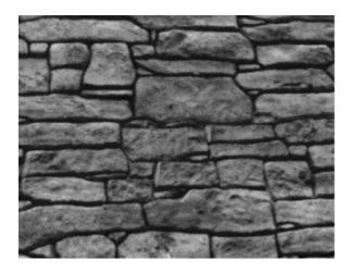
All texture is to be in addition to the nominal thickness of each element within tolerances. Relief of any texture is to have a minimum depth of  $\frac{1}{2}$ " and not a maximum depth of  $1\frac{1}{2}$ ".
