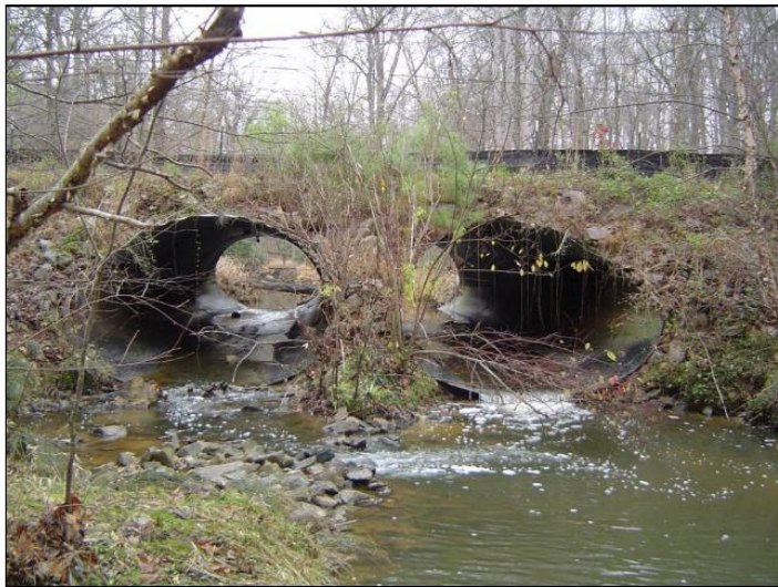
Looking upstream at existing 2@12'x7.5' CSPA
