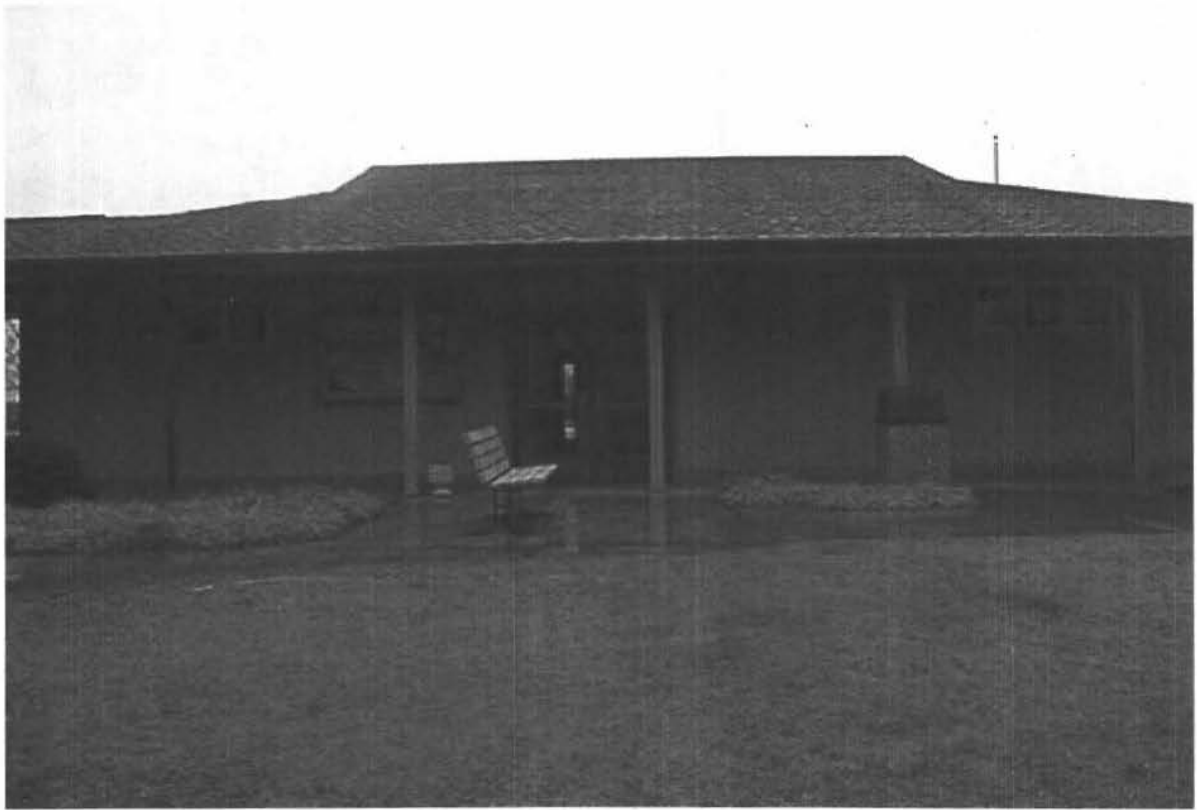
RESTROOM BUILDING FA# 15-04-02
