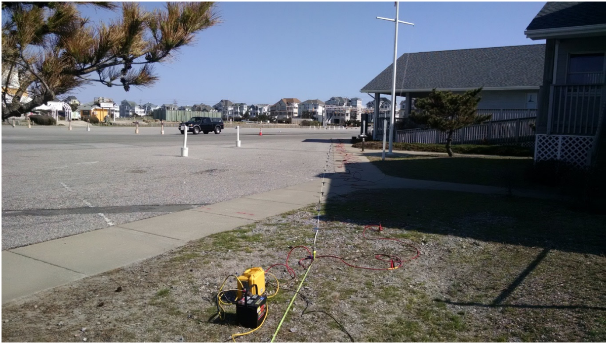
2.a. Photo looking southeast showing seismograph (yellow box) and geophone array laid out across site .
