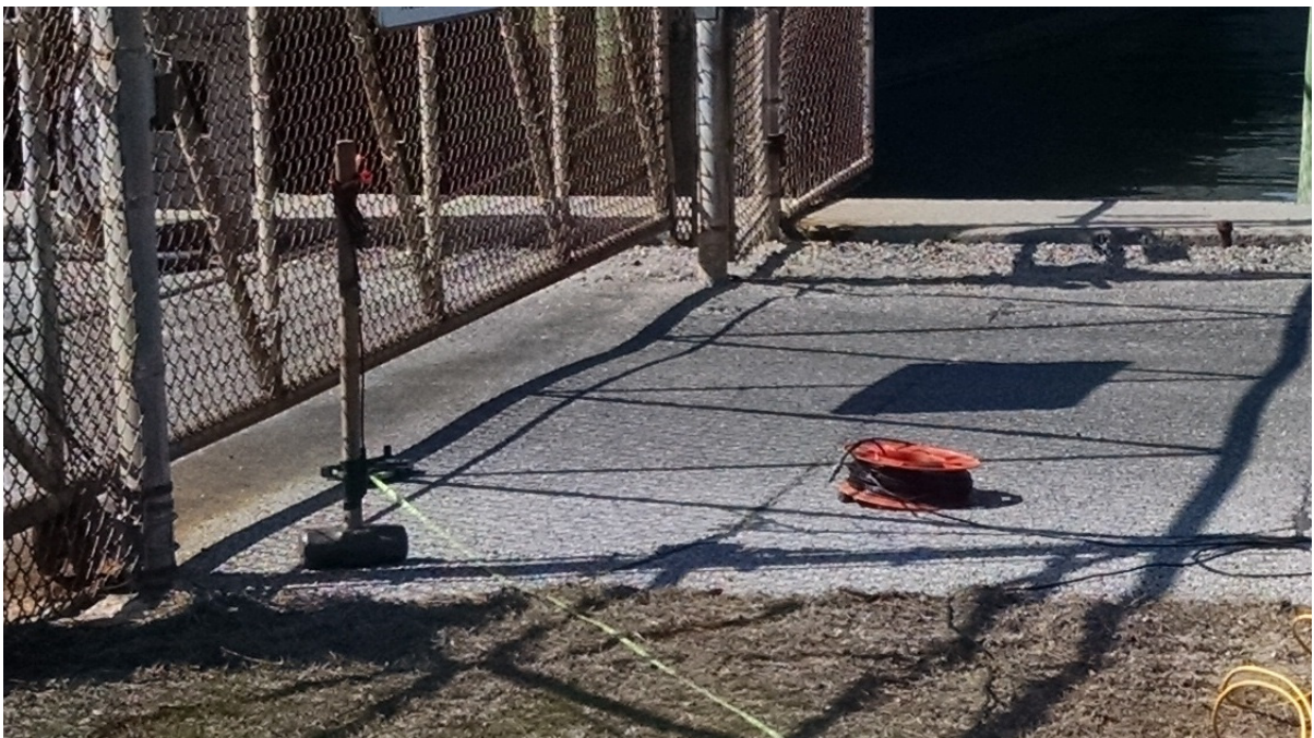
2.b. Photo showing 20-pound sledgehammer used as energy source.
