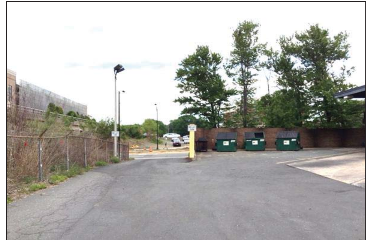
PHOTOGRAPH NO. 4: WEST APPROACH TO END BENT NO.2 ON -S1- ALIGNMENT, LOOKING EAST
