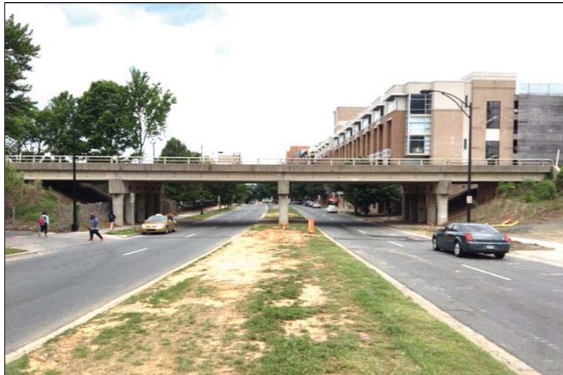
PHOTOGRAPH NO. 2: ON WEST TRADE STREET MEDIAN, SOUTHEAST OF -S2- ALIGNMENT, LOOKING NORTHWEST
