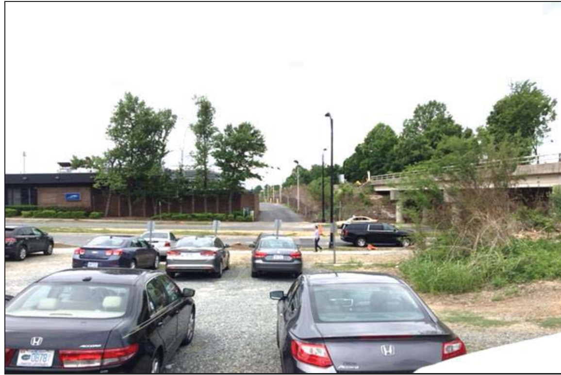
PHOTOGRAPH NO. 1: EAST APPROACH TO END BENT NO. 1 ON -S2- ALIGNMENT, LOOKING WEST
