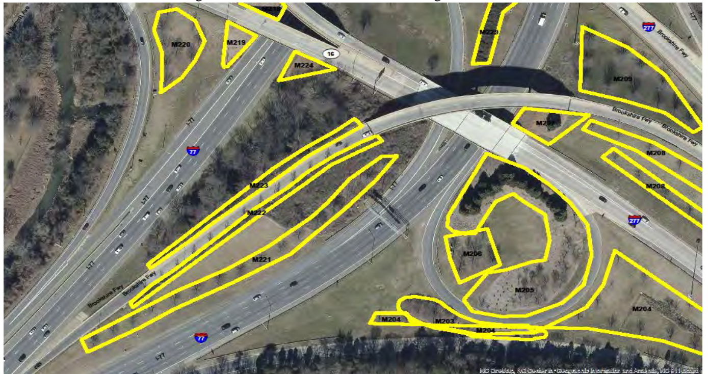
I-77 at the Brookshire Interchange, the southern section of the interchange, Exit 11
