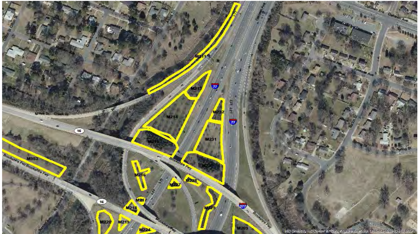
I-77 at the Brookshire Interchange, the northern section the interchange, Exit 11
