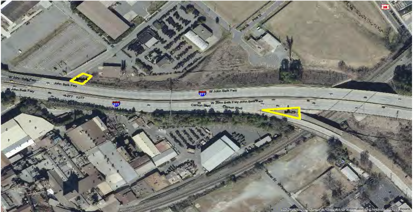
I-277, Beds from Clarkson St. to the Carson St. Exit, Exit 1D
