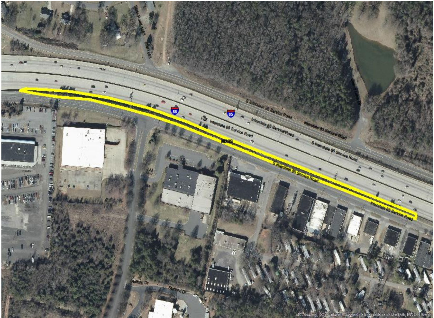
Bed between Little Rock Rd. and Billy Graham Parkway, between jersey barrier wall and control access fence
