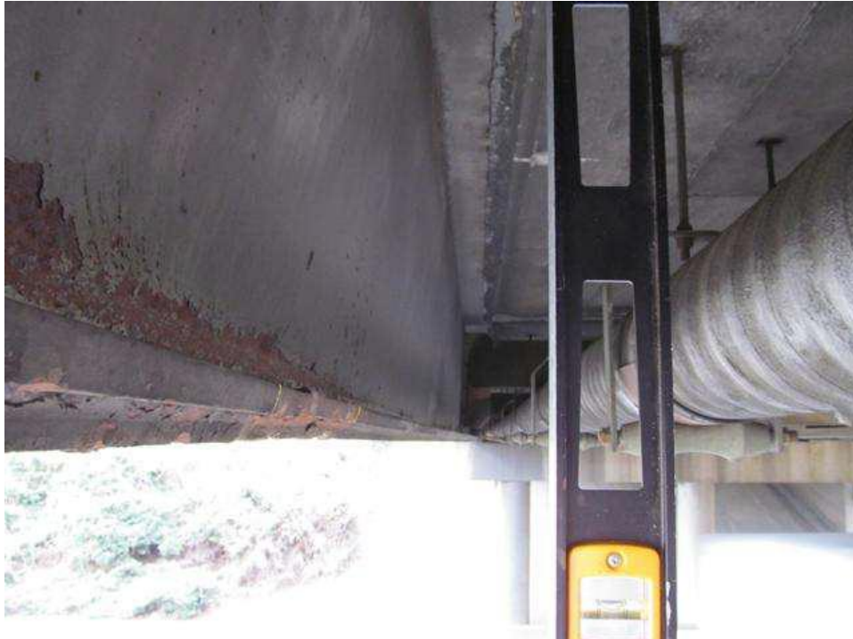
BEAM 10 IS OUT OF PLUMB ( 7 1/4" ) TO THE NORTH @ 24'-11" FROM THE FACE OF BENT 2. BEAM 10, SPAN 2
