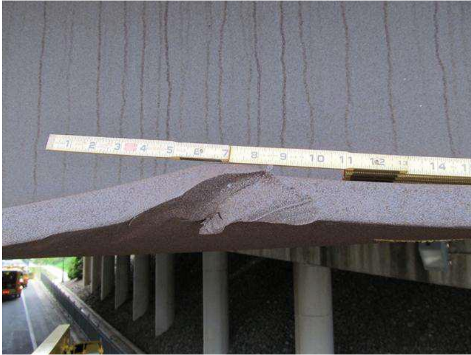
POINT OF IMPACT ON BEAM 1 IS 23'-10" FROM THE FACE OF BENT 1. INDENTATION ( 6" X 3/4" ) AND GOUGE ( 5" X 1" X 1/8" ) IN FLANGE. FLANGE IS BENT UPWARD ( 1 1/2" ).
