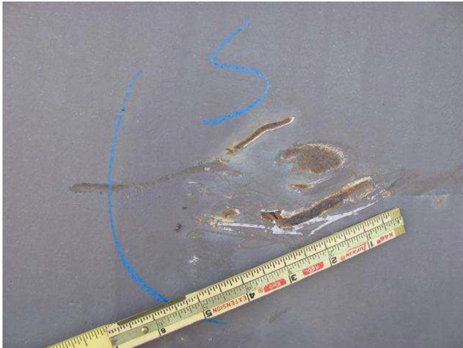
GOUGE IN WEB 3" X 1/2" X 1/32" +/- DEEP AT 4'-0" FROM ABUT 2
