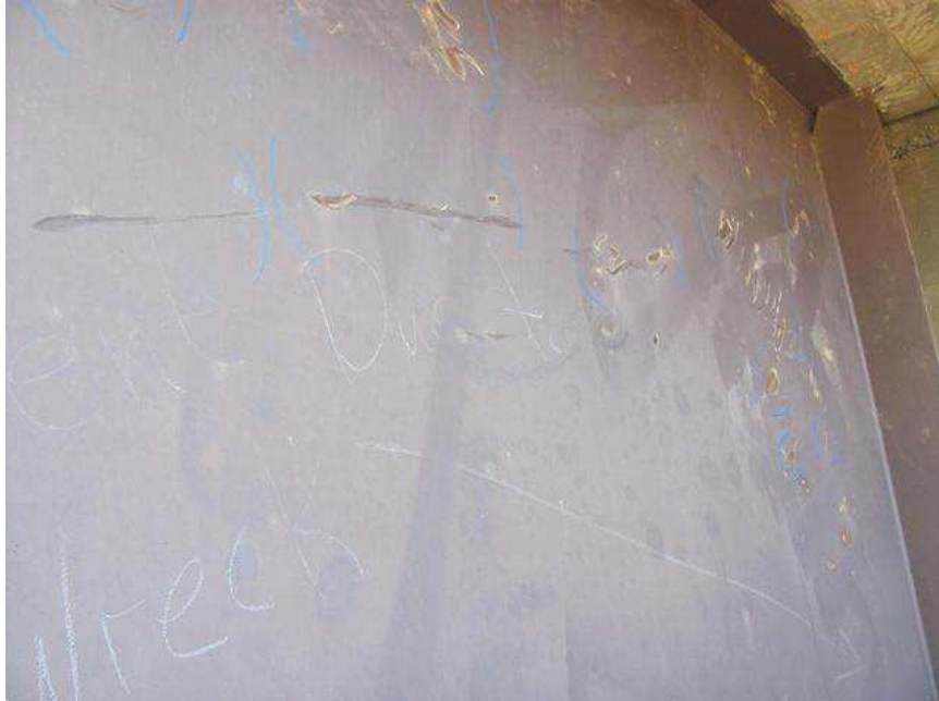
DAMAGE IN WEB 8'-0" FROM ABUT.2
