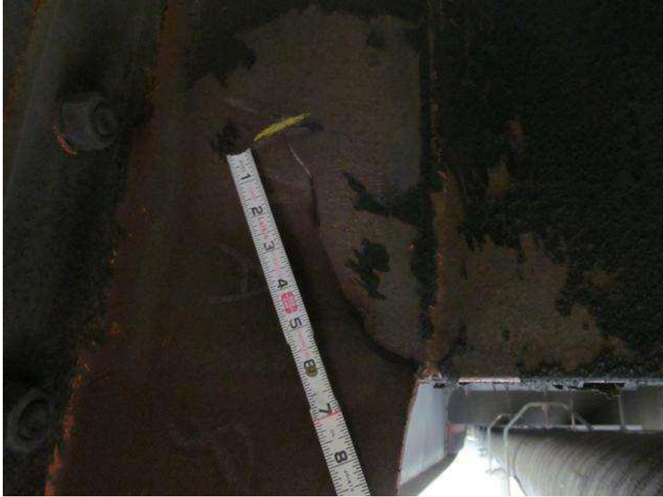
DIAPHRAGM BRACKET HAS A 7 INCH LONG CRACK IN IT ON THE WEST SIDE. BEAM 10, SPAN 2
