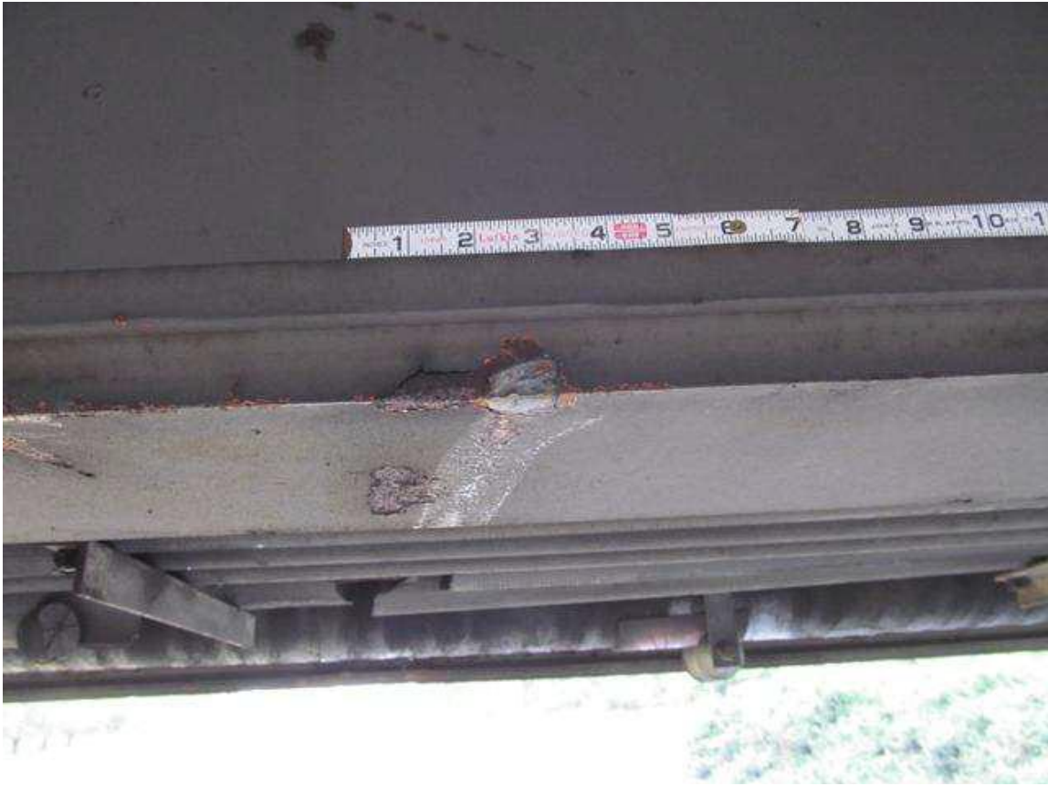
POINT OF IMPACT ON BEAM 9 IS 24'-7" FROM THE FACE OF BENT 2.
