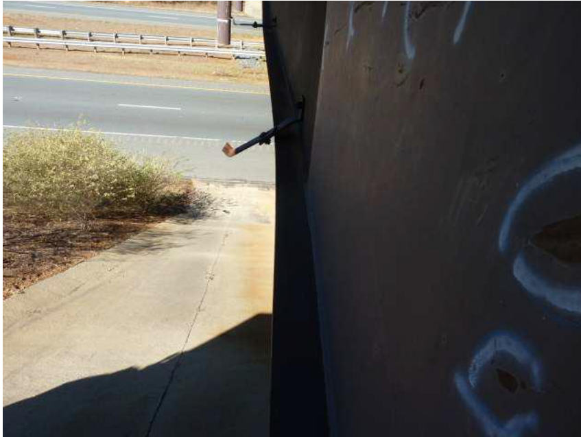
UP TO 3 1/2" OUT OF PLANE BENDING DUE TO IMPACT DAMAGE IN BOTTOM FLANGE AND WEB OF GIRDER 8 IN SPAN 2 EXTENDING 15' FROM END BENT 2
