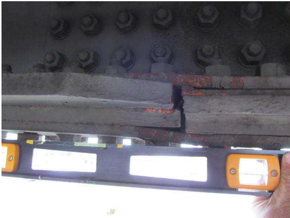
SPLICE PLATE IS BENT 3/8" OUT OF PLUMB. BEAMS ARE SEPERATED 3/4" APART @ 18'-4" FROM THE FACE OF BENT 2. BEAM 10, SPAN 2
