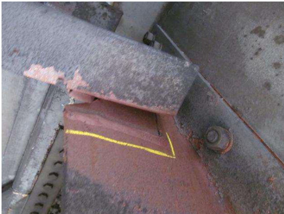
BOTTOM AND END WELD ON BEAM 10 IS BROKEN LOOSE @ 20'-8" FROM THE FACE OF BENT 2. BEAM 10, SPAN 2
