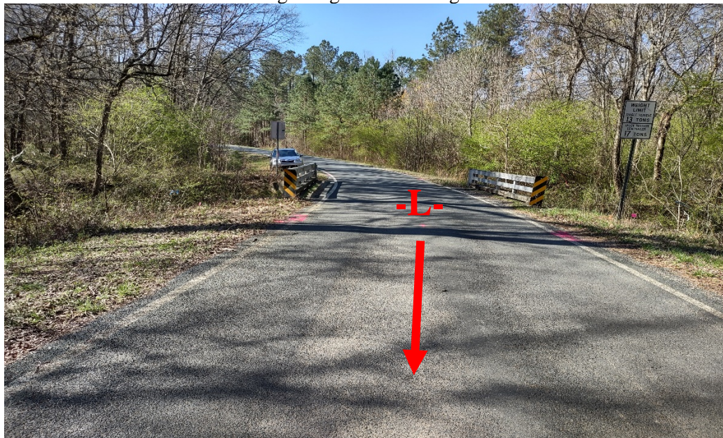
View of Along Bridge 231 Looking Downstation
