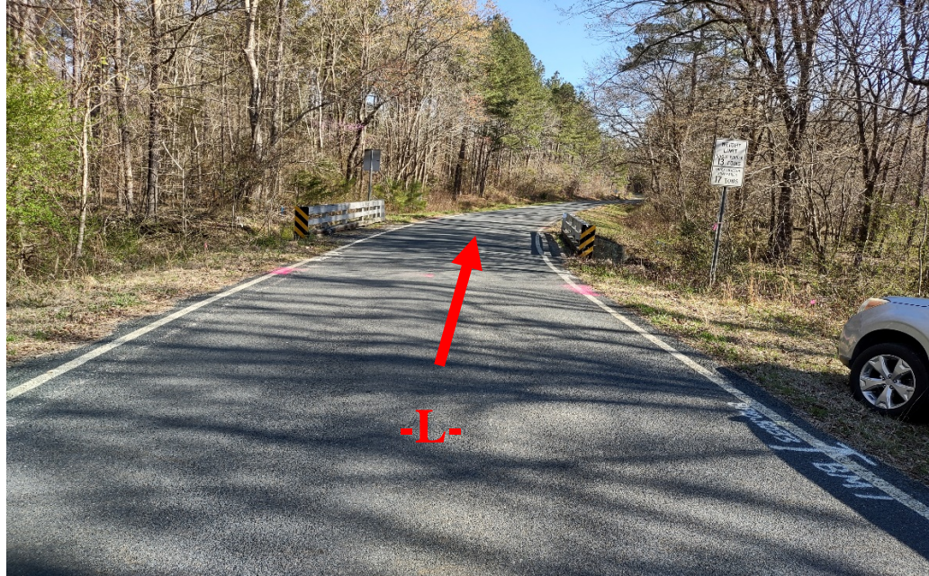
View Along Bridge 231 Looking Upstation
