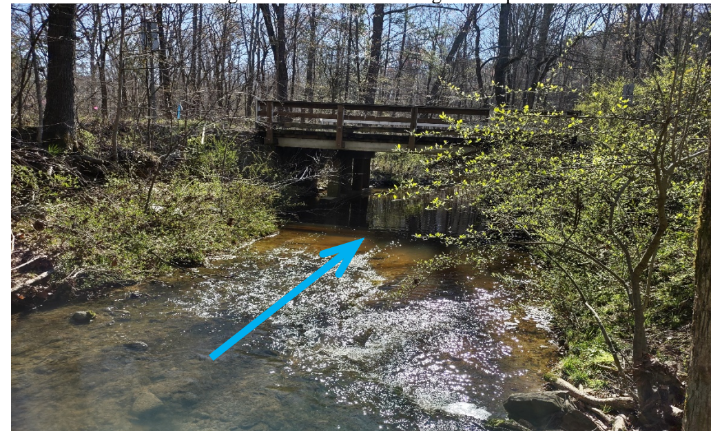
View Looking Downstream from Bridge 231 Upstream Side
