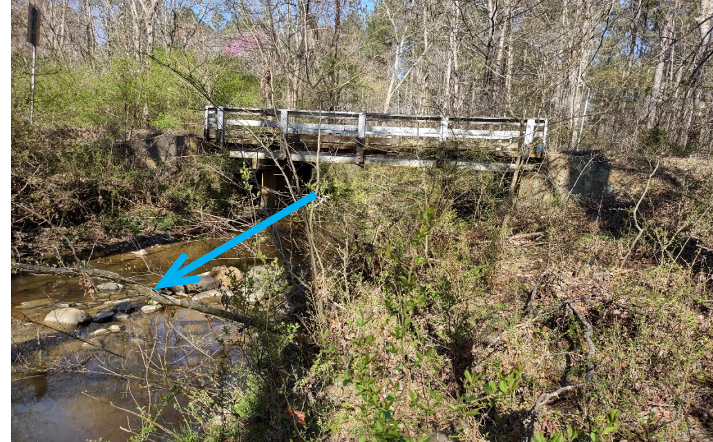
View Looking Upstream from Bridge 231 Downstream Side
