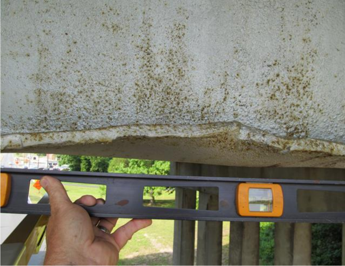
FLANGE BENT UPWARD 2 1/2" @ 14'-9" FROM THE FACE OF BEAM #1 OF SPAN# 2
