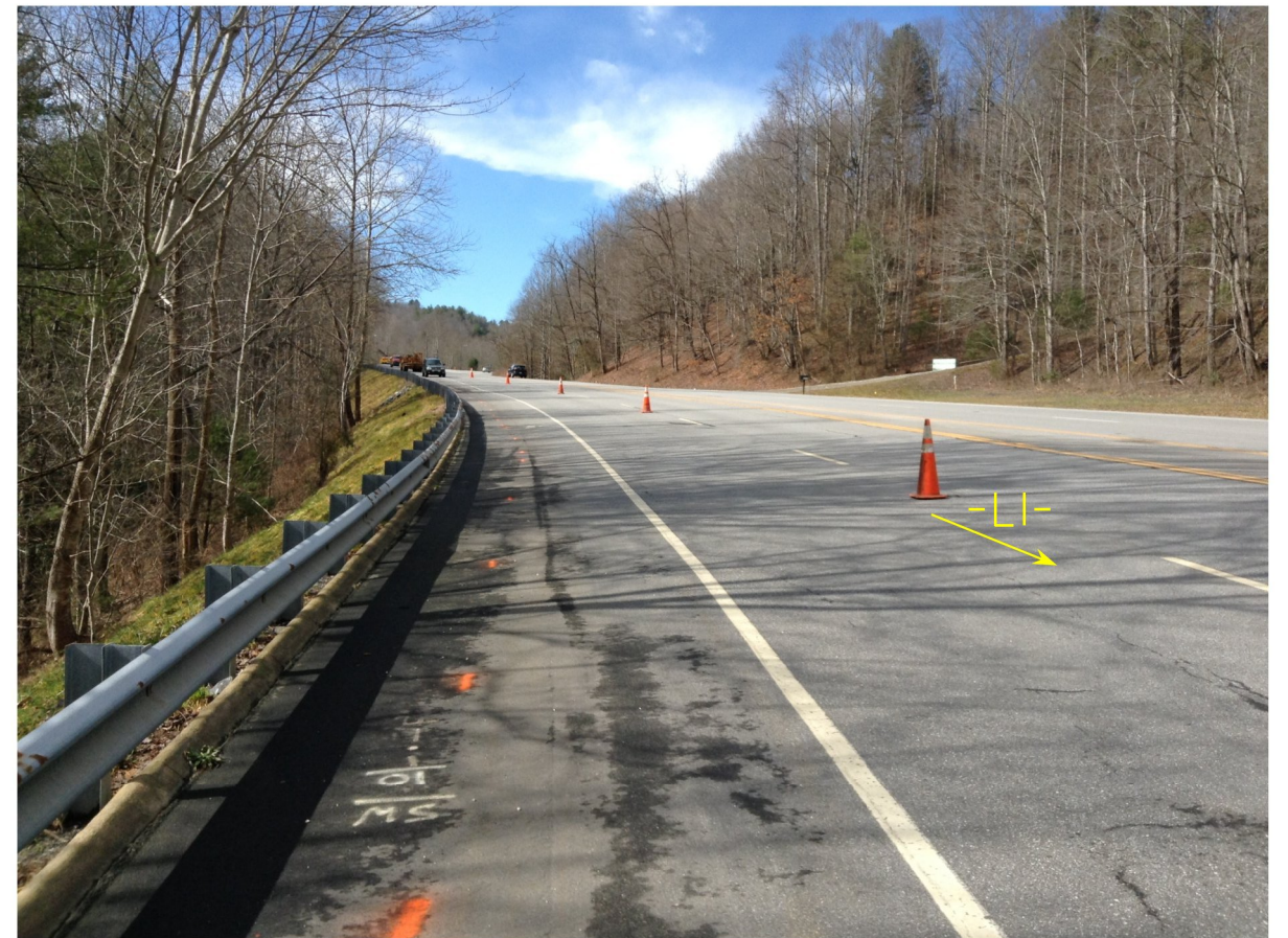
Boring W-6, looking north on US 421
