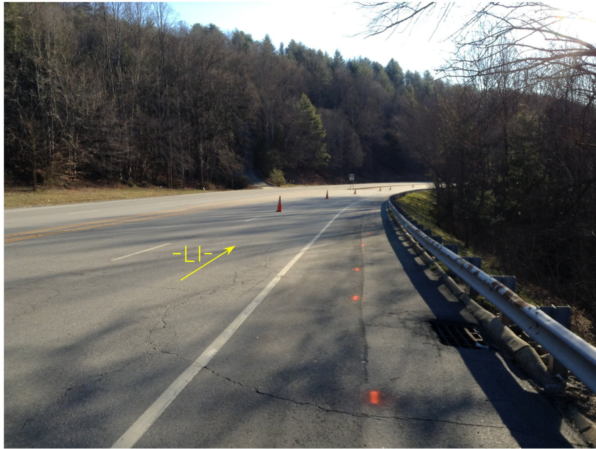
Boring W-4, looking south on US-421
