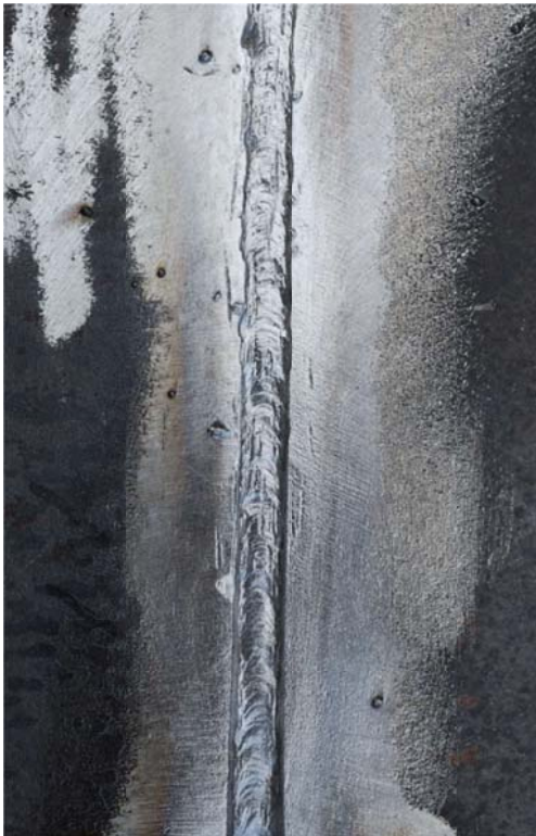
Typical appearance after cleaning first pass.
