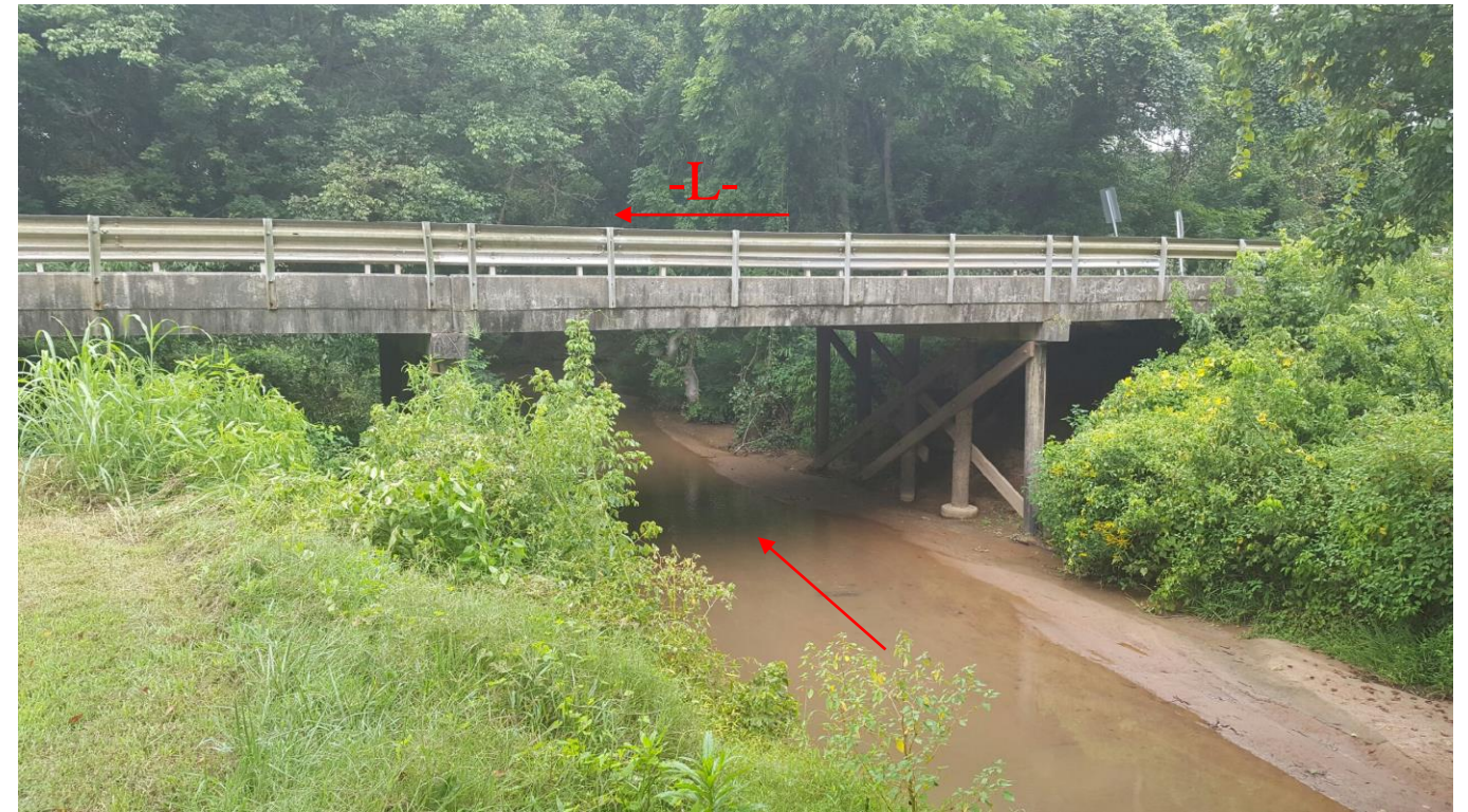
Photograph No. 2: Looking Downstream
