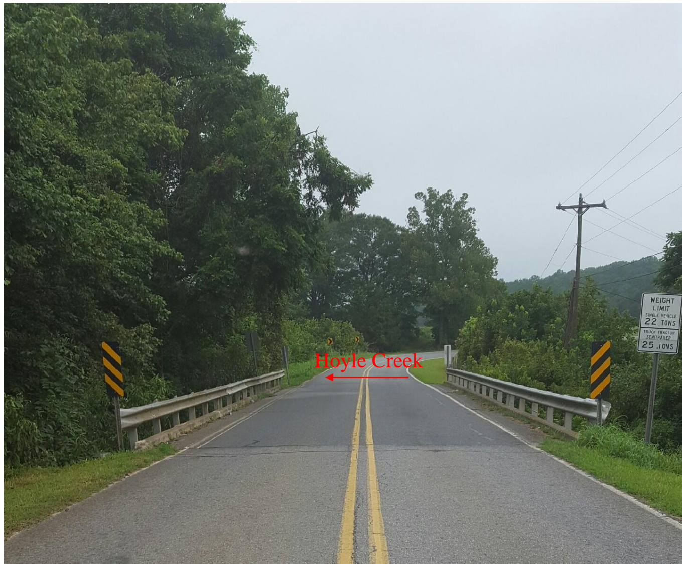
Photograph No. 1: At End Bent 2 looking towards End Bent 1
