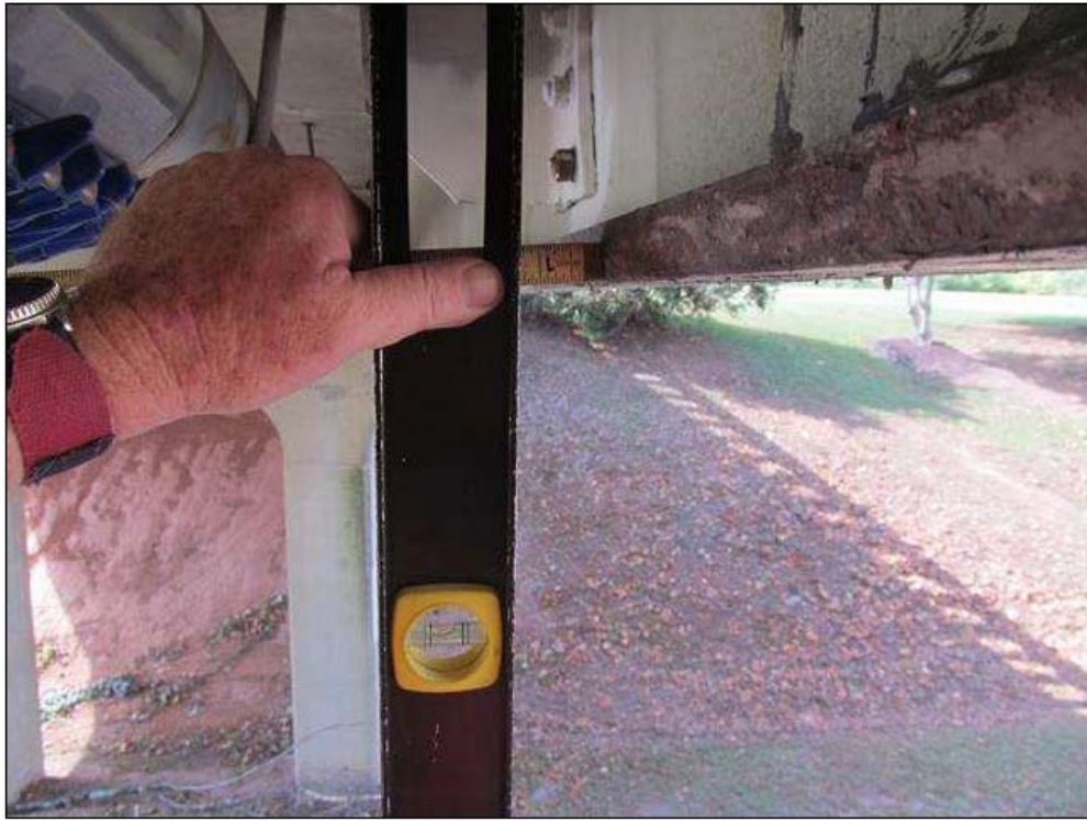
BEAM 1, BENT OUT OF PLUMB 1.5"
