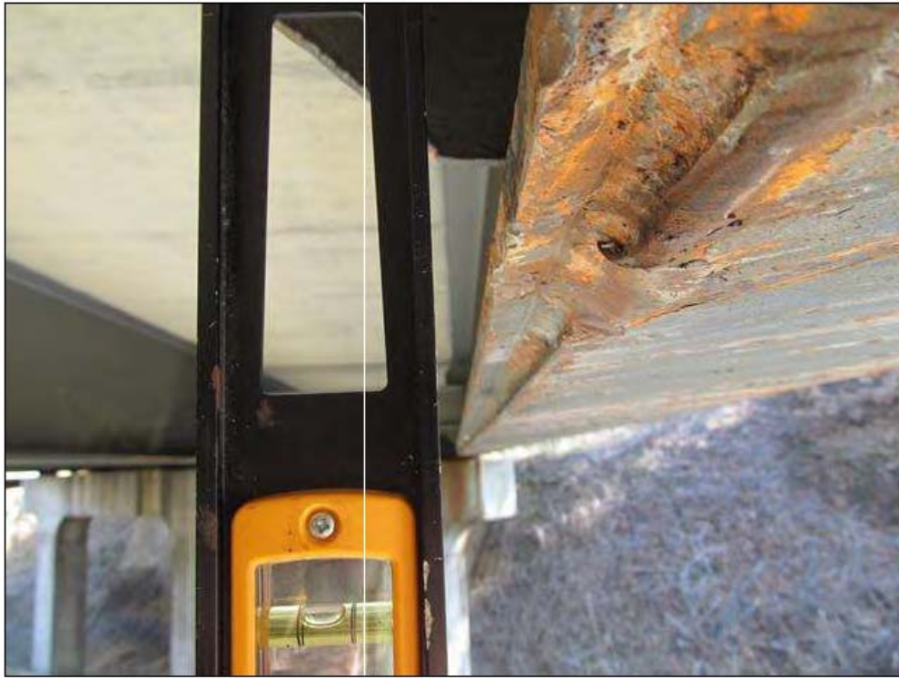
BEAM 1 IS OUT OF PLUMB ( 5/8" +/- ) TO THE NORTH @ 21'-4" FROM THE FACE OF BENT 2. BEAM 1, SPAN 2
