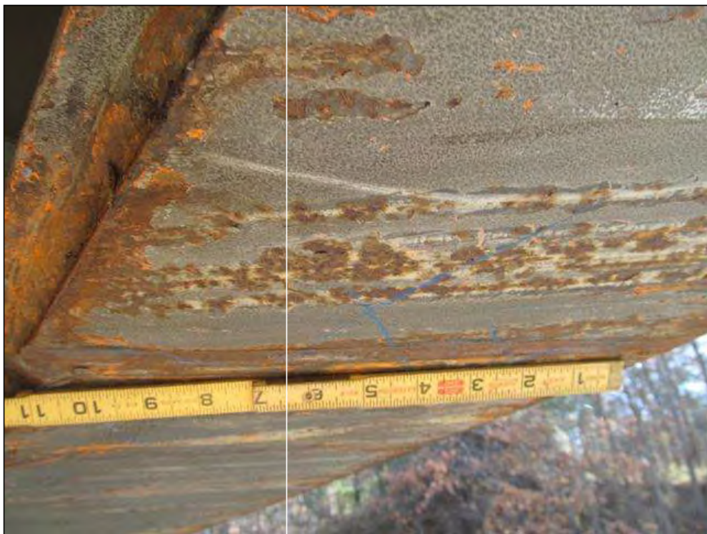
GOUGE IN COVER PLATE ( 12" X 3/4" X 1/16" ) @ 20'-7" FROM THE FACE OF BENT 2. BEAM 1, SPAN 2. ( NBL )
