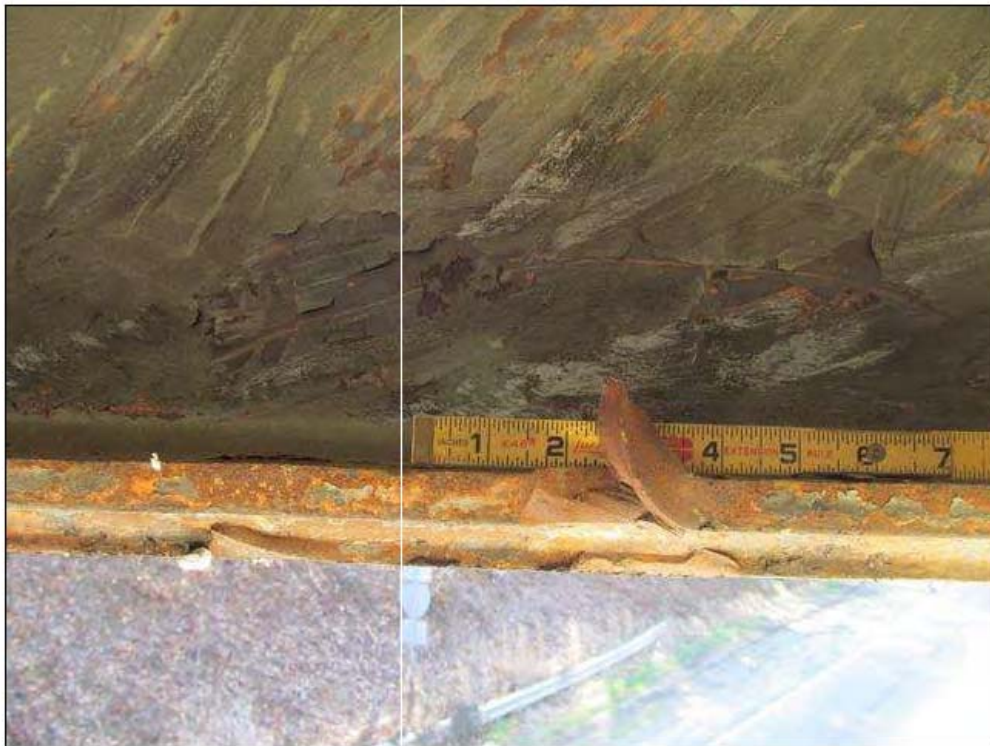
POINT OF IMPACT ON BEAM 1 IS 18'-9" FROM THE FACE OF BENT 2. INDENTION IN FLANGE ( 2" X 1/2" ) & COVER PLATE ( 2" X 1/16" ). BEAM 1, SPAN 2. NBL
