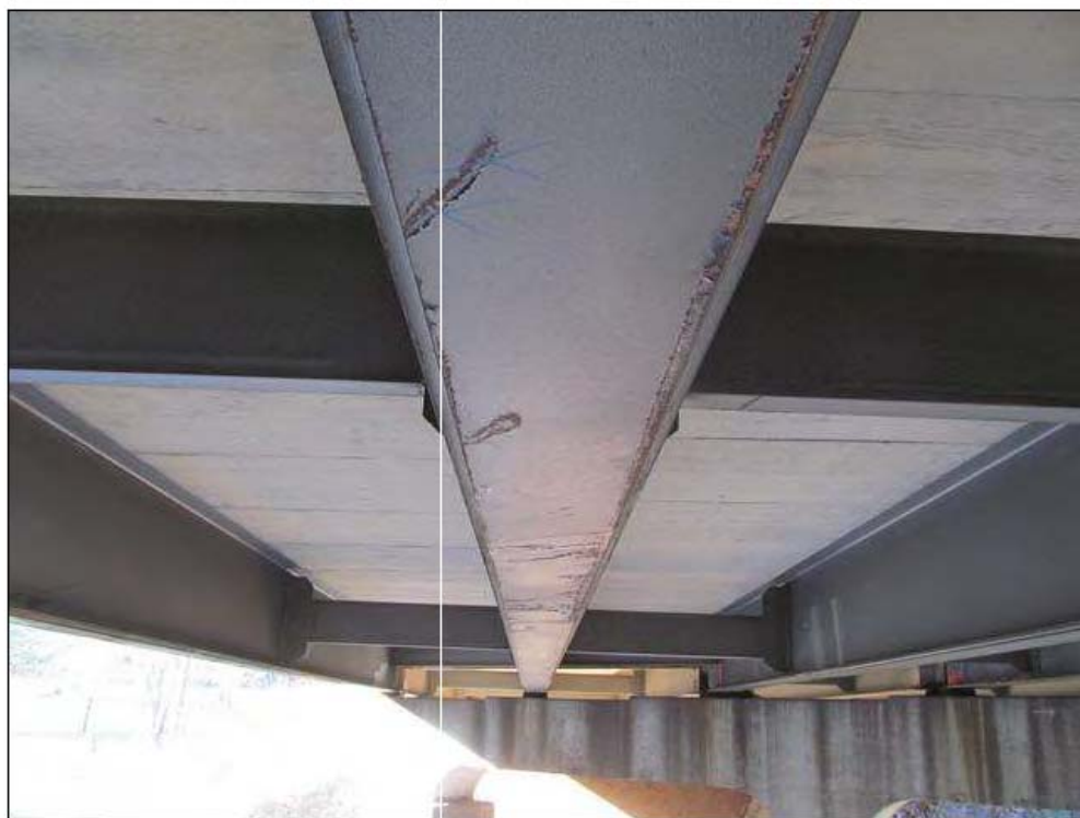
SCRAPES ON BOTTOM OF COVER PLATE OF BEAM 2 IN SOUTH BOUND LANE. BEAM 2, SPAN 2. ( SAME IN NORTH BOUND LANE )
