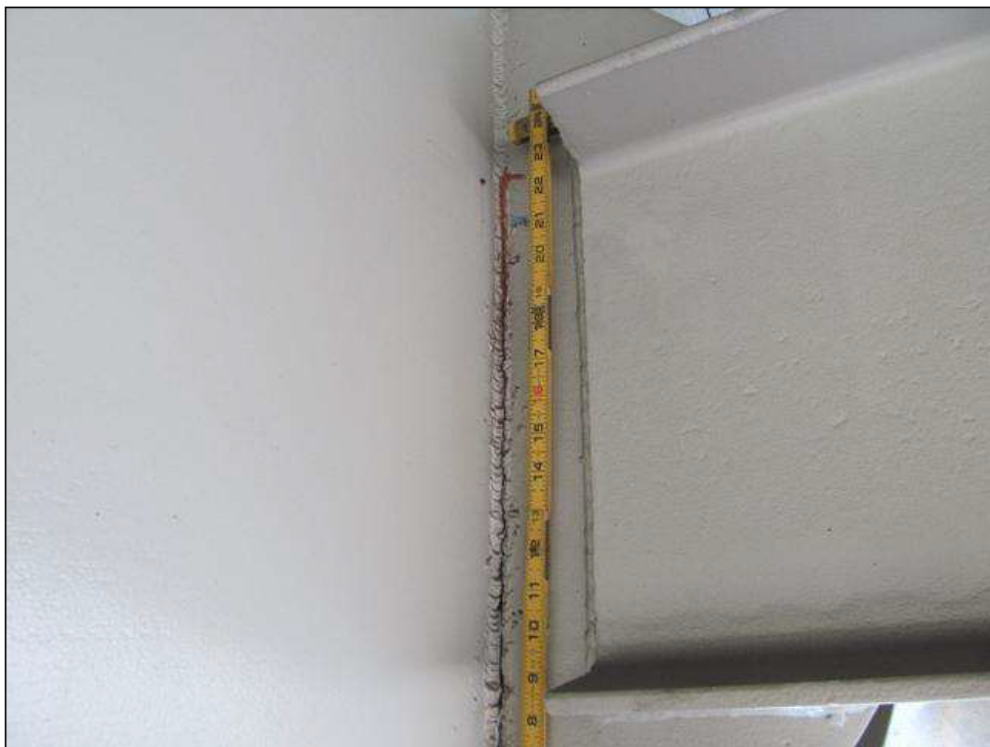
A 23" CRACK IN DIAPHRAGM WELD AT DIAPHRAGM ON BEAM 5 AT 14'-2" FROM BENT 1
