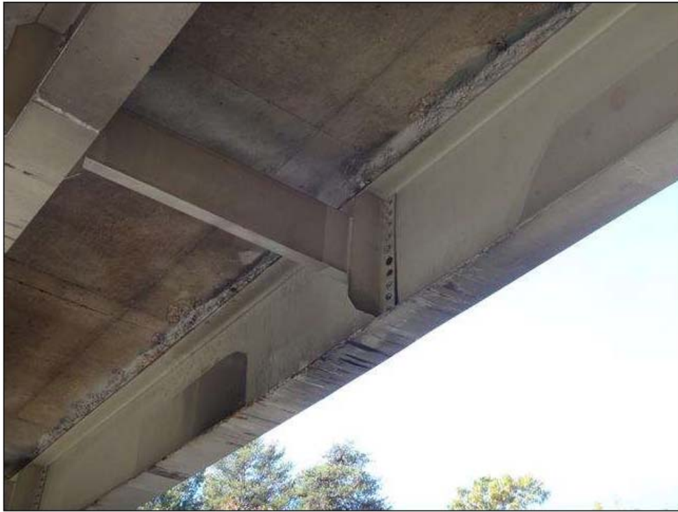
SPAN 3 BEAM 1 WEB AND BOTTOM FLANGE AT 20FT FROM BENT 3, IMPACT DAMAGE (12LF), OUT OF PLUMB (UP TO +/- 3IN)
