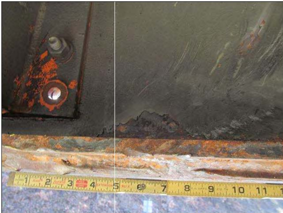
INDENTATION IN COVER PLATE ( 8" X 1/16" ) & FLANGE ( 10" X 1/8" ) AT 20'-7" FROM THE FACE OF BENT 2. BEAM 1, SPAN 2. ( NBL )
