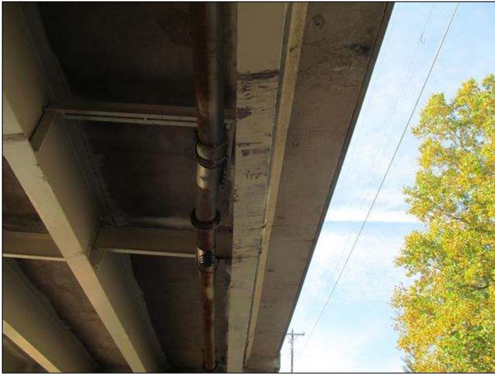
LOOKING UP AT BEAM 1 IMPACT AREA
