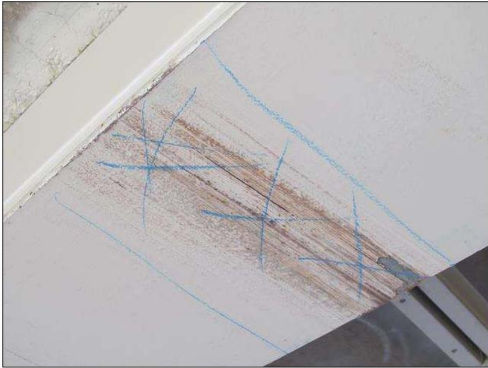
BEAM 2, @ 13.583' OUT FROM BENT 2 BEARING, SCRAPE MARKS.
