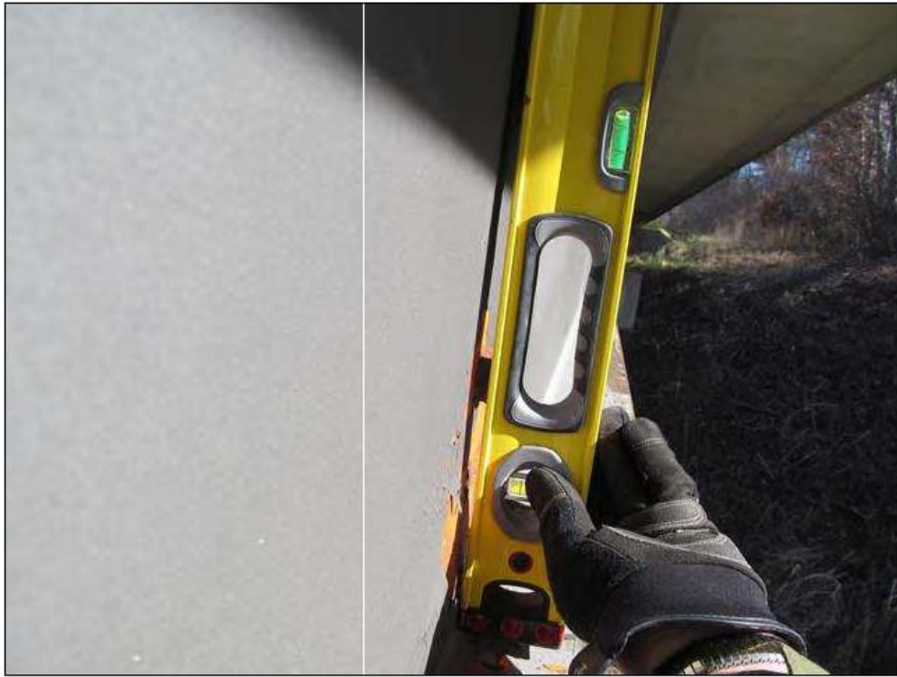
BOW IN BEAM 1 ( 3/8" ) @ 21'-4" FROM THE FACE OF BENT 2. BEAM 1, SPAN 2
