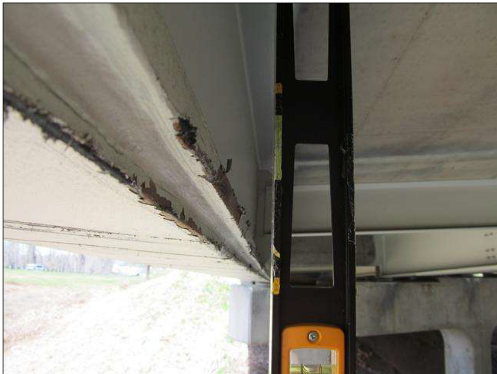
BEAM 5 IS 1 1/2" OUT OF PLUM AT 24'-9" FROM FACE OF BENT 1
