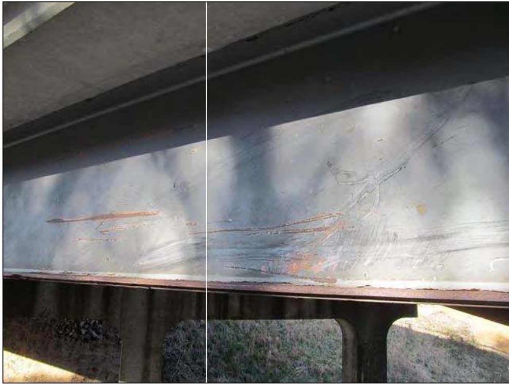
SCRAPES ON THE OUTSIDE OF BEAM 1, SPAN 2
