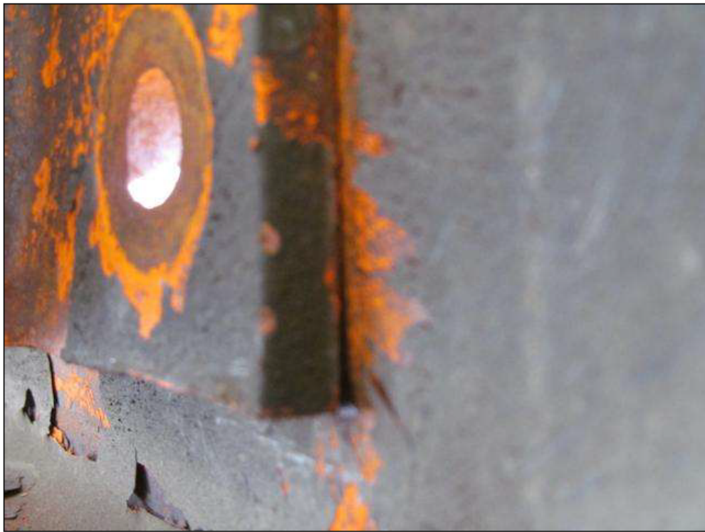
BOTTOM OF DIAPHRAGM PLATE HAS PULLED AWAY FROM THE WEB ( 1/16" +/- ) @ 21'-4" FROM THE FACE OF BENT 2. BEAM 1, SPAN 2
