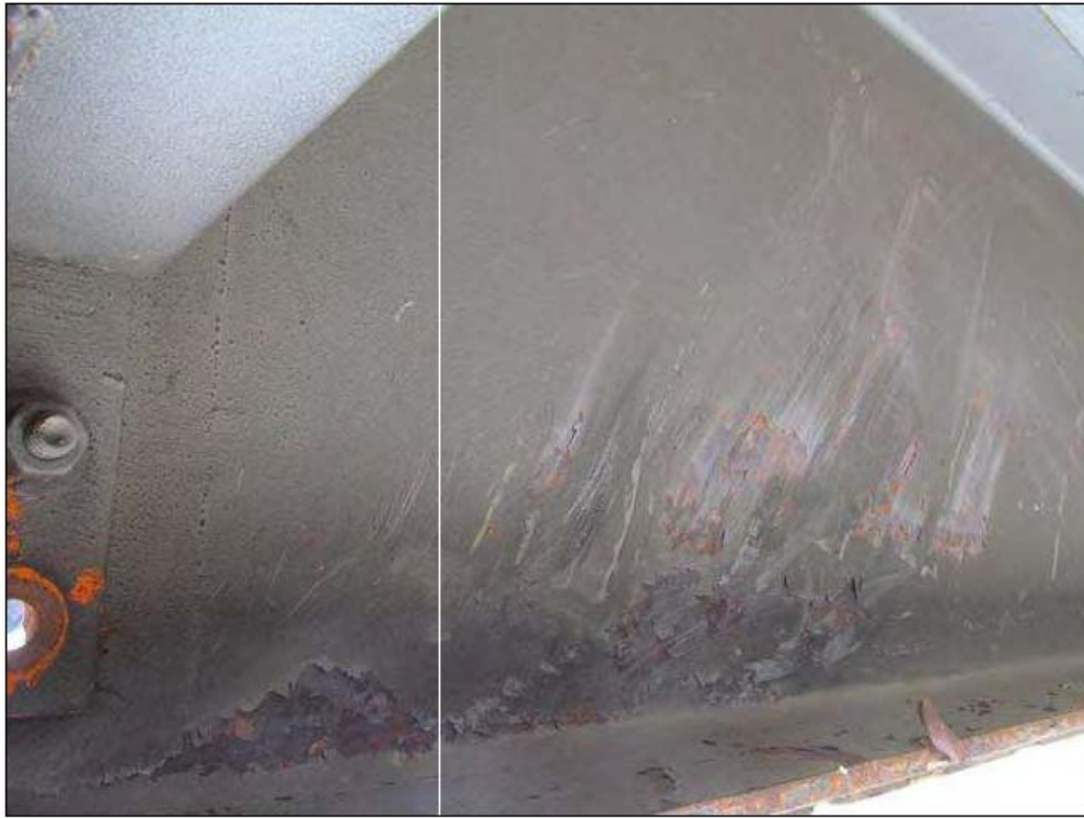
SCRAPES ON INSIDE OF WEB ON BEAM 1, SPAN 2 ABOVE NBL
