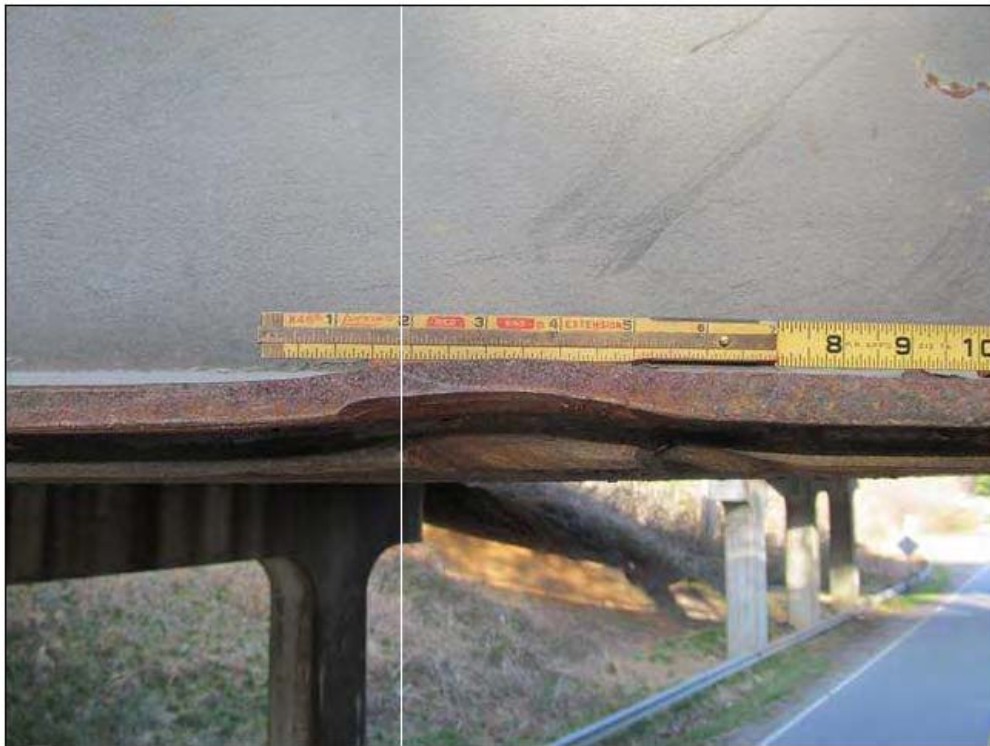
POINT OF IMPACT ON BEAM 1 IS 28'-3" FROM THE FACE OF BENT 1. INDENTION IN FLANGE ( 5" X 1/8" ) & COVER PLATE ( 5" X 1/4" ). BEAM 1, SPAN 2
