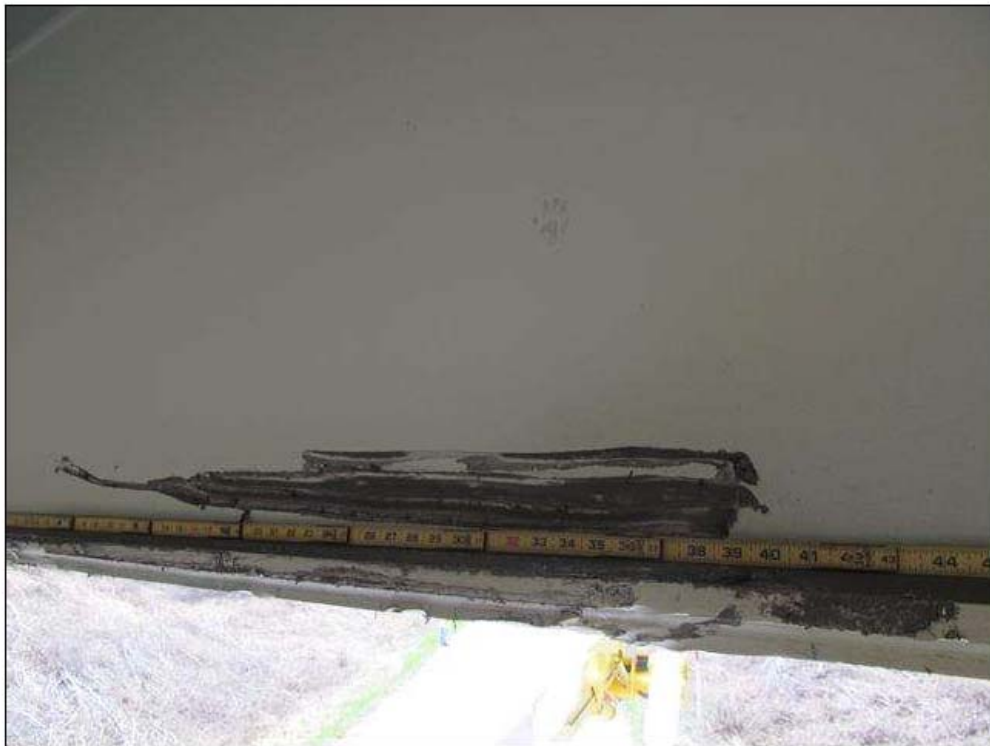
SCRAPES ON BEAM 5 FROM 17'-8" FROM BENT 1 TO 24'-9" FROM FACE OF BENT 2
