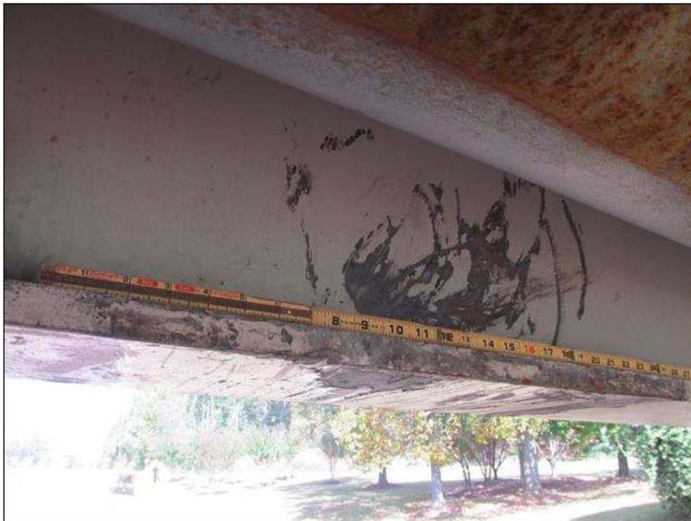
IMPACT ZONE 2, @ 13.083' OUT FROM BENT 2 BEARING, AREA IS 2' LONG
