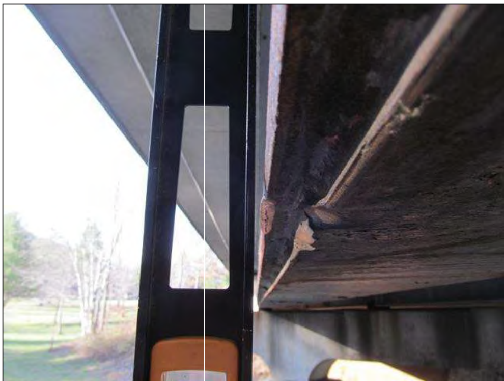
BEAM 1 IS OUT OF PLUMB ( 1/2" ) TO THE SOUTH @ 26'-3" FROM THE FACE OF BENT 1. BEAM 1, SPAN 2
