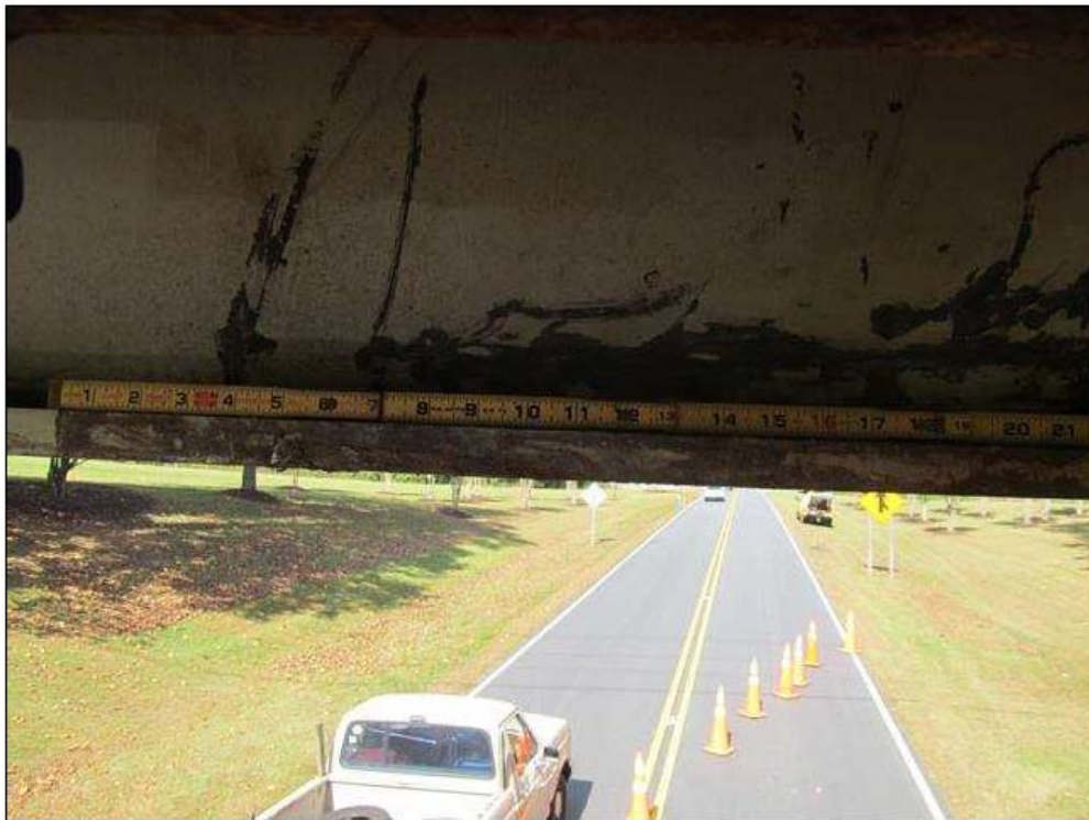
IMPACT AREA @ 20.167' OUT FROM BEARING AT BENT 2, AREA IS 2' LONG
