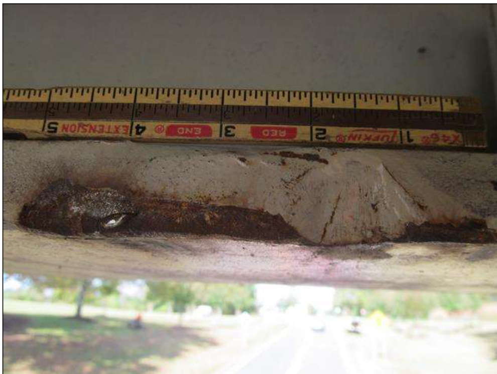
OLD IMPACT AREA @ 16.417' OUT FROM BENT 2 BEARING, DIVOT IS 1"WIDE X 1/2"DEEP IN BOTTOM FLANGE.
