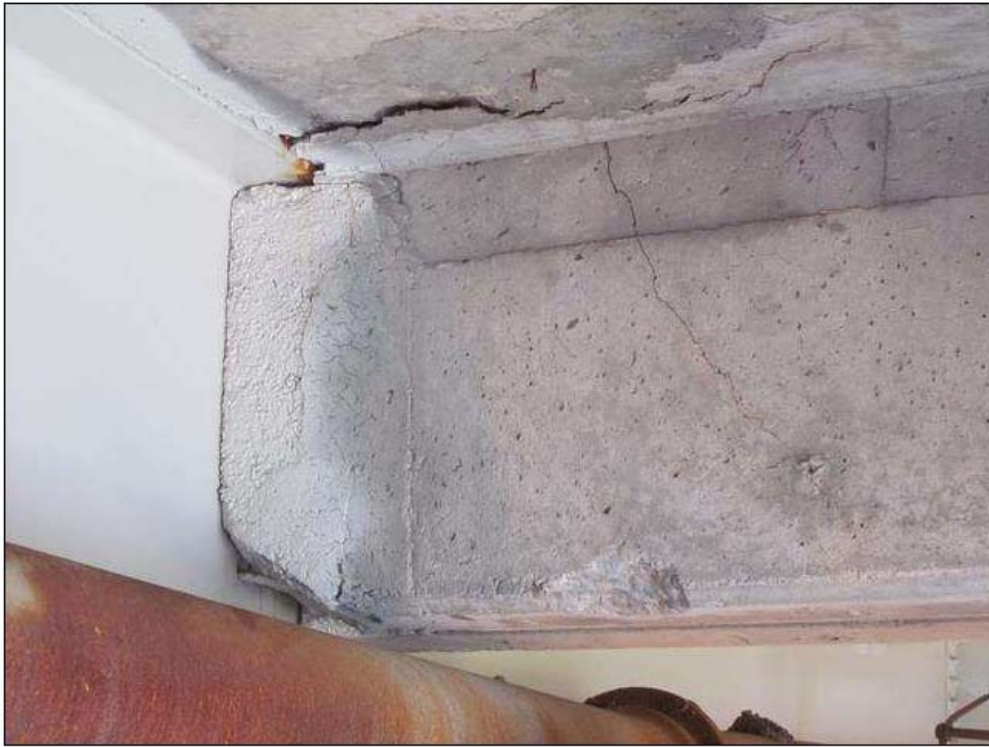
END DIAPHRAGM IN BAY 1, AT BENT 2. CRACKED.
