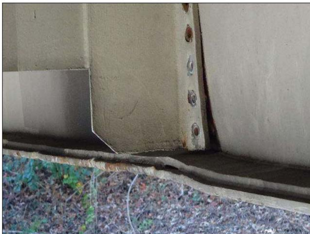
SPAN 3 BEAM 1 AT 20FT FROM BENT 3, BROKEN WELD BETWEEN COVER PLATE AND BOTTOM FLANGE (UP TO 4IN)
