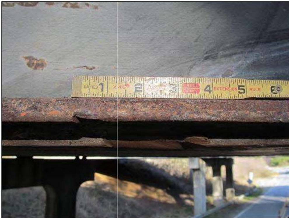
INDENTATION IN COVER PLATE ( 3" X 1/4" ) AND FLANGE ( 1" X 1/4" ) @ 24'-2" FROM THE FACE OF BENT 1. BEAM 1, SPAN 2
