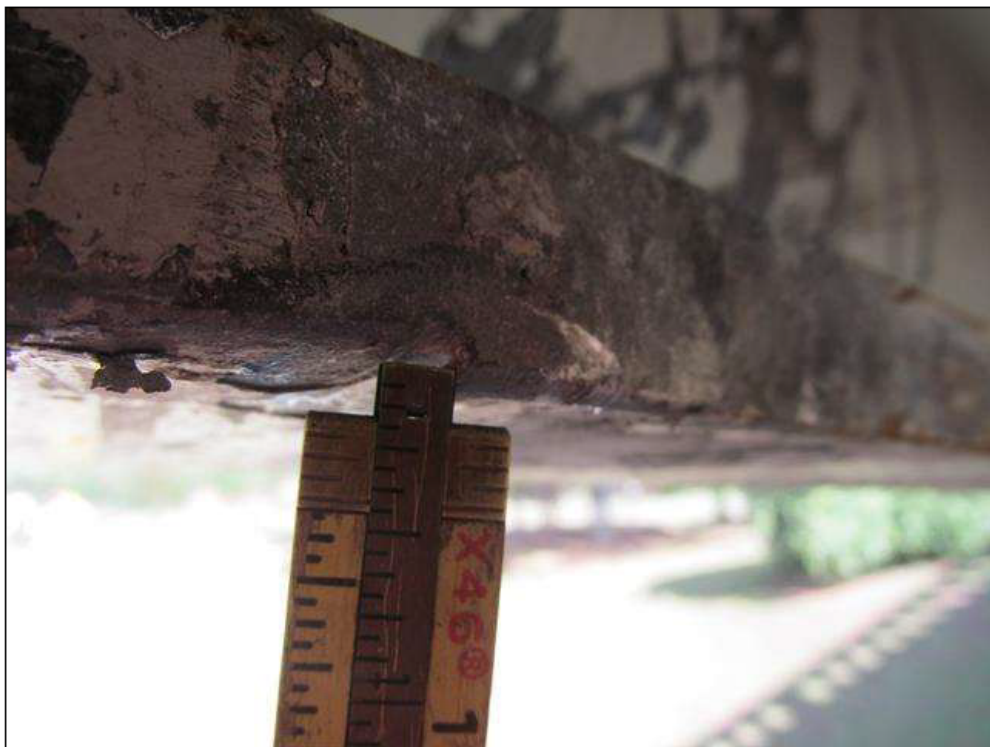
VIEW OF 1/8" DEEP OF SCRAPE TO BOTTOM FLANGE ON BEAM 1
