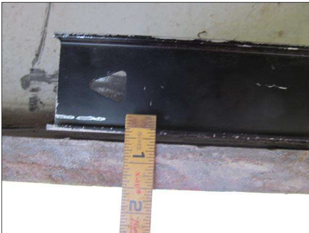
BEAM 1, BOTTOM FLANGE BENT DOWNWARD, UP TO A 1/4"
