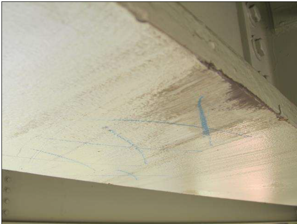
BEAM 2, @ 19.75 FROM BENT 2 BEARING, SCRAPE MARKS
