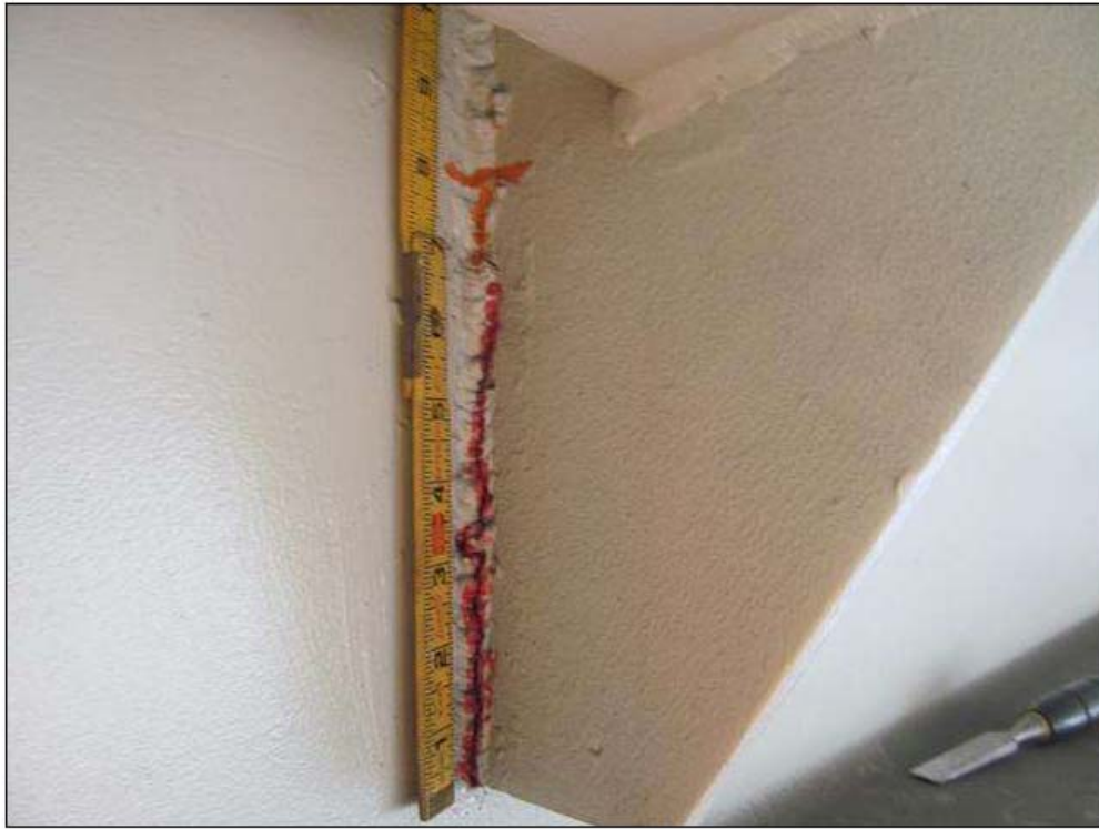
A 8" LONG CRACK IN DIAPHRAGM WELD AT DIAPHRAGM ON BEAM 5 AT 20'-00" FROM FACE OF BENT 2
