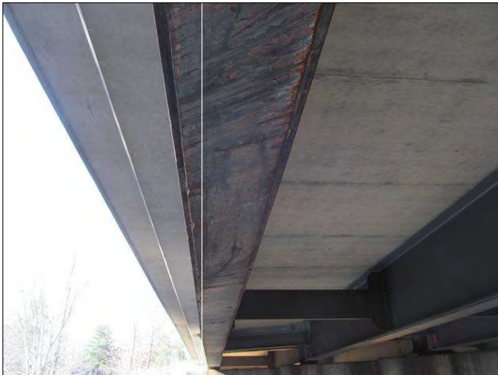
SCRAPES ON THE BOTTOM OF BEAM 1 IN FLANGE & COVER PLATE. FROM 12'-4" OF BENT 1 TO 8'-10" OF BENT 2. BEAM 1, SPAN 2
