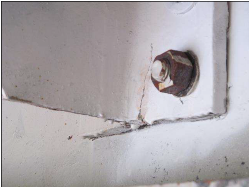
CRACK ON DIAPHRAGM CONNECTION BRACKET HAS NOT CHANGED FROM PREVIOUS HIT.
