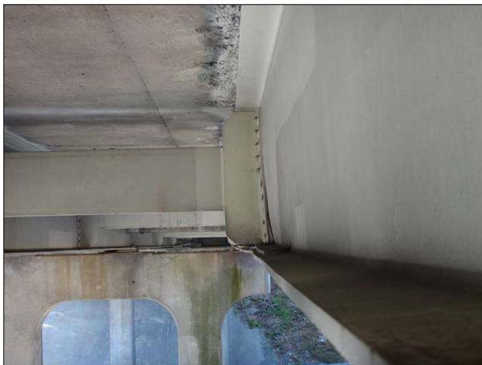
SPAN 3 BEAM 1 AT 20FT FROM BENT 3, TWO ROWS OF FIVE BOLTS SHEARED AND MISSING FROM IMPACT DAMAGE
