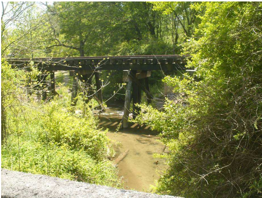
Photograph No. 4: View looking south downstream from bridge deck
