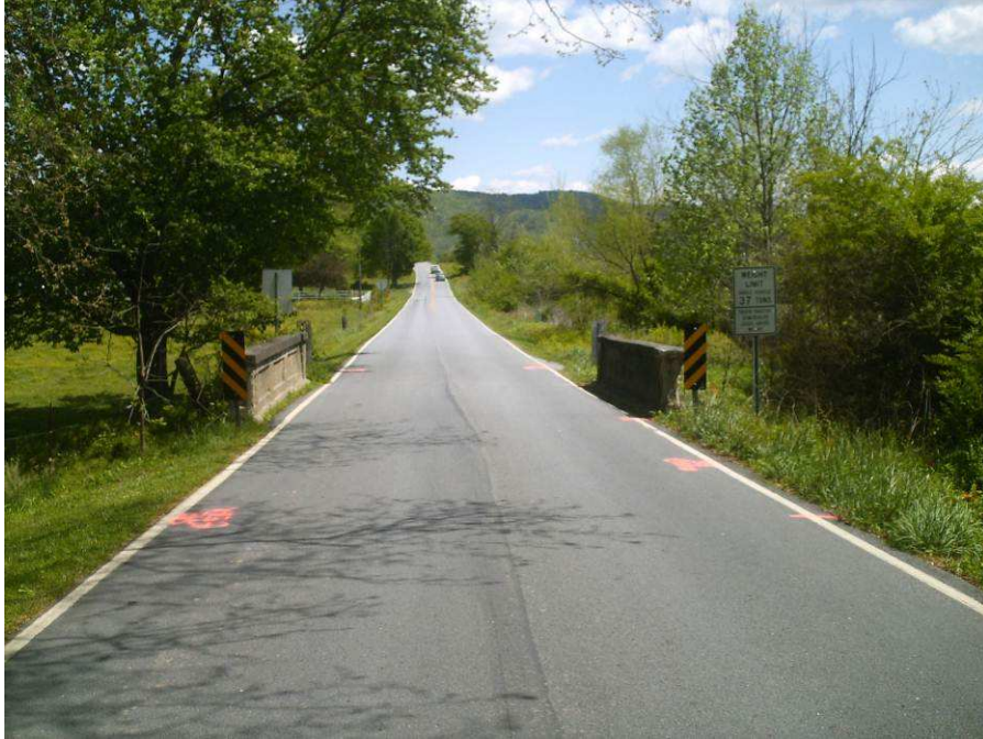
Photograph No. 1: View looking east up-station from west approach
