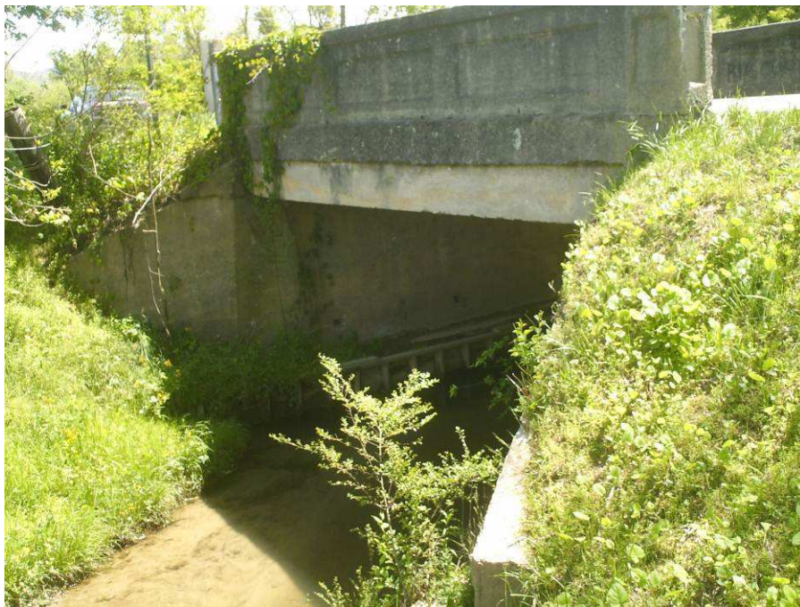
Photograph No. 6: View looking east at End Bent 2
