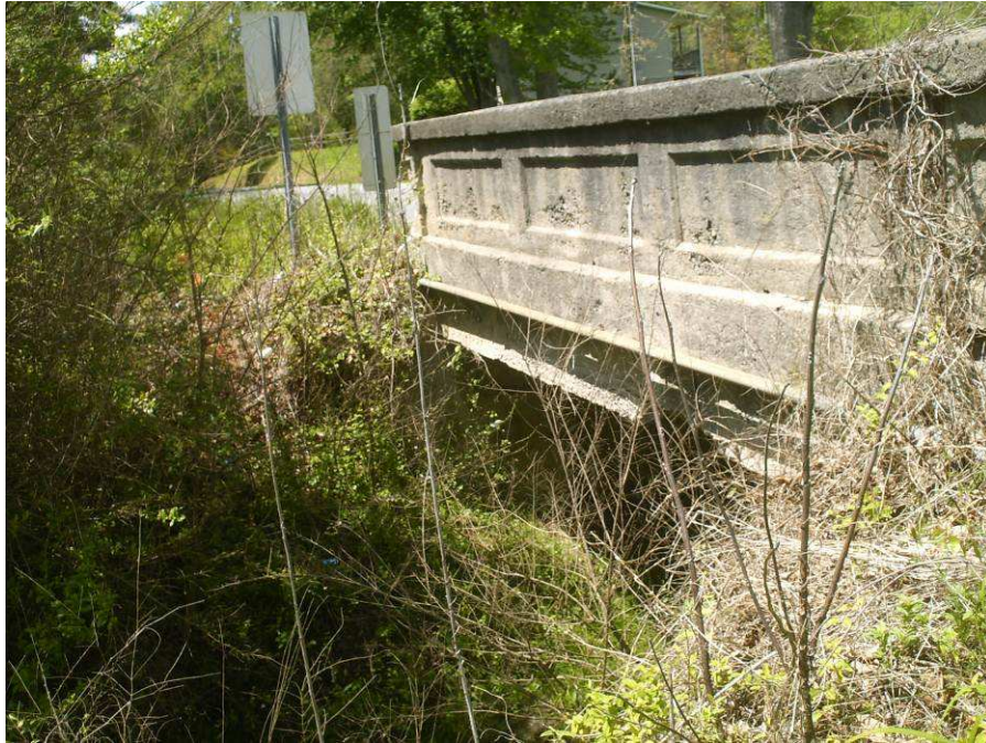
Photograph No. 5: View looking west at End Bent 1
