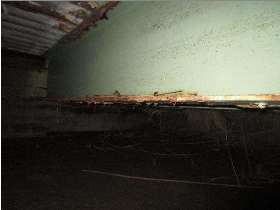
Span 5 Beam 10: SPAN 6, INTERMITTENT FULL LENGTH AREA OF SECTION LOSS DOWN TO 5/16IN REMAINING IN BOTTOM FLANGE, PAR
