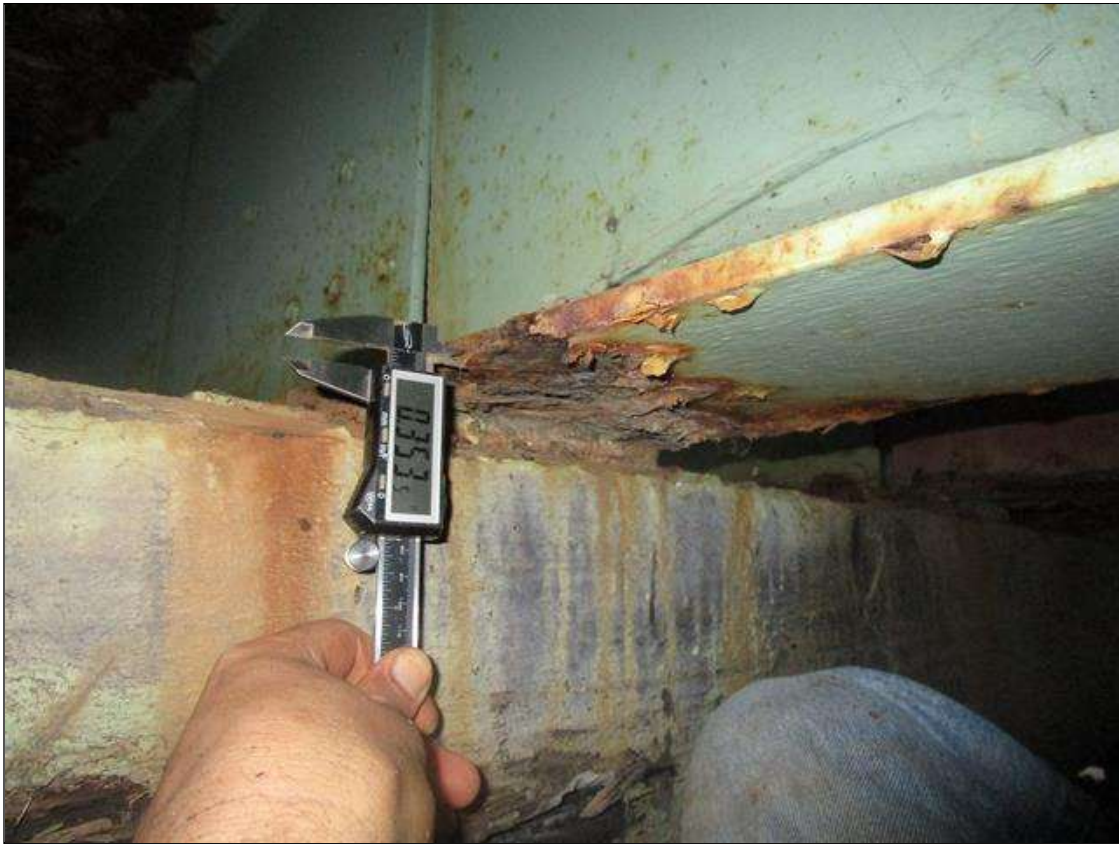
Span 1 Beam 3: SPAN 2, AT BENT 2, 1FT AREA OF SECTION LOSS WITH 0.353IN REMAINING IN BOTTOM FLANGE, PAR
