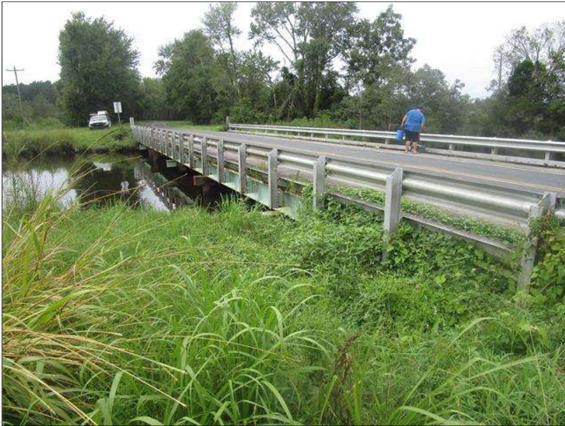
UPSTREAM STRUCTURE PROFILE, LOOKING NORTH
