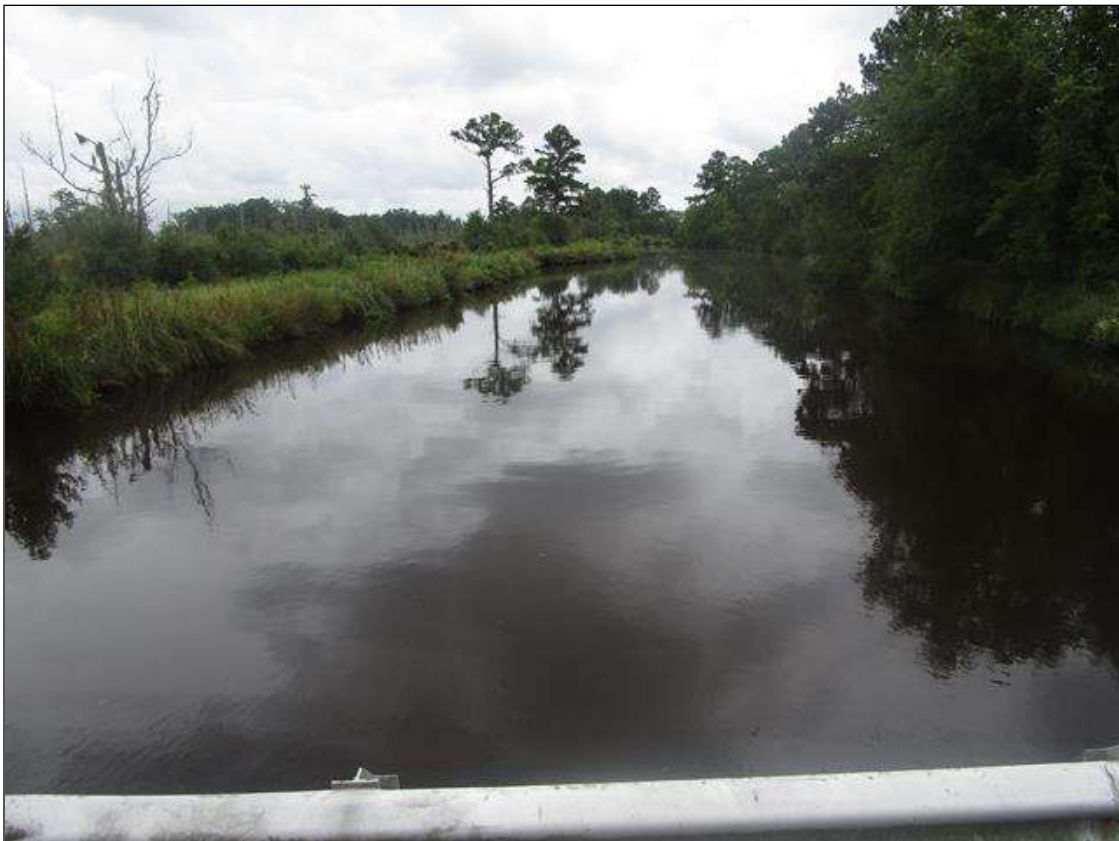
LOOKING UPSTREAM, SOUTH
