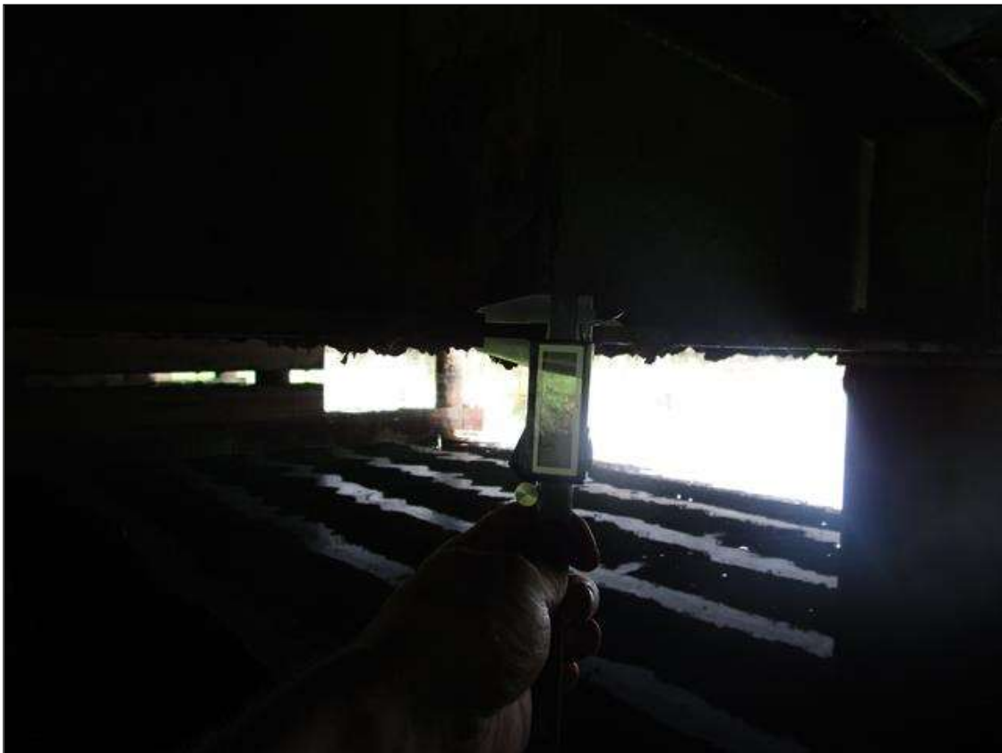
Bent 1 Cap 1: AT BEAM 6, 0.285IN REMAINING IN BOTTOM FLANGE, PAR
