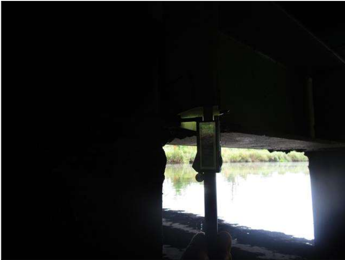
Bent 1 Cap 1: AT BEAM 8 AND PILE 4, 0.20IN REMAINING WITH 1.5IN BENDING DISTORTION OF FLANGE, PAR
