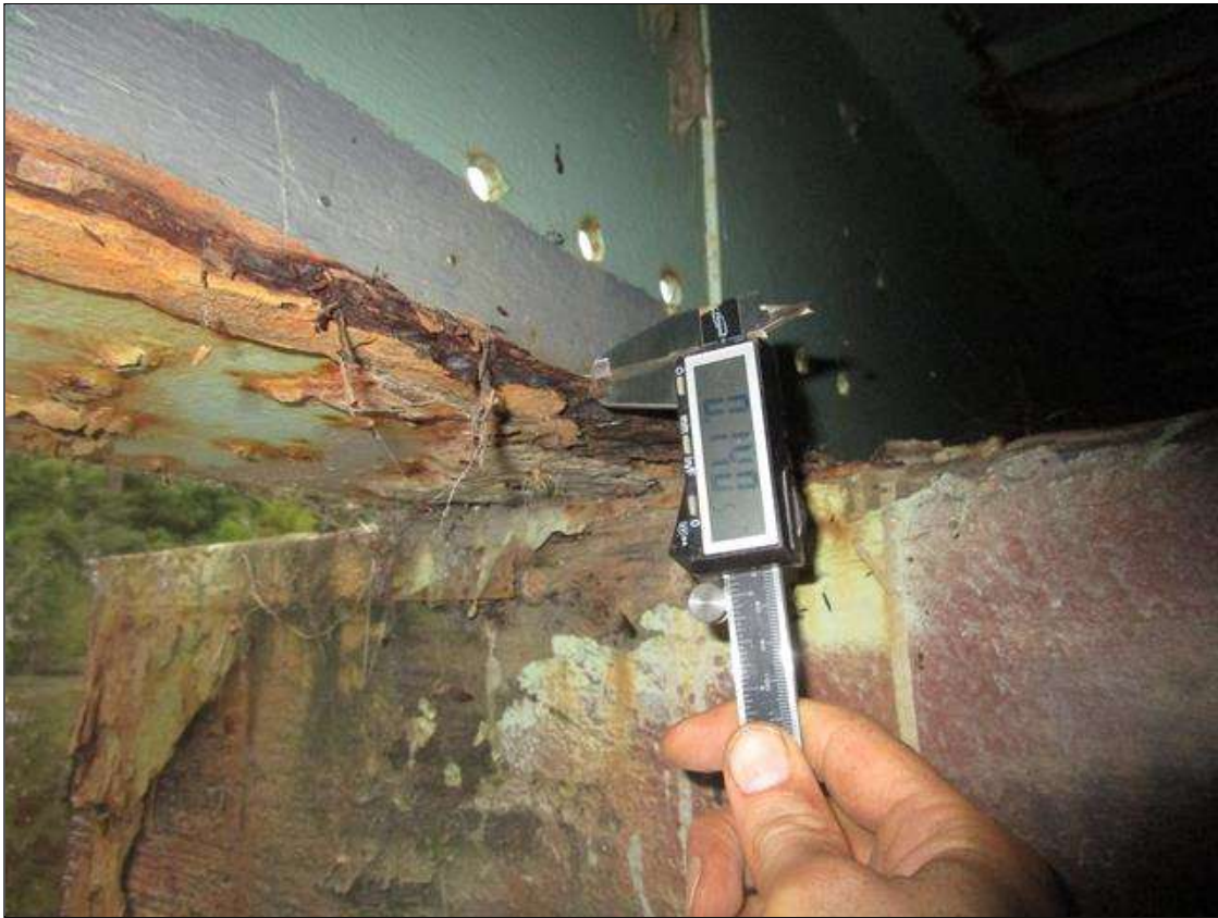
Span 1 Beam 1: SPAN 2, AT BENT 2, 2FT AREA OF SECTION LOSS DOWN TO 0.14IN REMAINING IN BOTTOM FLANGE, PAR
