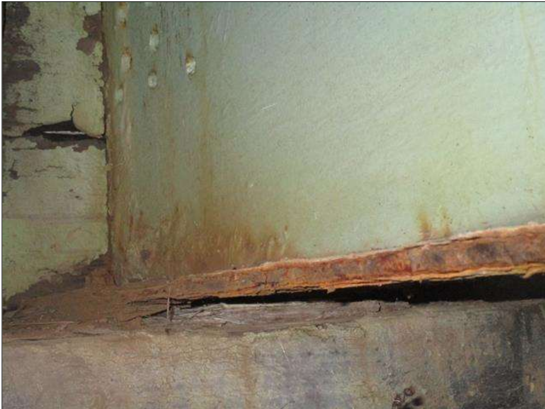
Span 5 Beam 4: SPAN 6, AT END BENT 2, 2FT AREA OF SECTION LOSS DOWN TO 3/16IN REMAINING IN BOTTOM FLANGE, PAR
