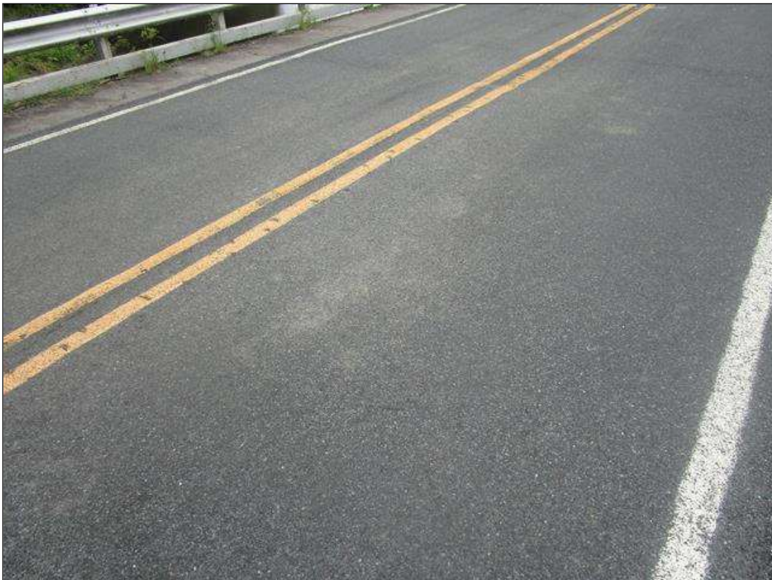
SPAN 1 WEARING SURFACE
