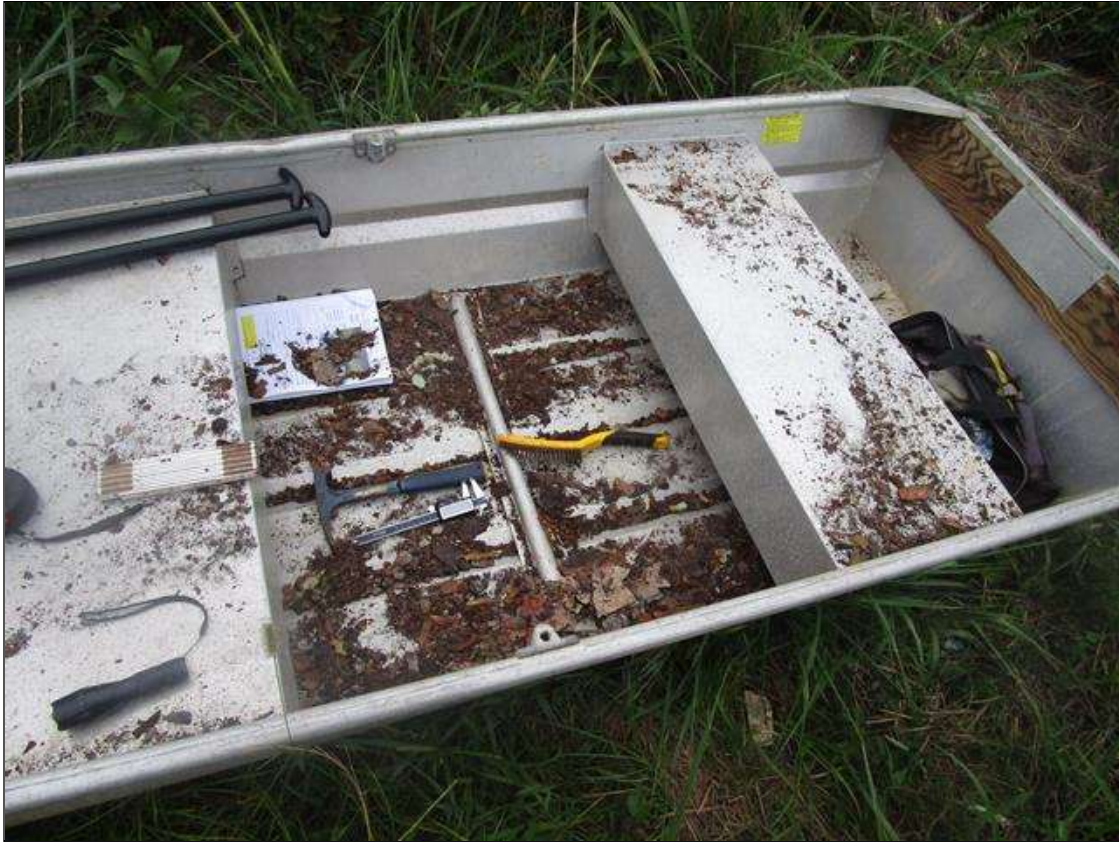
INSPECTION BOAT WITH CORRODED STEEL REMOVED FROM BEAMS
