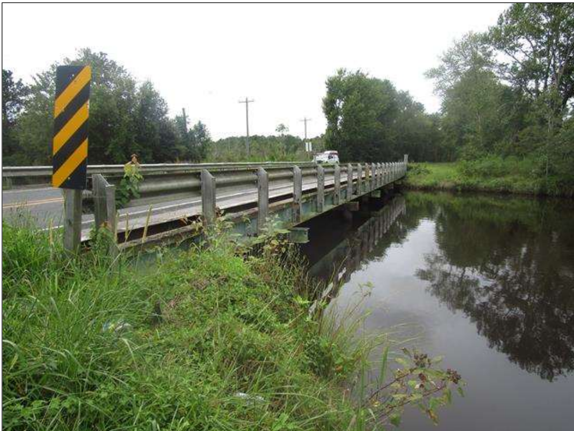
DOWNSTREAM STRUCTURE PROFILE, LOOKING SOUTH
