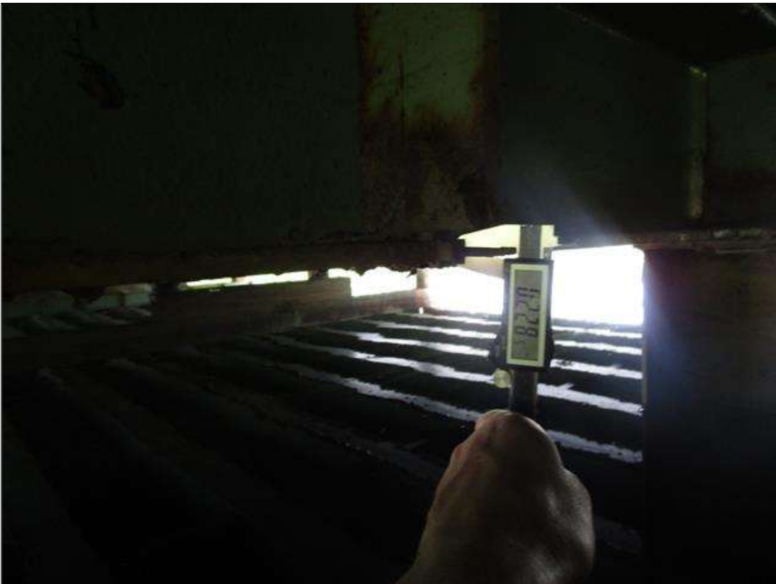
Bent 1 Cap 1: 1FT OF CORROSION IN BOTTOM FLANGE AT BEAM 4, 1IN WIDE X 1FT LONG AREA OF SECTION LOSS DOWN TO 0.228IN REMAINING IN BOTTOM FLANGE, PAR
