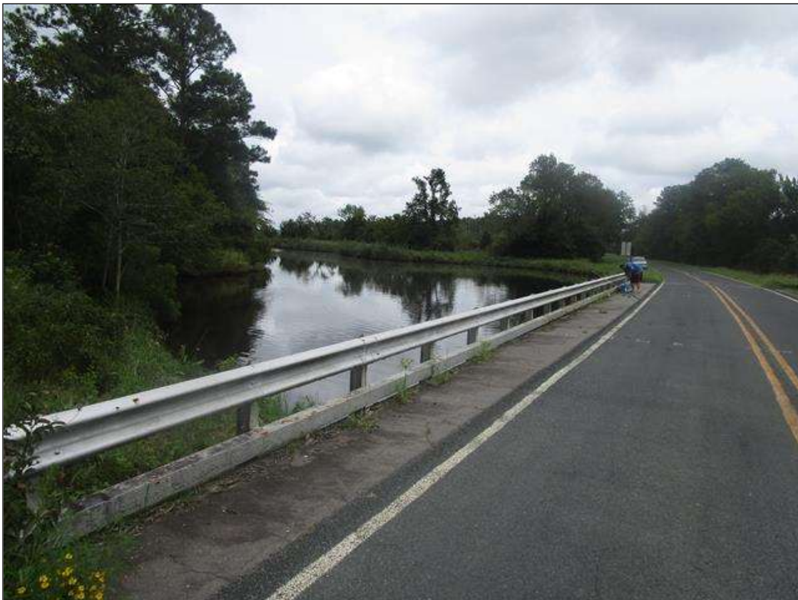
LEFT BRIDGE RAIL
