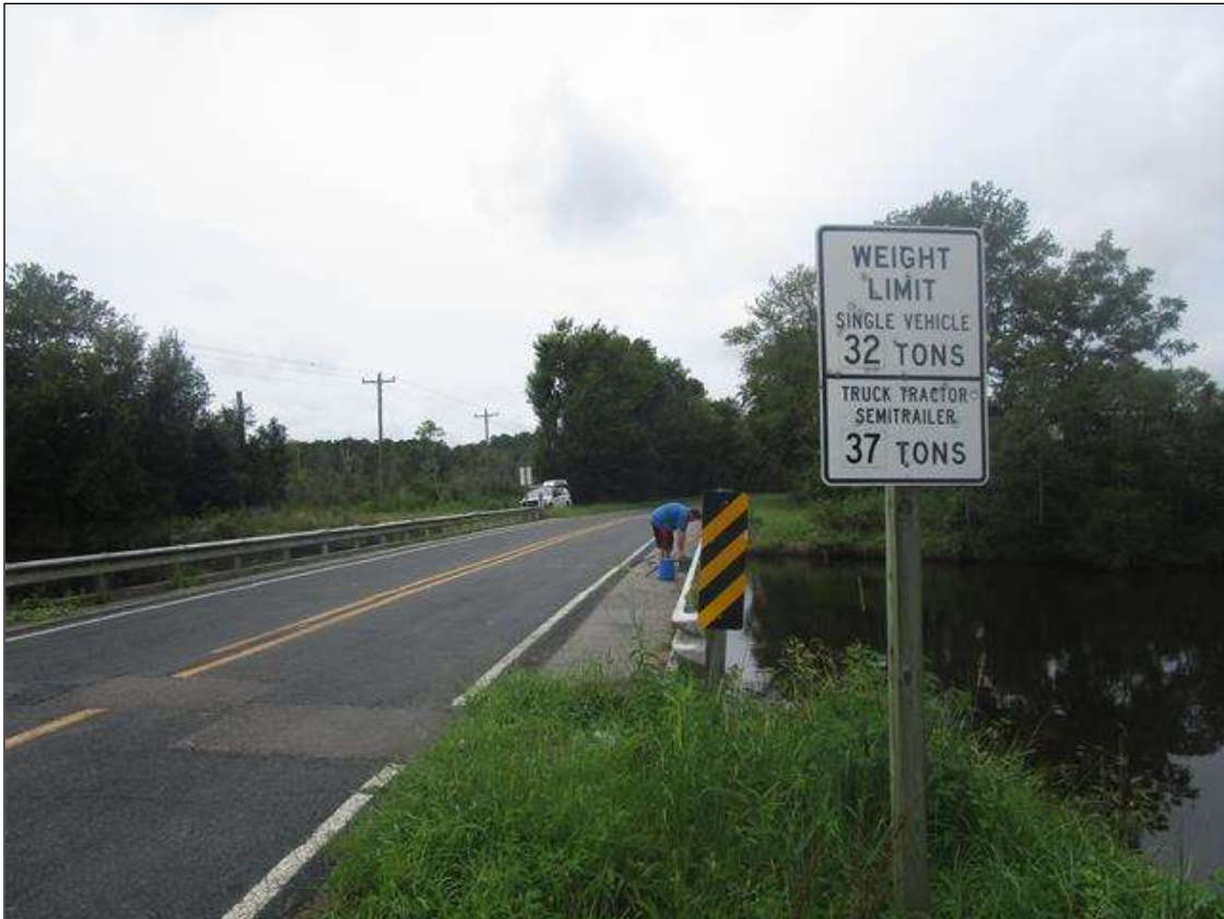
EAST APPROACH WEIGHT LIMIT SIGN
