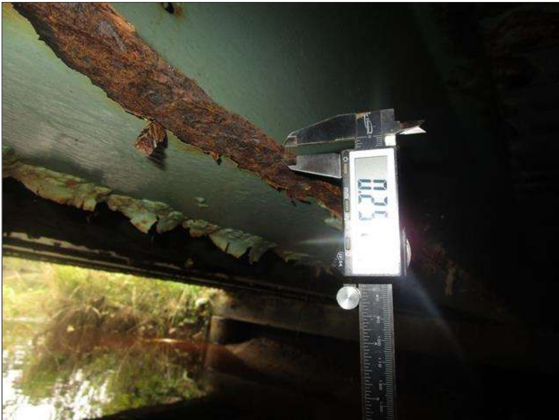
Span 5 Beam 5: SPAN 6, BEAM 5 AT MID SPAN, SECTION DOWN TO 0.25IN REMAINING IN BOTTOM FLANGE, PAR
