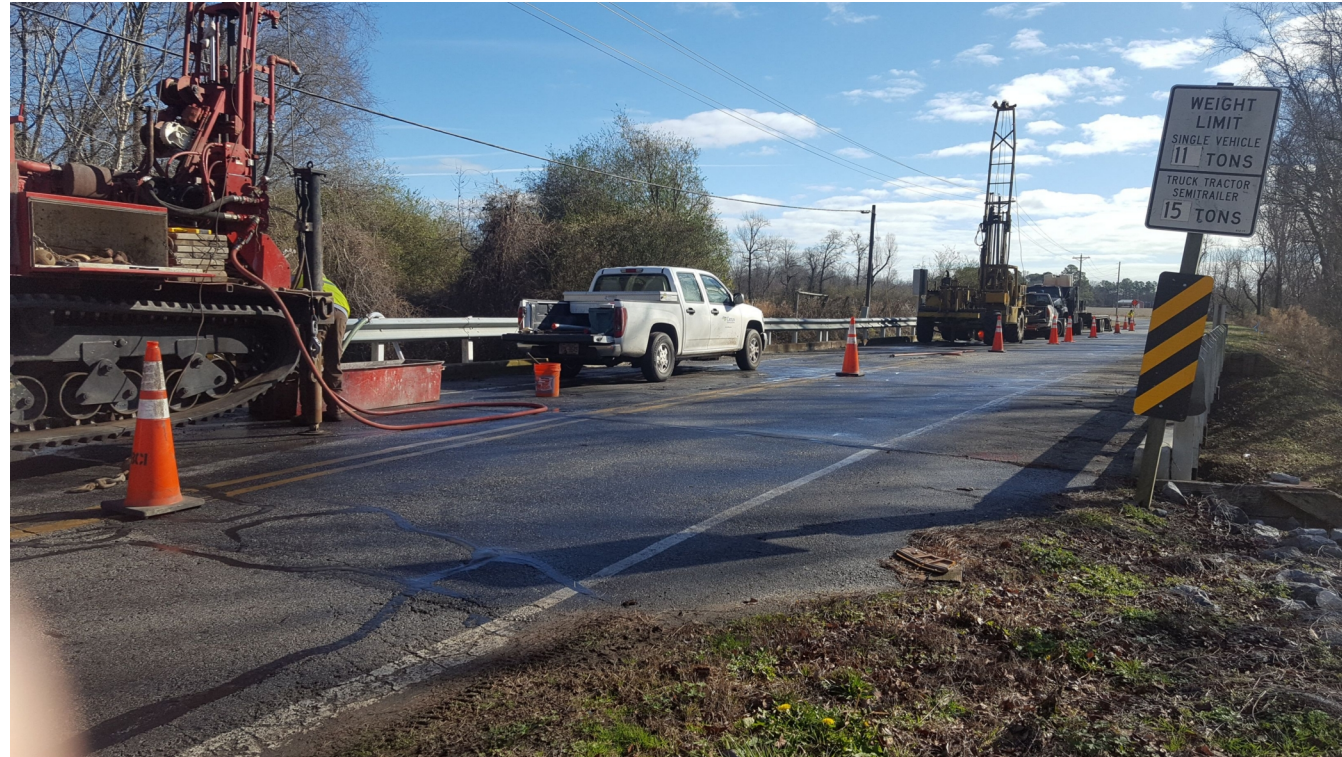
EB1 FOREGROUND - FACING EAST
