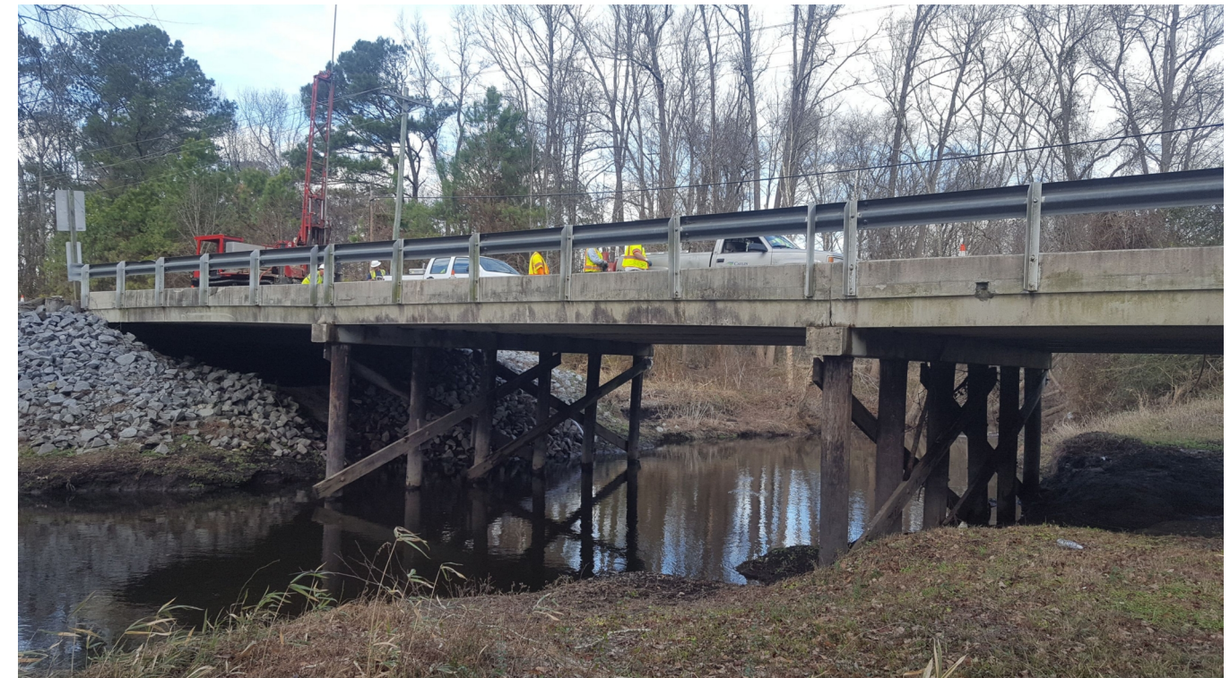
AT EB2 FACING DOWNSTREAM
