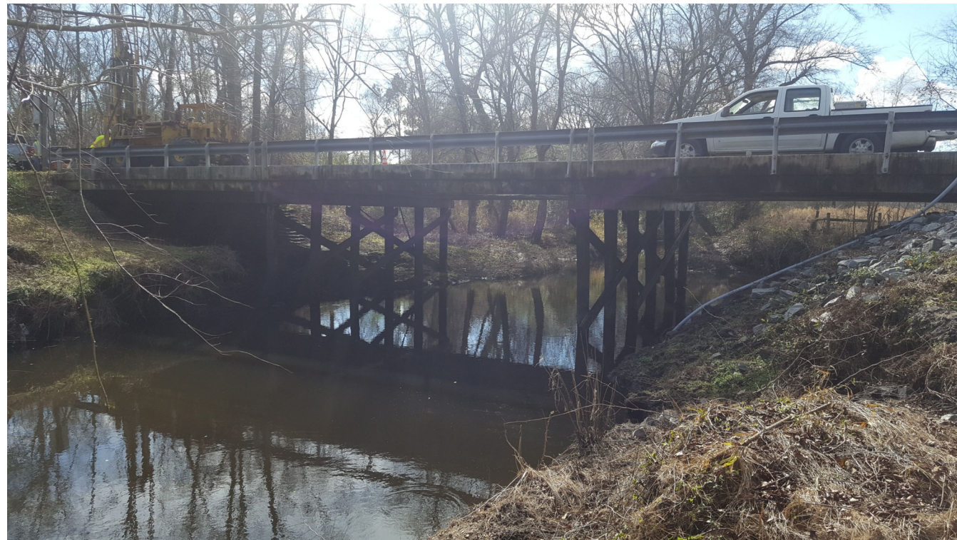
AT EB1 FACING UPSTREAM
