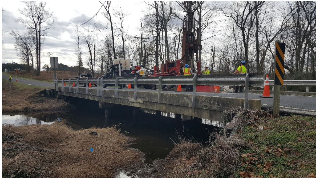
EB2 FOREGROUND FACING DOWNSTREAM
