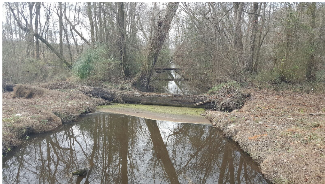
DOWNSTREAM FROM BRIDGE
