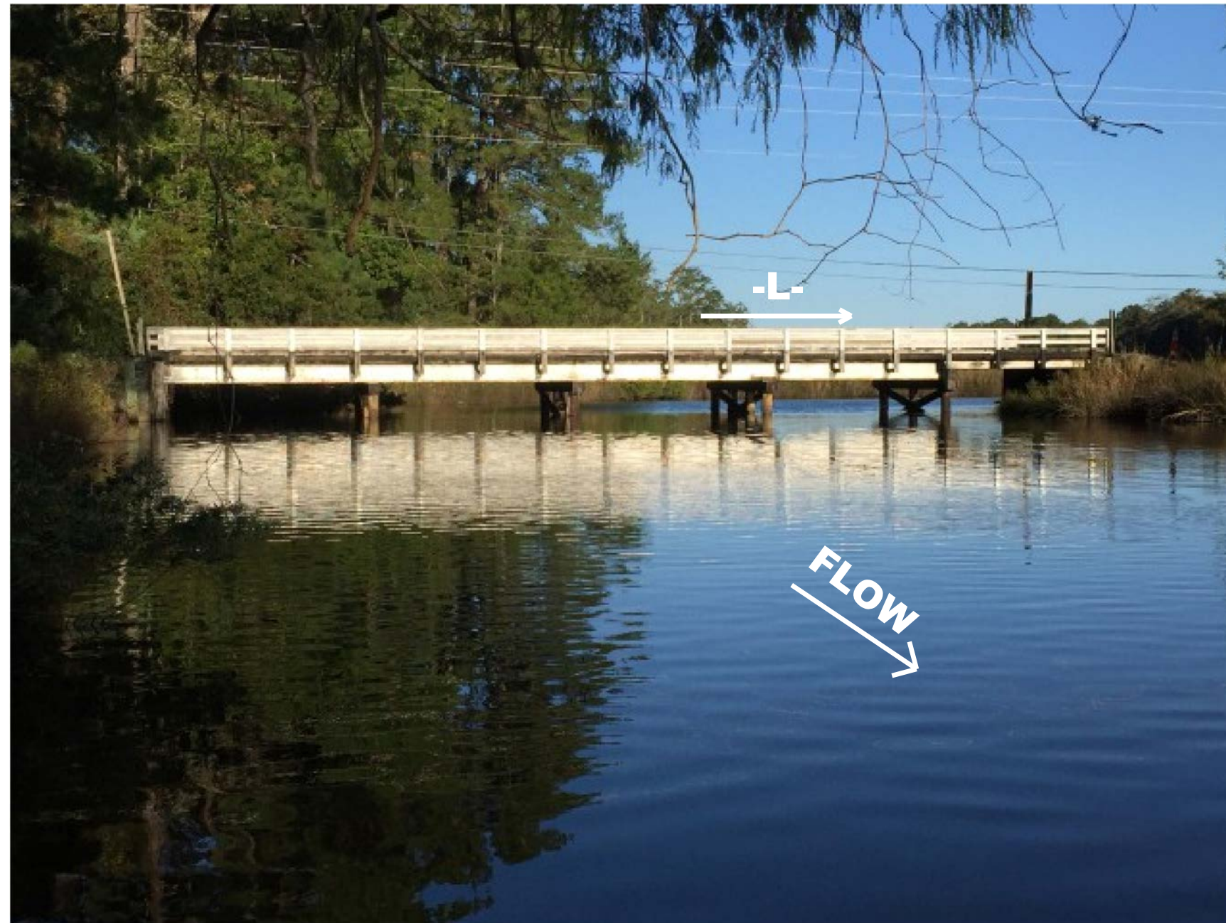
PHOTOGRAPH NO.1. VIEW LOOKING NORTHWEST
