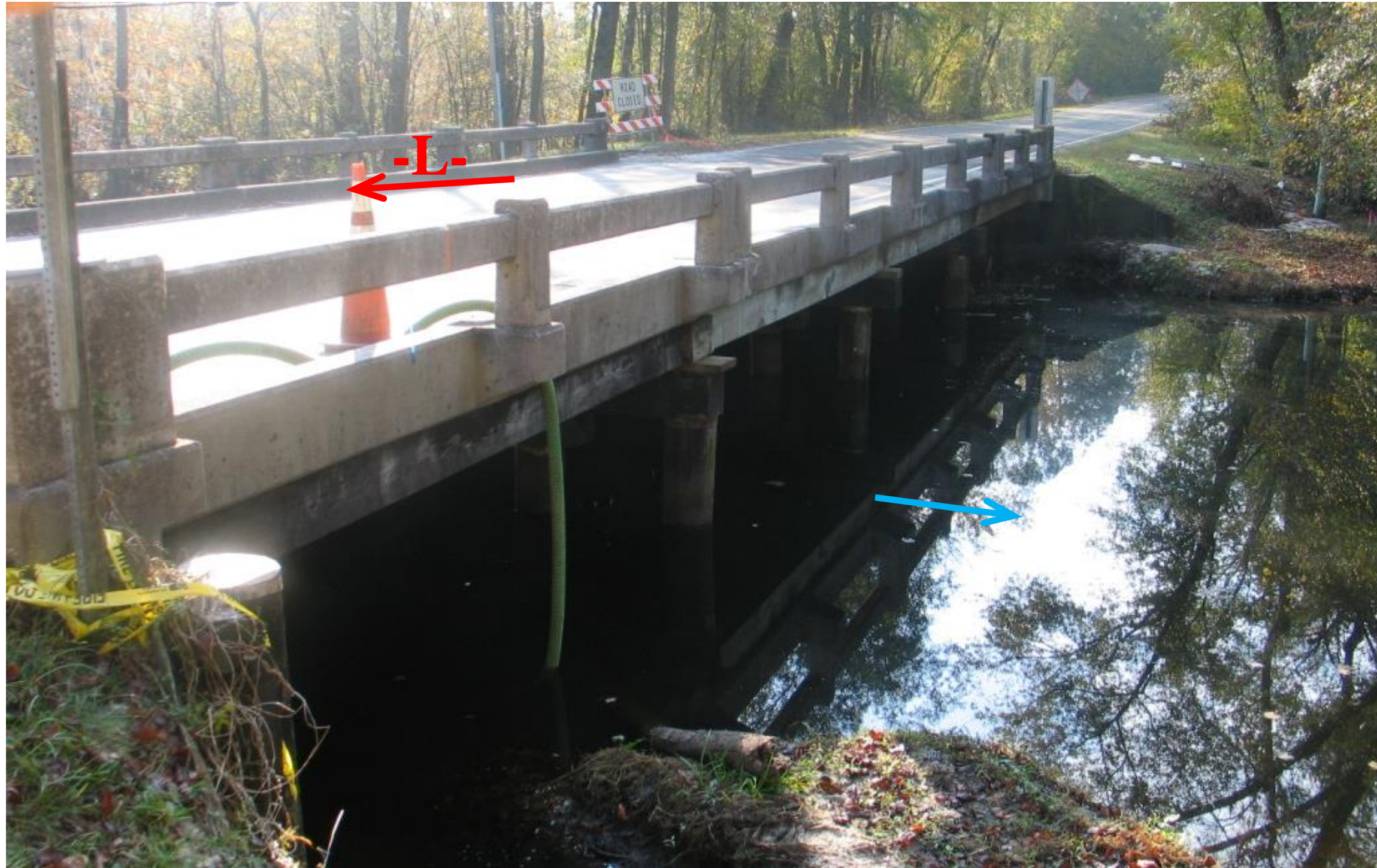
Looking Southeast towards End Bent 1
