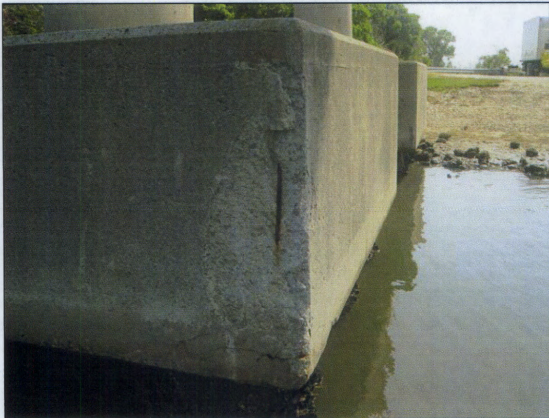
BENT 5 NORTHWEST CORNER SPALL ON FOOTING
