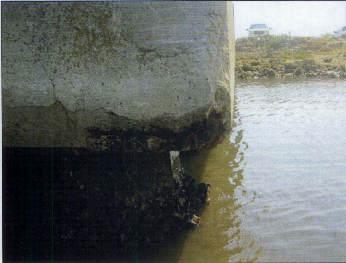
BENT 4 NORTHWEST CORNER SPALL ON FOOTING
