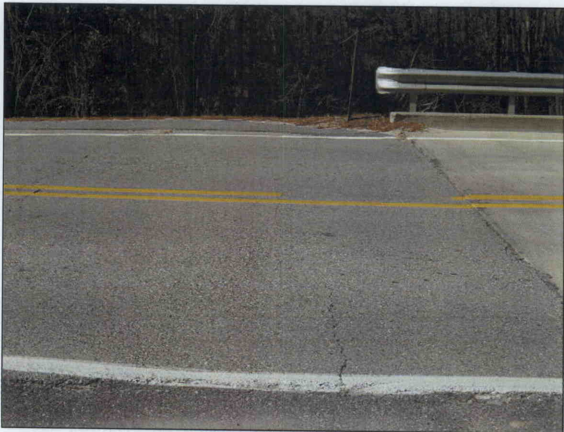
SOUTH APPROACH ASPHALT WEARING SURFACE CRACKED AND SETTLED 1"
