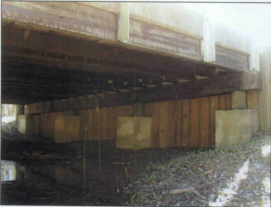
END BENT 1 ALL PILES ENCASED IN CONCRETE
