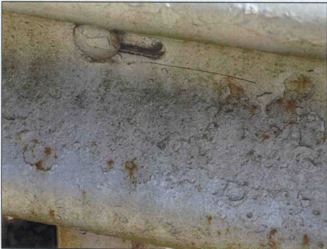
SURFACE RUST ALONG RAILS
