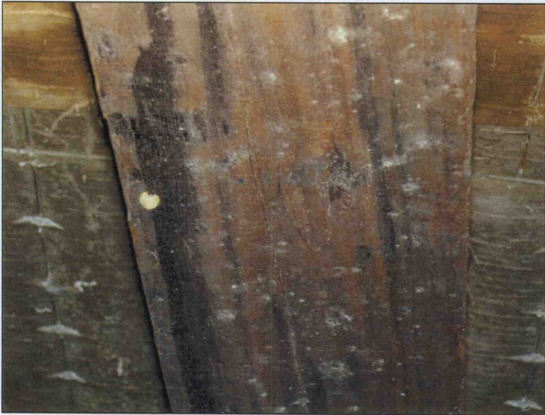
LONGITUDINAL CRACKING ALONG JOIST UP TO 1/16" WIDE
