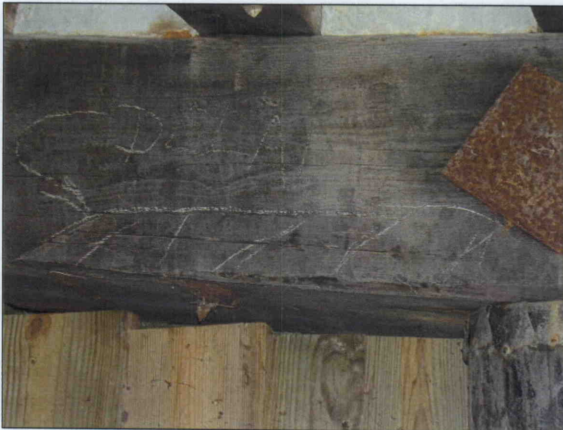
END BENT 2 CAP AT PILE 3 DELAMINATED AREA 30" LONG X 4" HIGH.
