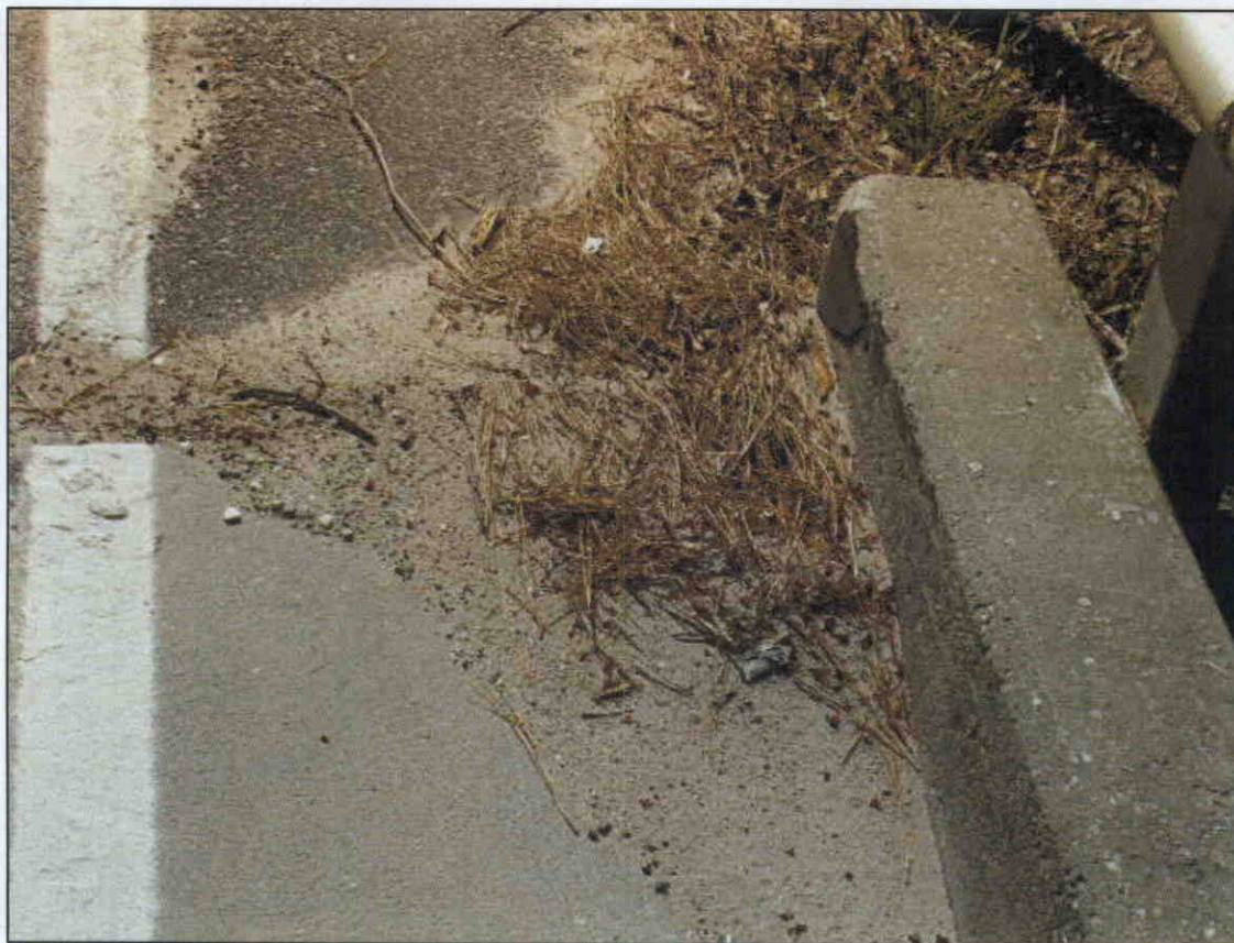
DEBRIS BUILDUP AT SOUTHWEST CORNER CURB, SIMILAR AT NORTHWEST CORNER
