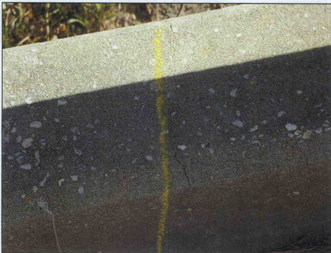
HAIRLINE CRACKING ALONG CURBS
