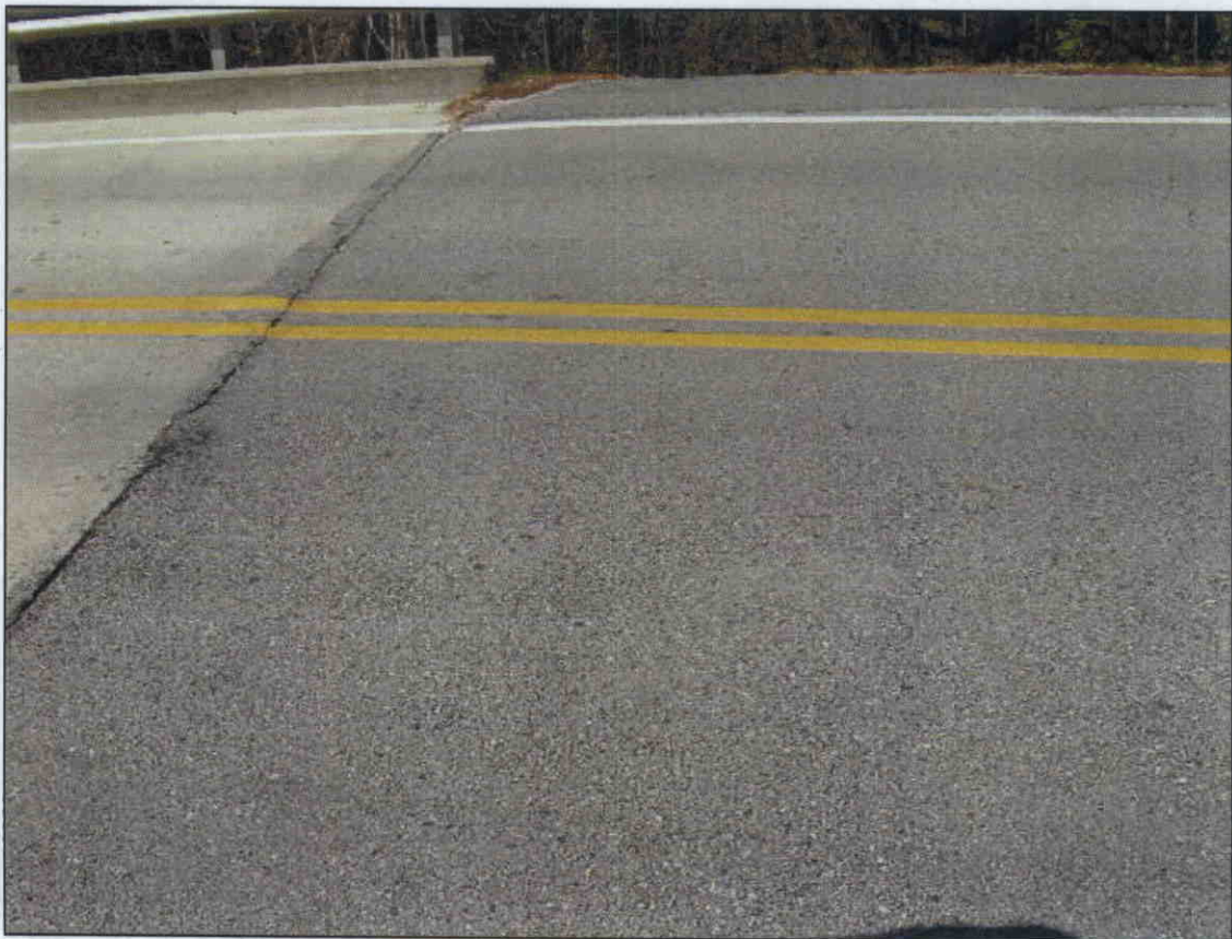
NORTH APPROACH ASPHALT WEARING SURFACE CRACKED AND SETTLED 1"
