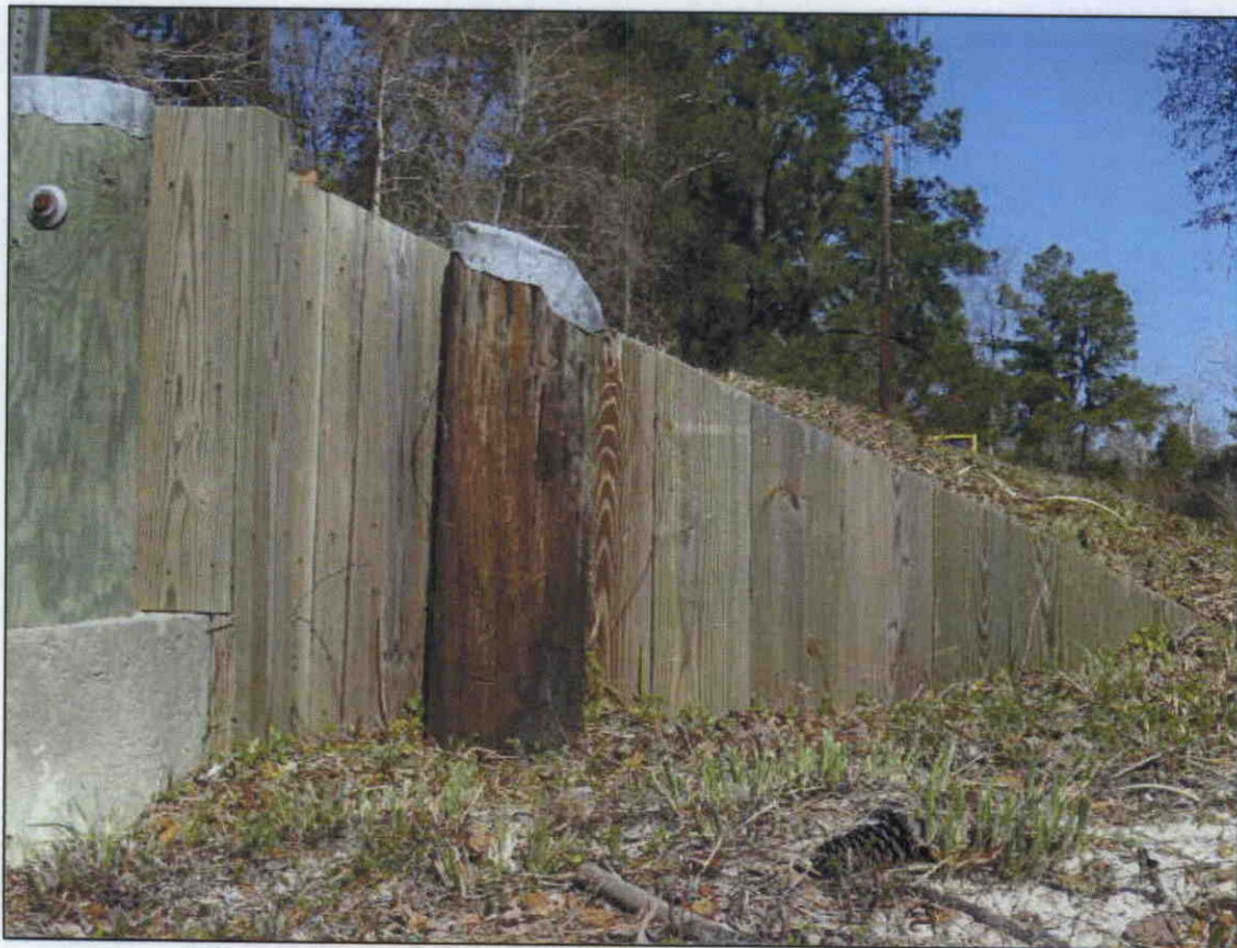
NEW SHEETPILE BOARDS IN PLACE AT ALL WINGWALLS
