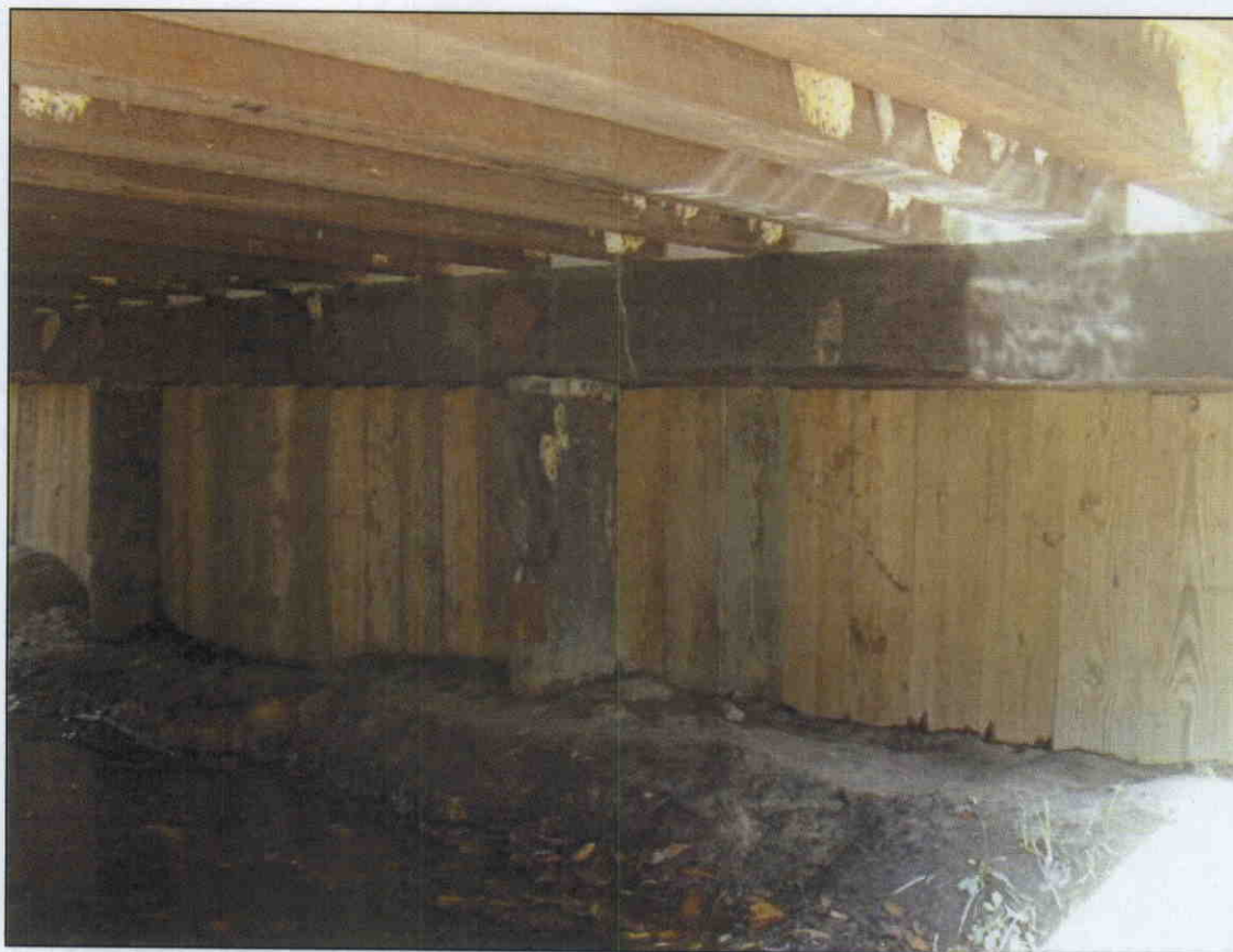
NEW SHEETPILE BOARDS IN PLACE ALONG BOTH BULKHEADS
