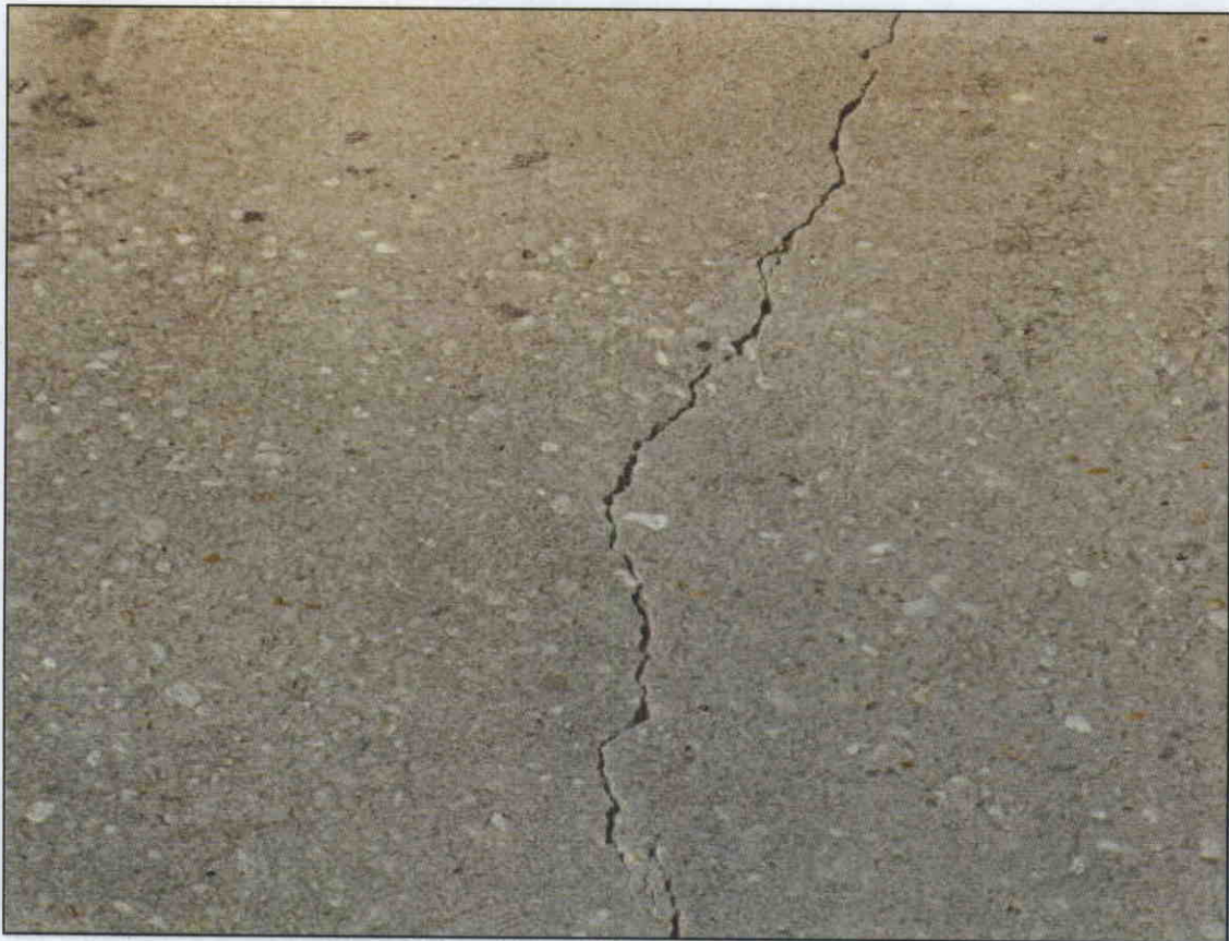
TRANSVERSE CRACKING IN DECK OVER END BENTS
