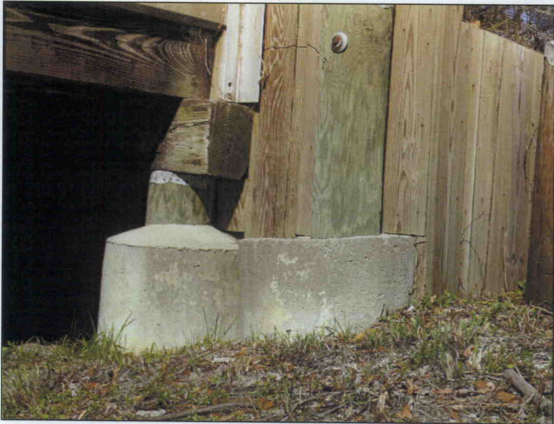
PILE 4 AT END BENT 2 AND NORTHEAST TURNPILE ENCASED IN CONCRETE
