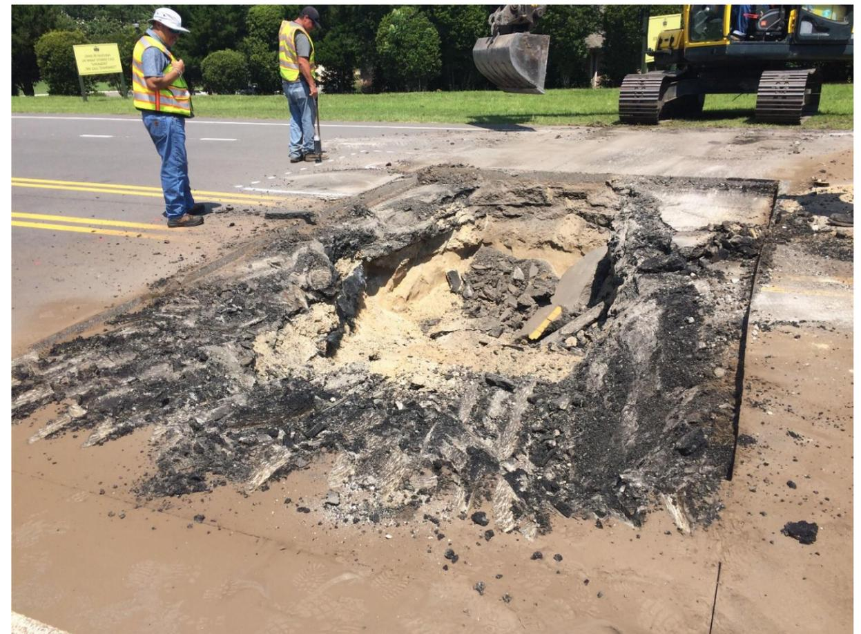
B. Photo looking north showing excavation of sinkhole location by NCDOT personnel. NCDOT person in upper left is marking area to expand excavation based on preliminary GPR results.
