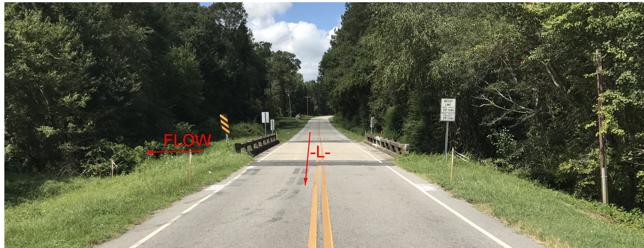
END BENT 2 (-L-) LOOKING WEST
