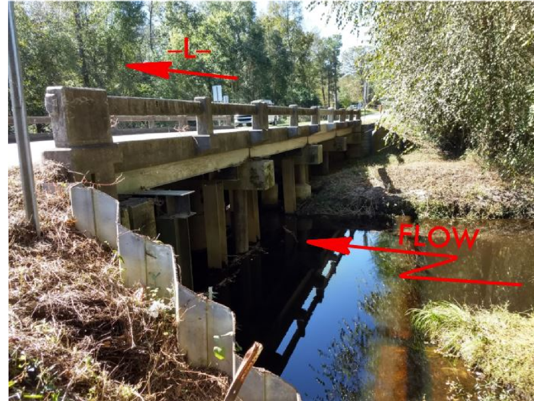
END BENT 2 (-L-) LOOKING SOUTHWEST
