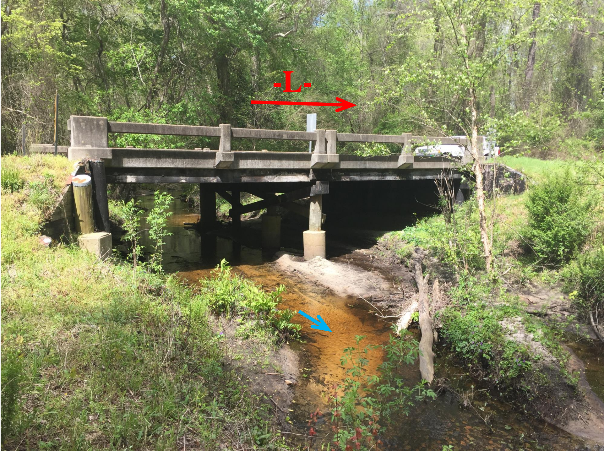
Bridge No. 83 on -L- (SR 1378) over Juniper Creek
