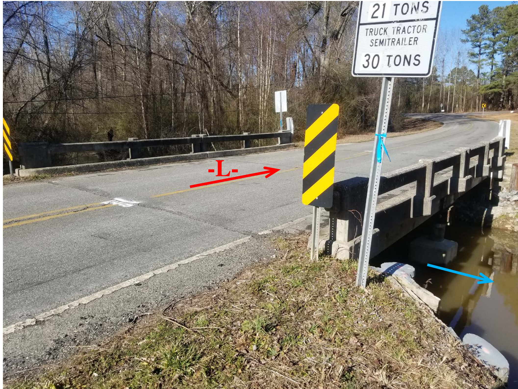
Looking North towards End Bent 2
