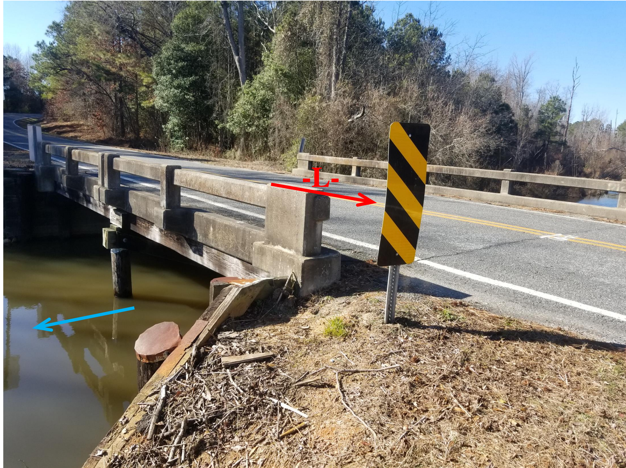
Looking Northwest towards End Bent 1
