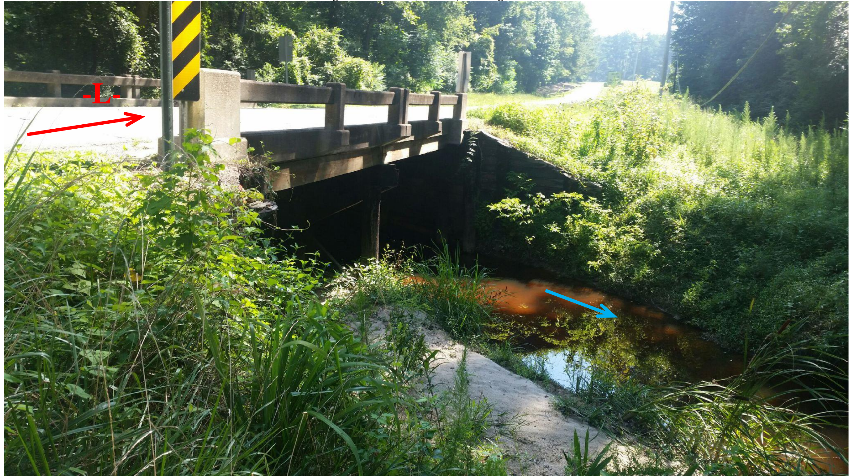
Looking East towards End Bent 2
