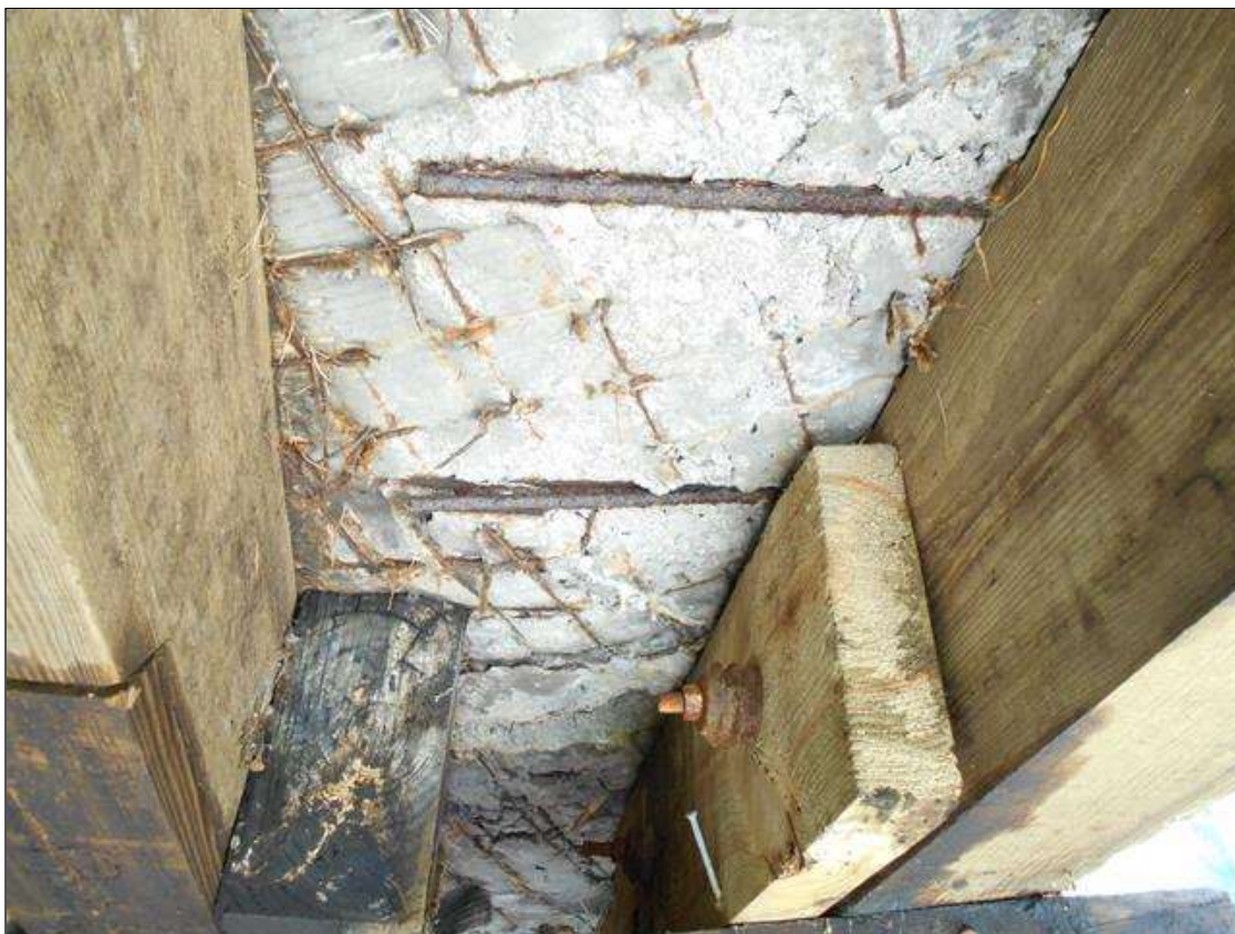
Span 1 Deck: 1 Square Feet of Delamination/Spall: Delaminated. Spall 1 in. or less deep or 6 in. or less in diameter. SPALL IN BOTTOM OF DECK OVER INTERIOR BENT 1 BAY 18.
