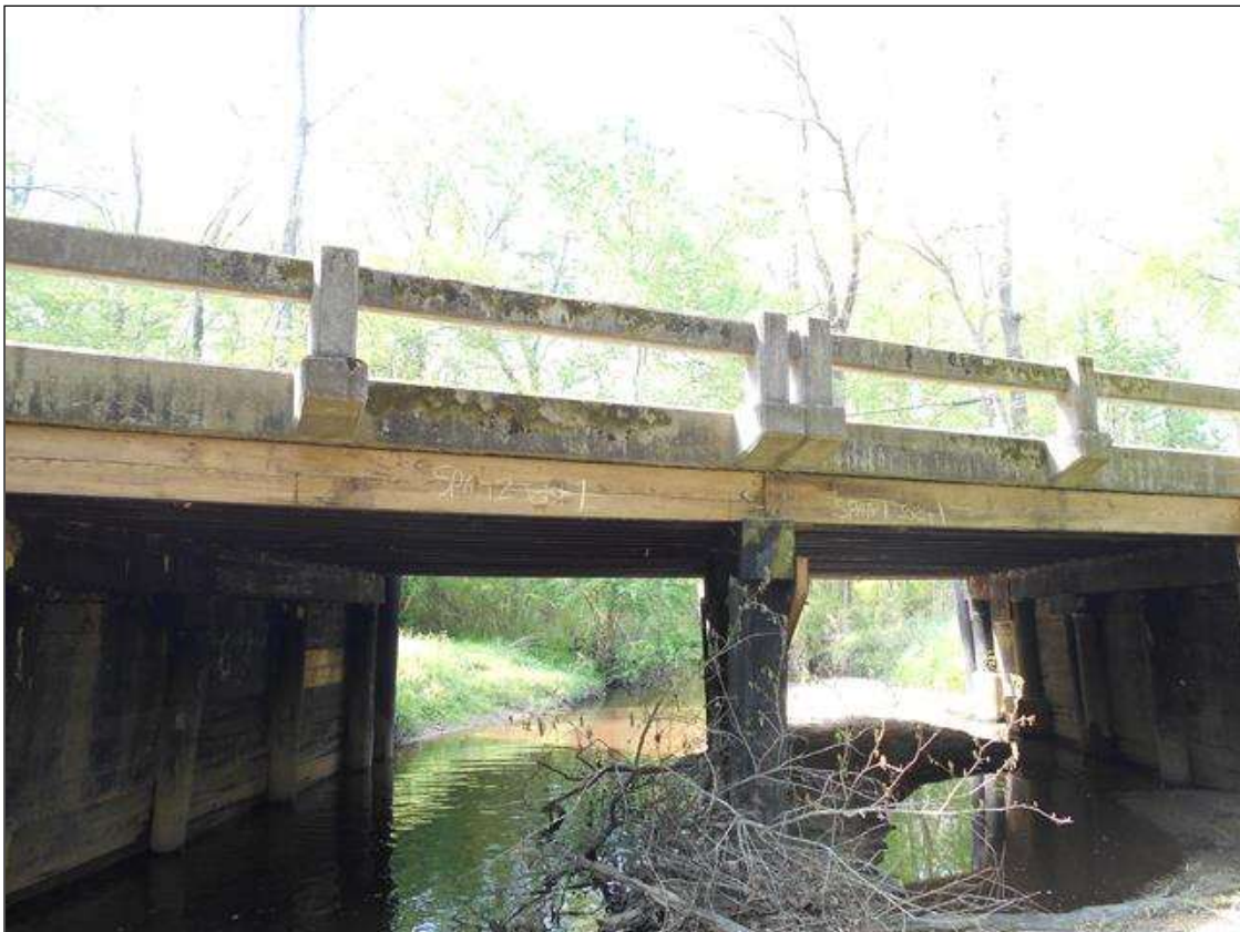
REPLACED JOIST 1 IN SPAN 1 AND SPAN 2
