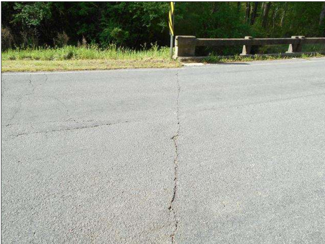
TRANSVERSE CRACK IN ASPHALT WEARING SURFACE OVER END BENT 2
