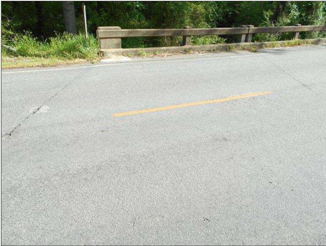
ASPHALT WEARING SURFACE TOP OF DECK SPAN 1
