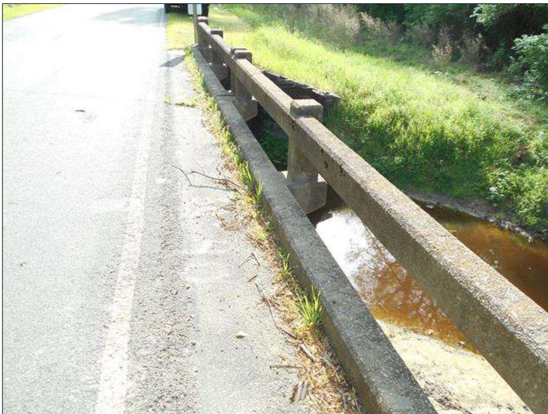
DIRT AND DEBRIS AND VEGETATION ALONG RIGHT SIDE WHEELGUARD ( LEFT SIDE SIMILAR )
