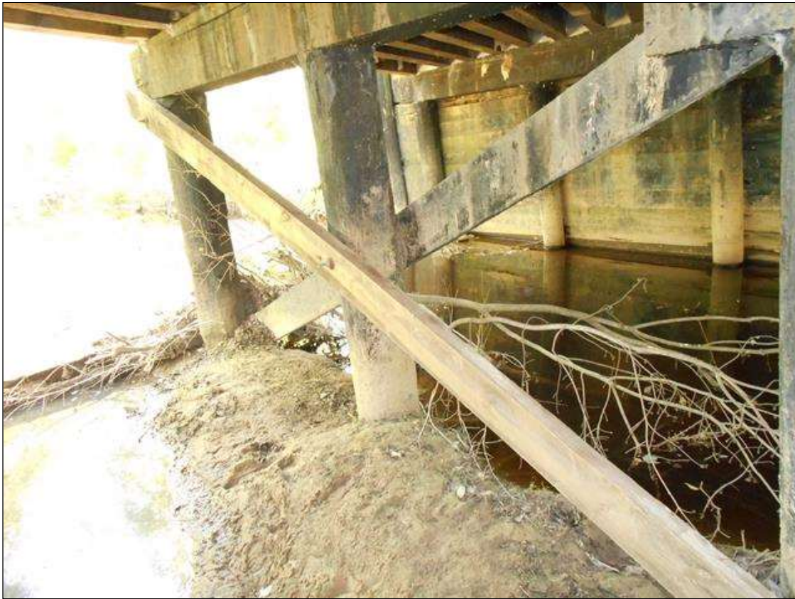
REPLACED CROSS BRACING @ INTERIOR BENT 1 SPAN 1 SIDE
