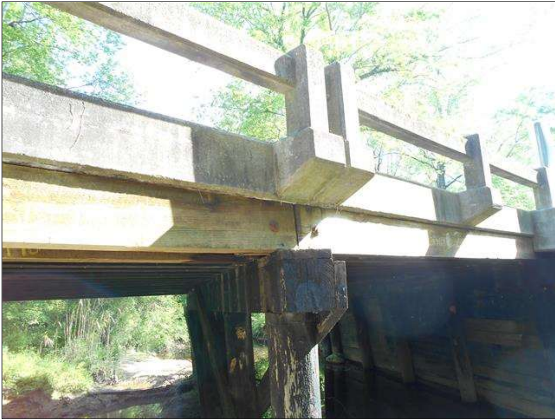
SUPERSTRUCTURE OVER INTERIOR BENT 1 RIGHT SIDE
