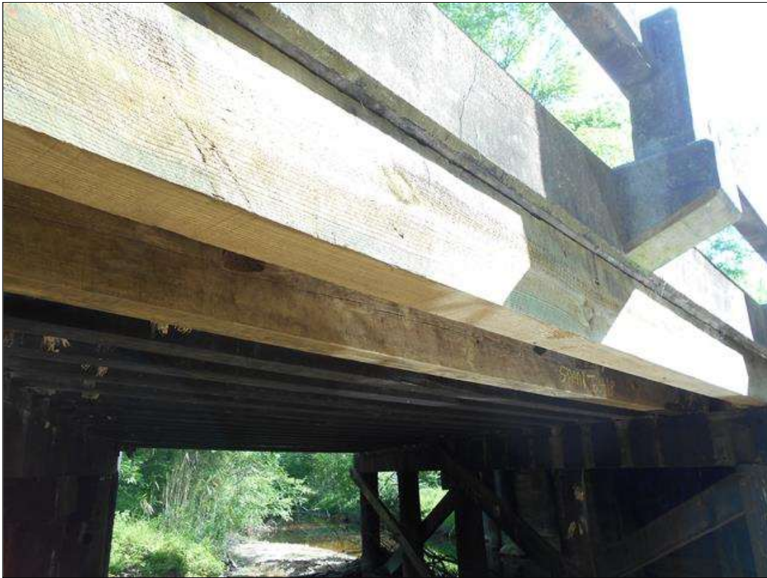
REPLACED JOIST 18 AND 19 SPAN 1 ( JOIST 19 IN SPAN 2 )
