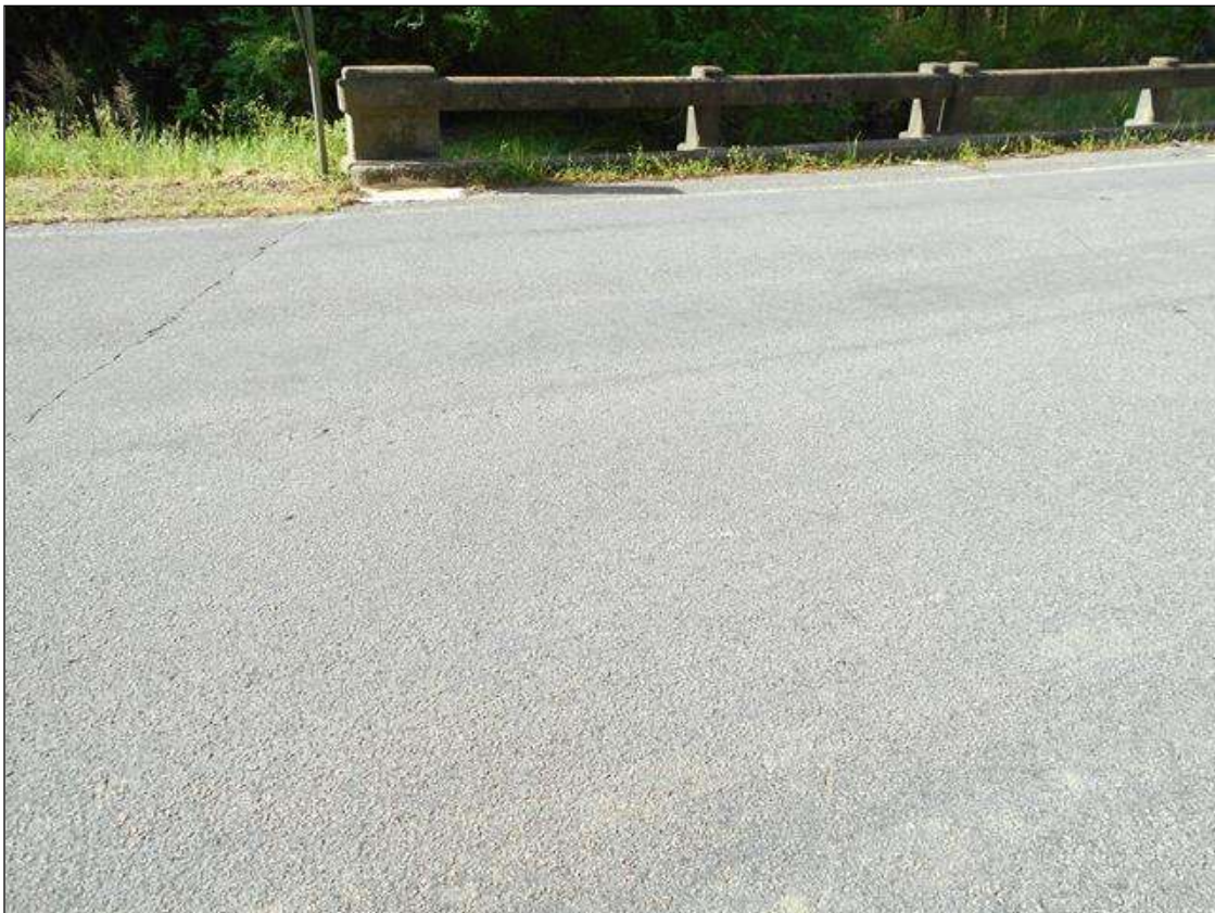
ASPHALT WEARING SURFACE TOP OF DECK SPAN 2
