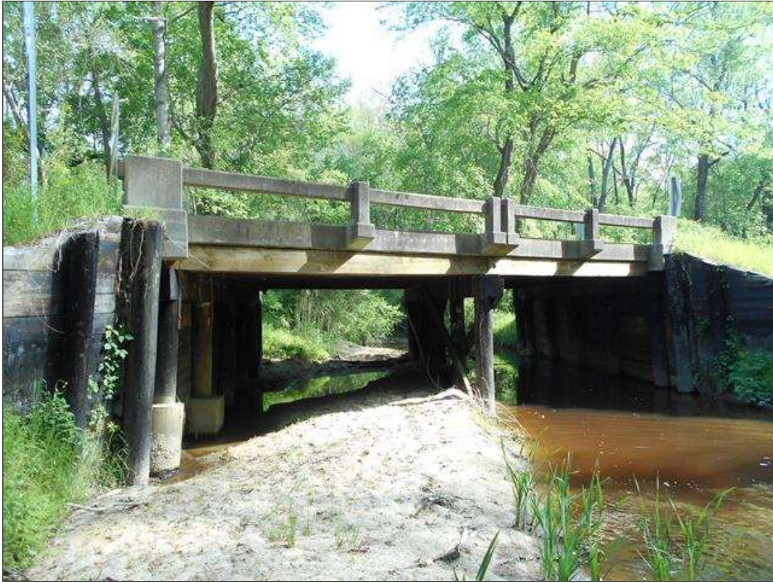
SOUTH SIDE LOOKING UPSTREAM
