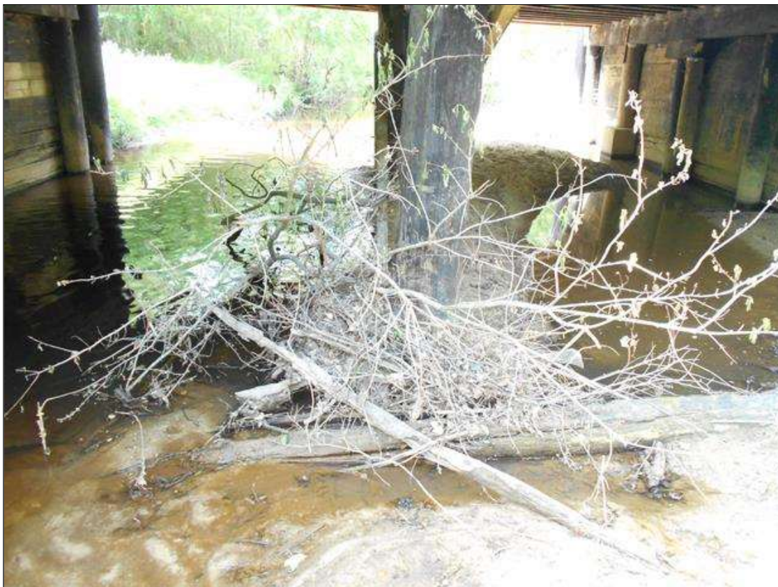
DRIFT AROUND BASE OF INTERIOR BENT 1
