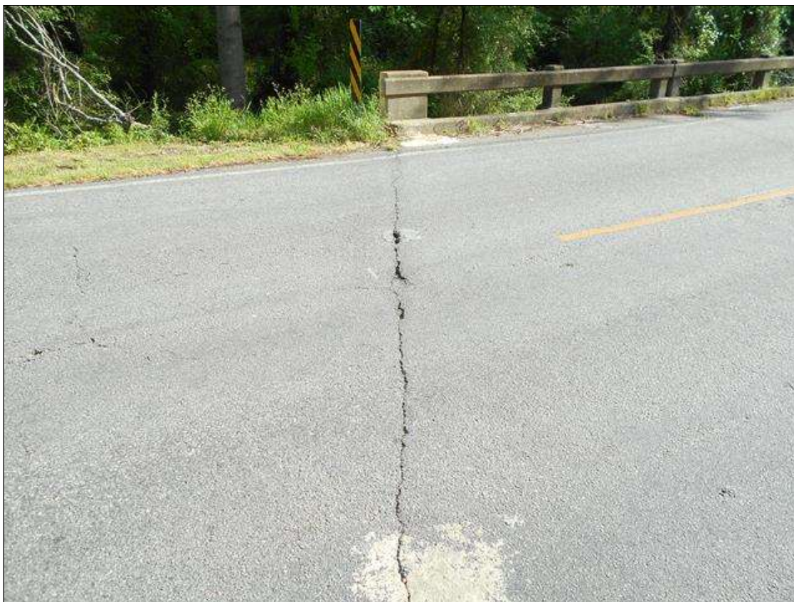
TRANSVERSE CRACK IN ASPHALT WEARING SURFACE OVER END BENT 1
