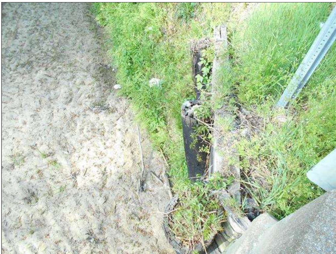
DECAY IN WINGWALL PILES @ SOUTH WEST CORNER WINGWALL WITH VEGETATION IN TOPS
