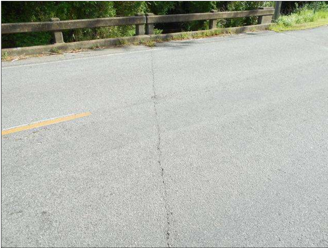
TRANSVERSE CRACK IN ASPHALT WEARING SURFACE OVER INTERIOR BENT 1
