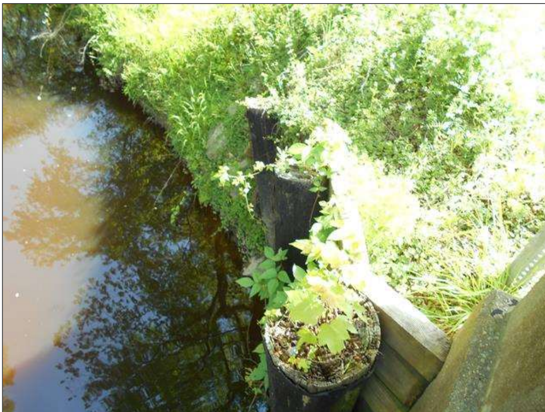
DECAY IN WINGWALL PILES @ NORTH EAST CORNER WINGWALL WITH VEGETATION IN TOPS
