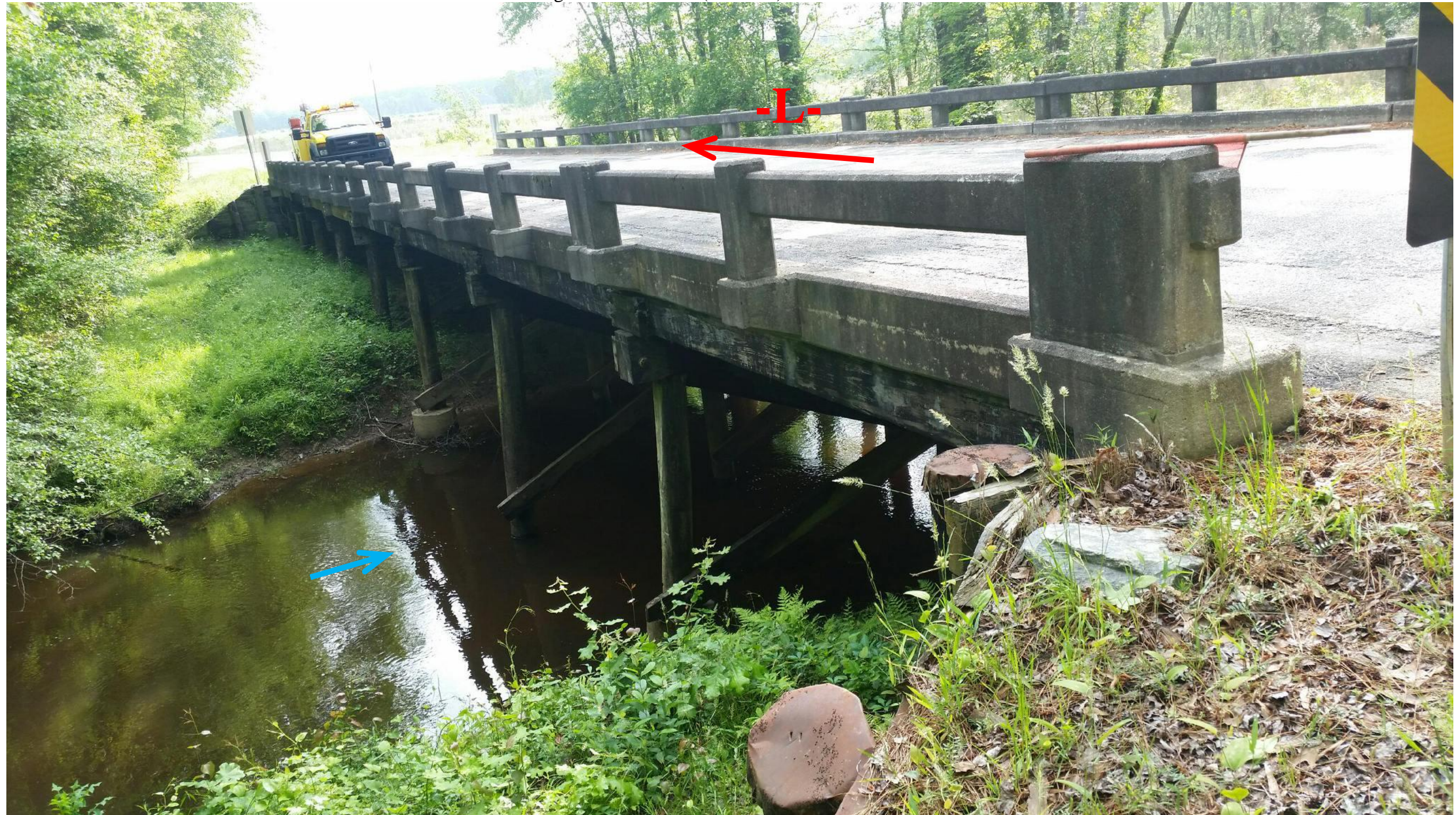
Looking Northeast towards End Bent 2
