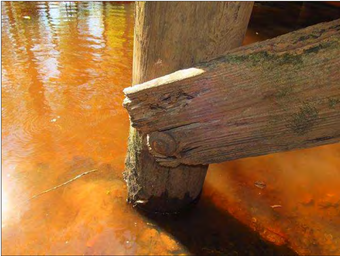
Decay in end of lower crossbrace for Pile 4 at Bent 3 span 4 side
