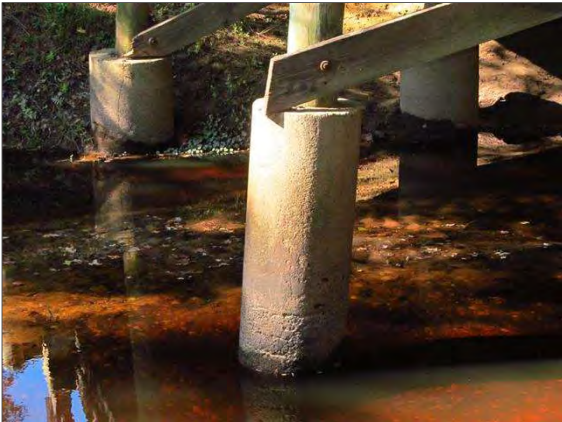
Temporary pile repairs throughout structure
