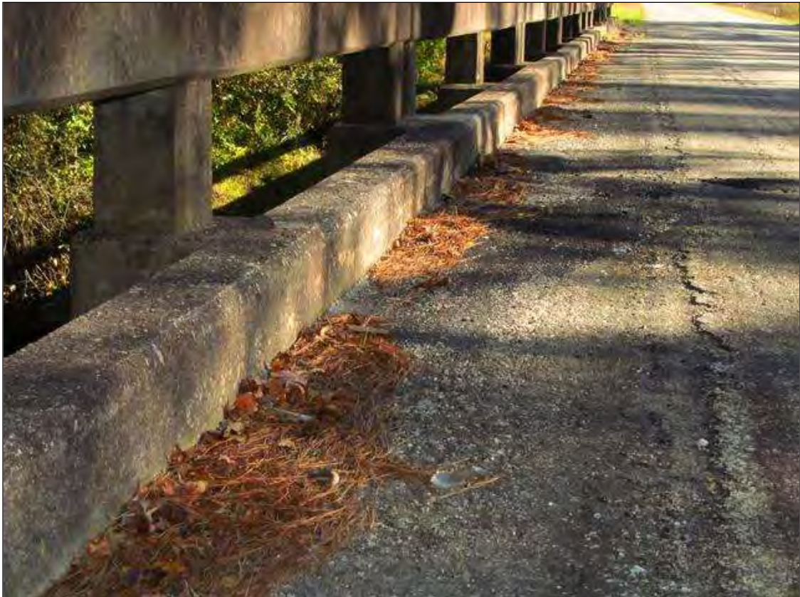
Dirt and debris along curblines
