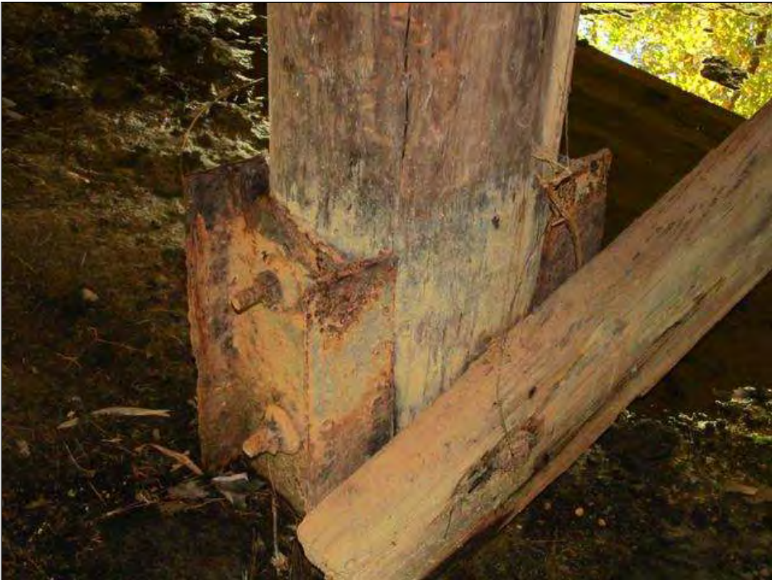
Temporary Repair for Pile 2 at Bent 6
