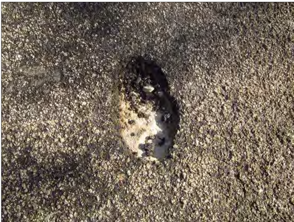
10" Diameter x 1.5" deep void pothole in the Northbound lane of Span 4
