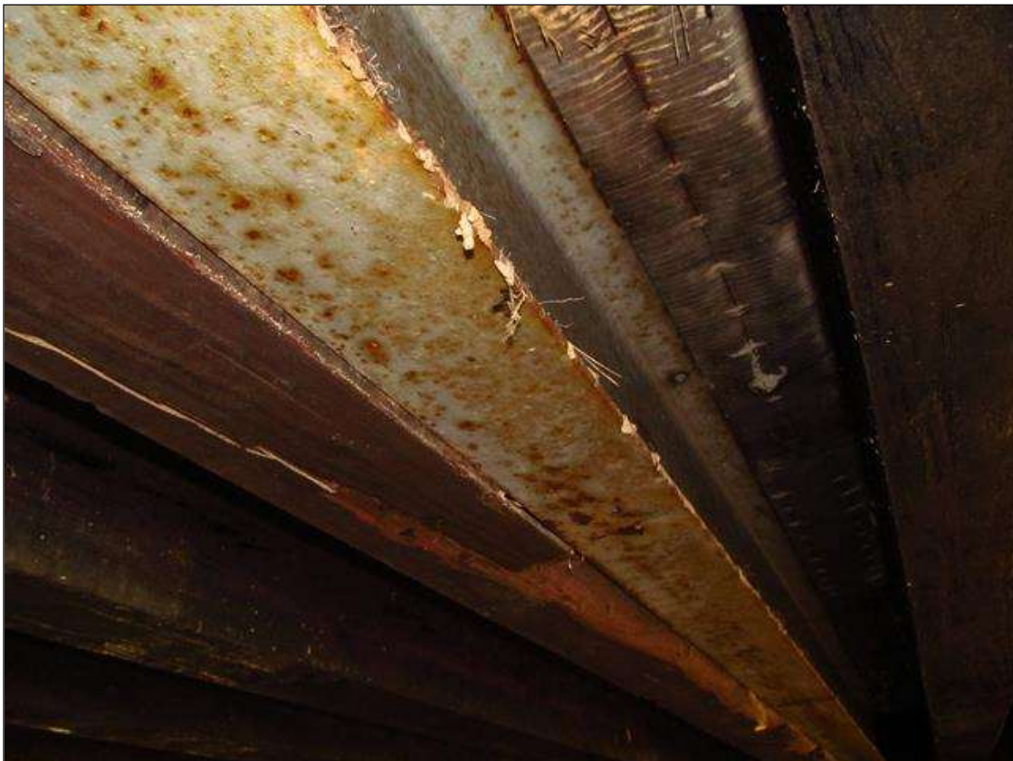
Existing steel beam (beam 12) at the Right side of beam 11
