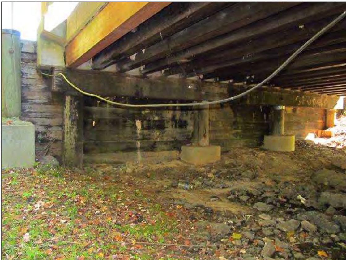
End Bent 2 overview
