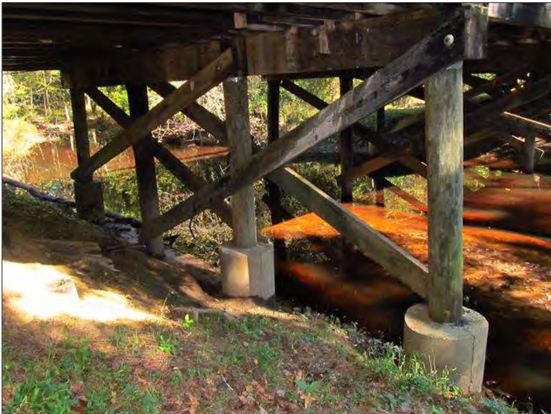
Bent 1 Span 1 side
