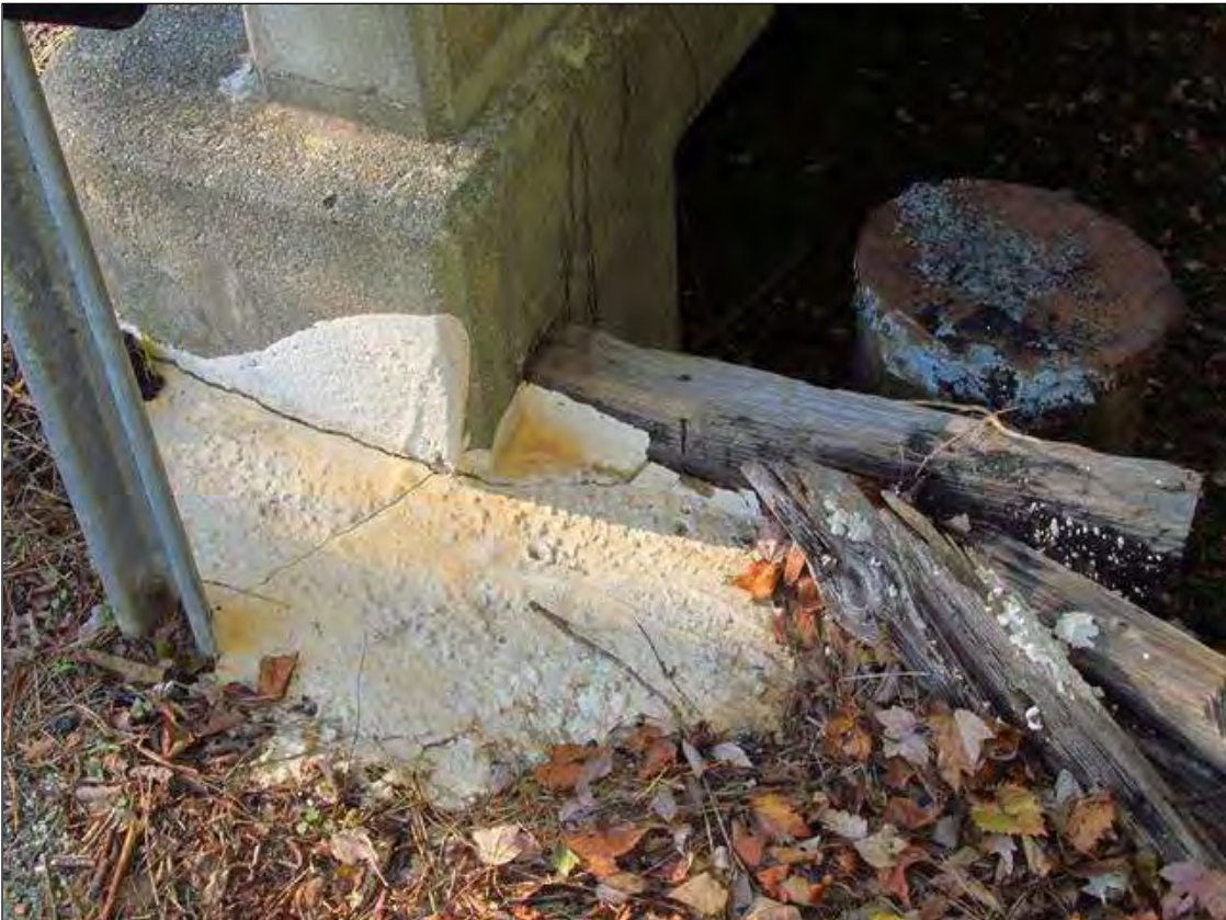
Grout Repair at the Left side of End Bent 2
