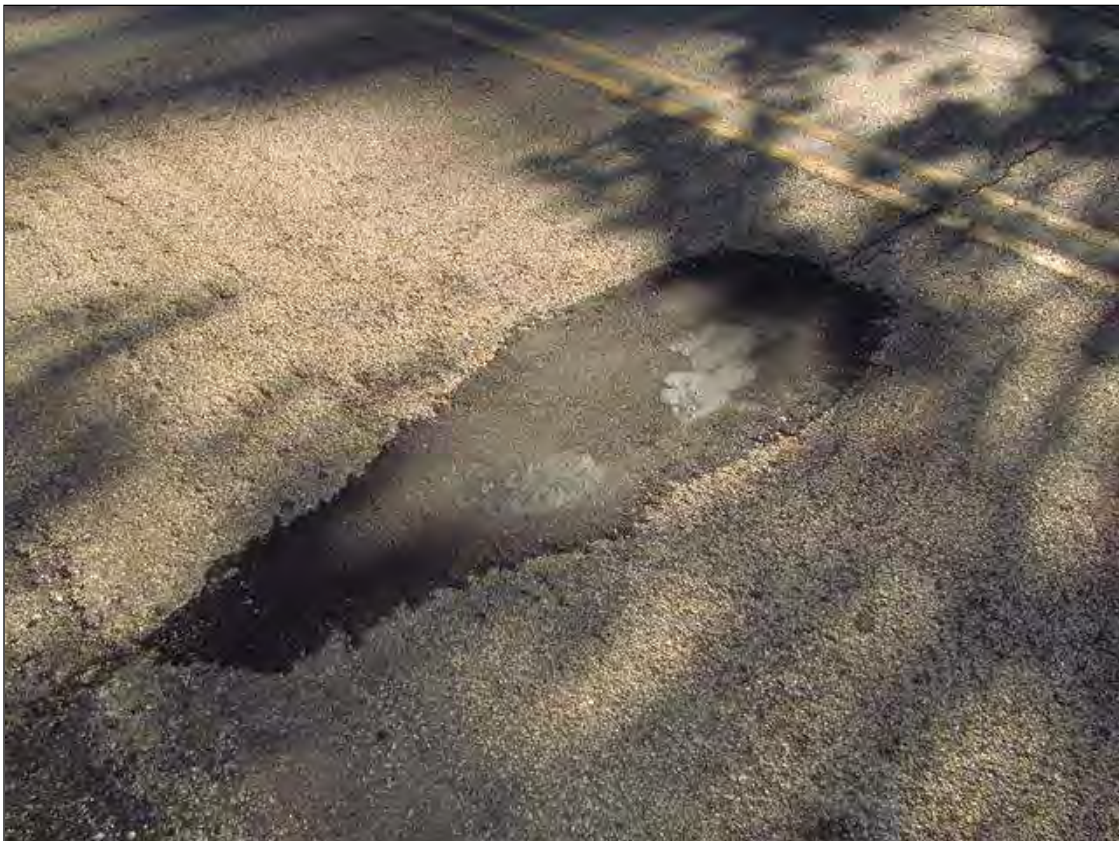
Asphalt patch in the Southbound lane over Bent 1
