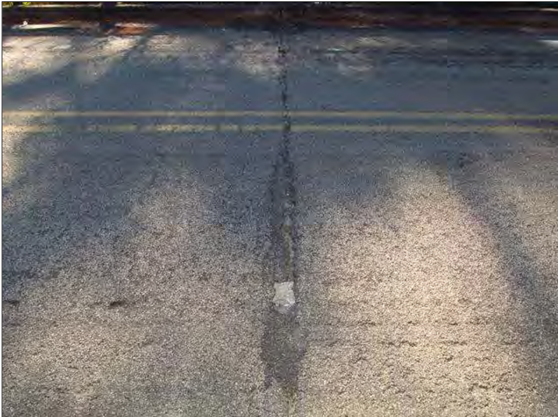
Cracking and separation in Asphalt wearing surface over Bent 2 - similar condition at other bents
