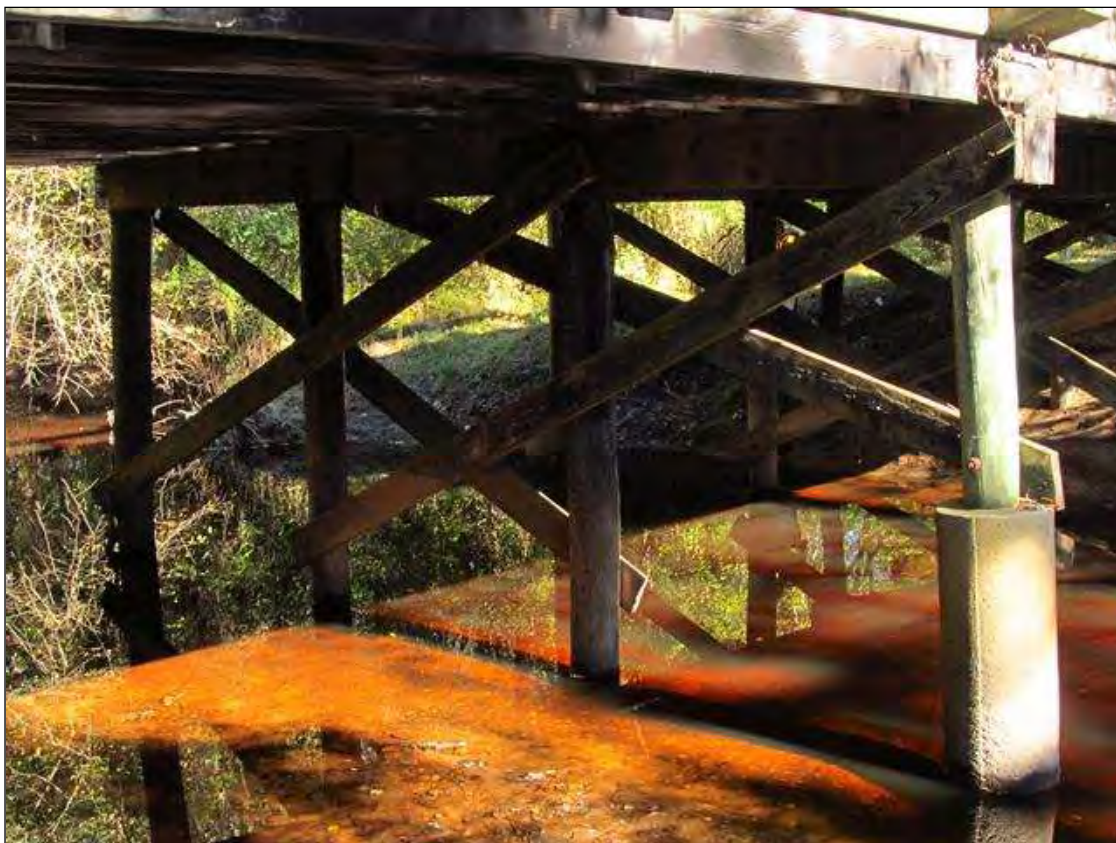
Bent 2 Span 2 side
