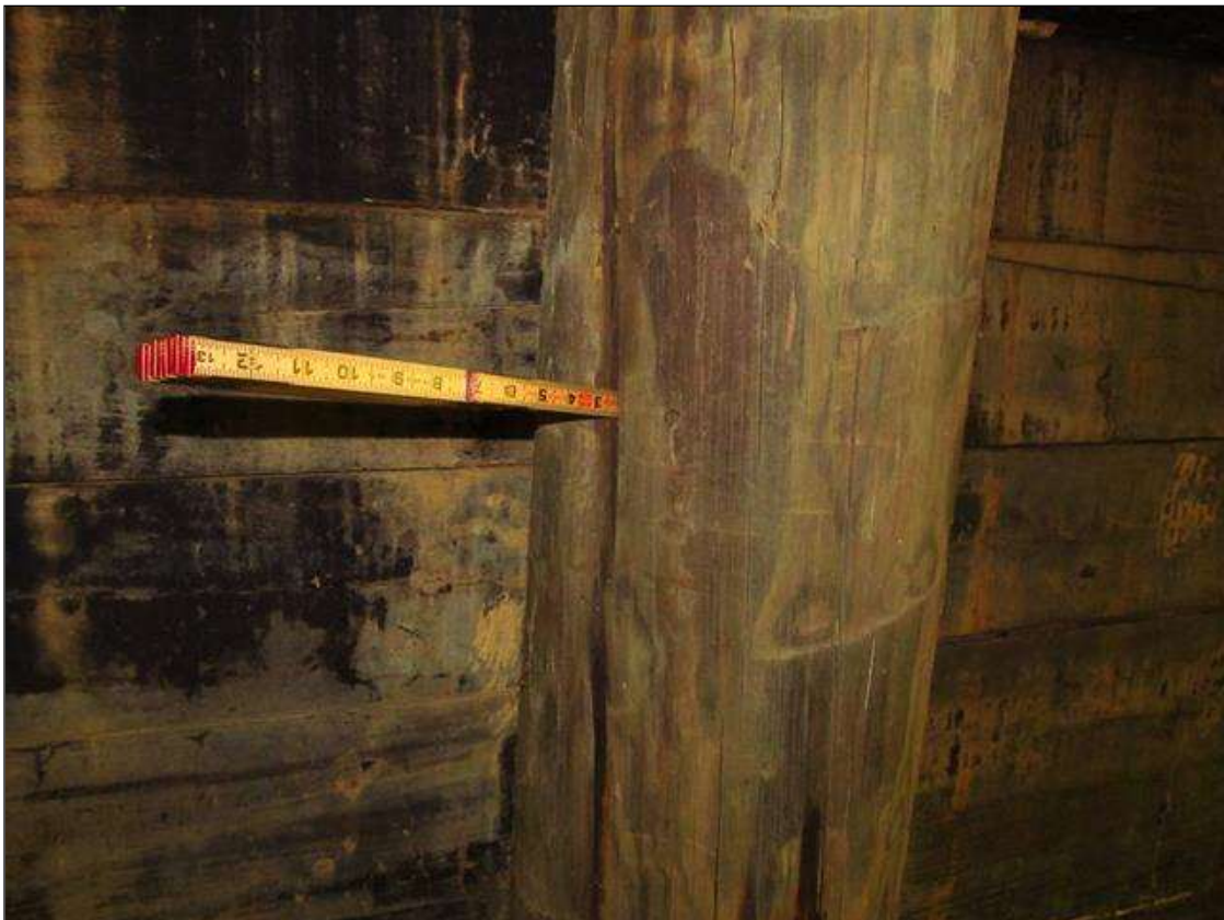
2-1/4" deep vertical check in Pile 2 at End Bent 2
