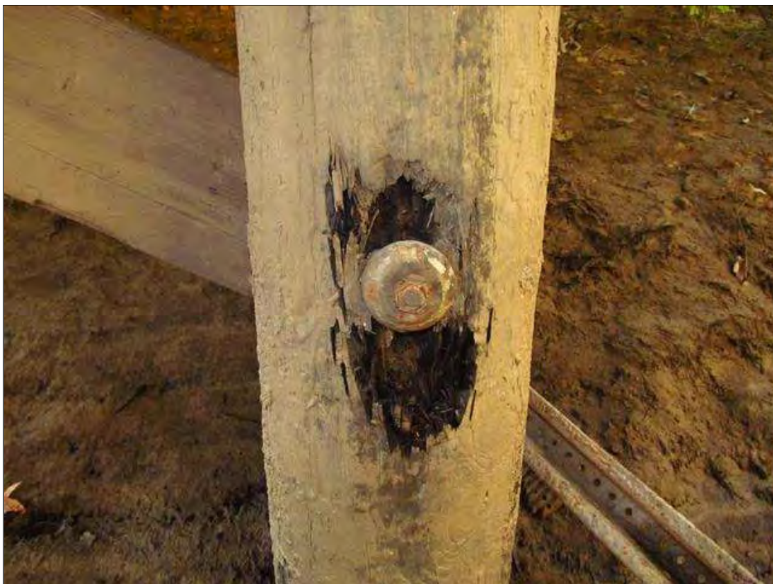
Decay in Span 2 side of Pile 2 at Bent 1 lower crossbrace connection - Pile 1 at Bent 2 similar
