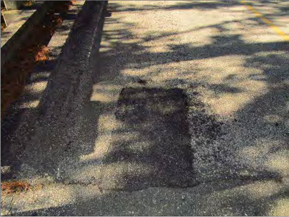
Asphalt patch in the Northbound lane at End Bent 2
