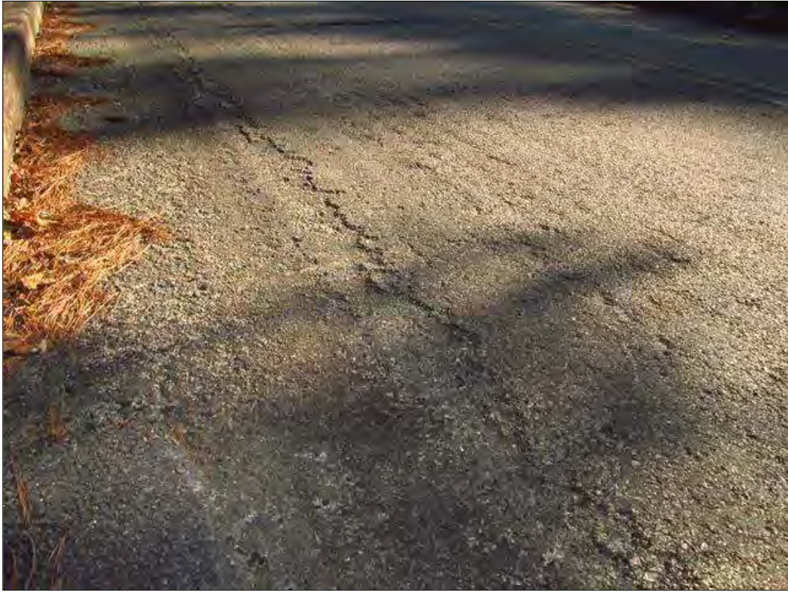
Longitudinal bands of deterioration in Span 1 Asphalt wearing surface - All spans similar
