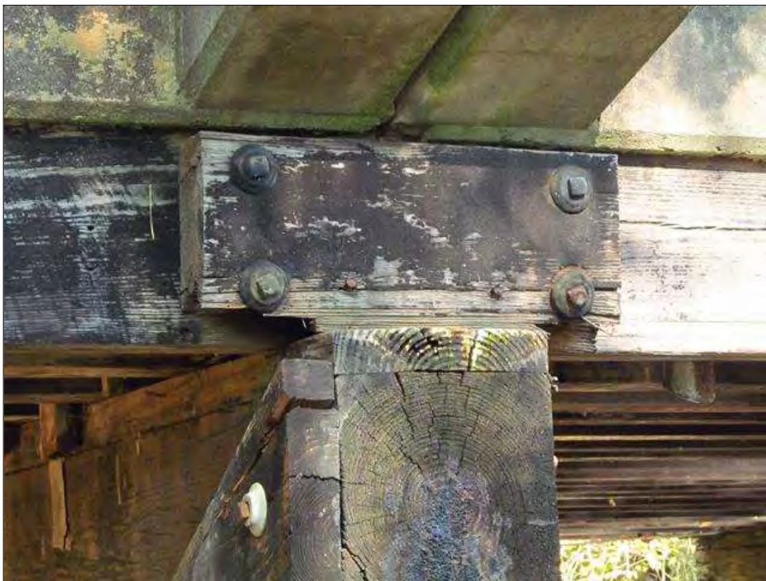
Superstructure over End of cap at Bent 1 - Other bents similar
