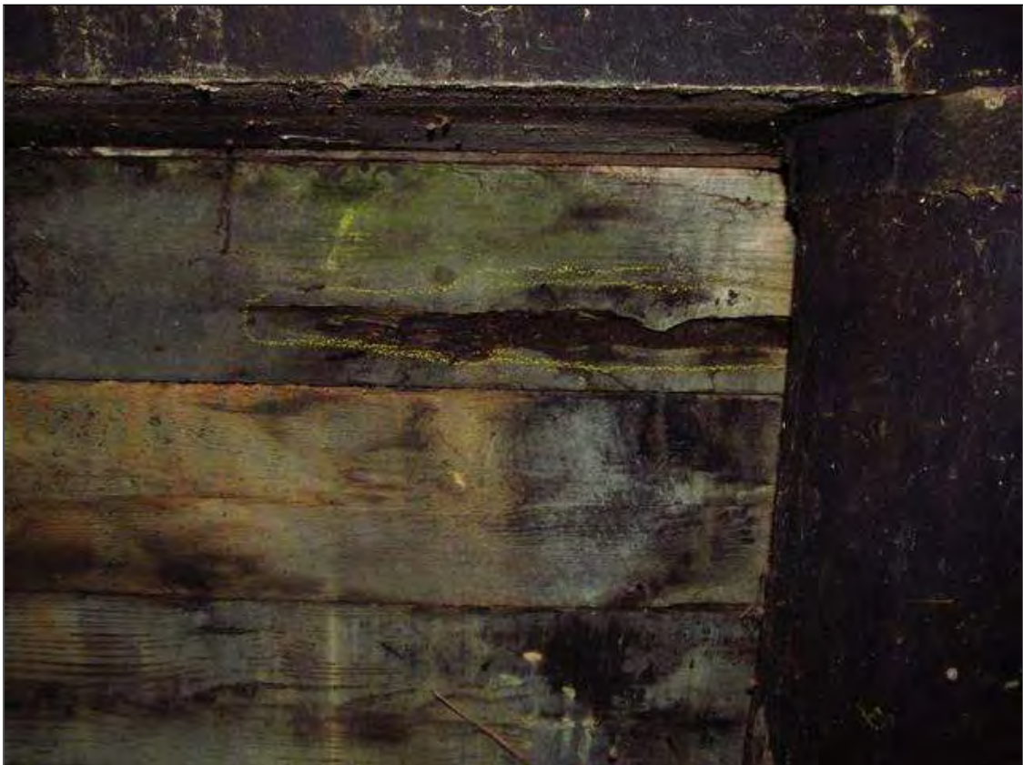
Rot areas of decay in Bulkhead boards at End Bent 1
