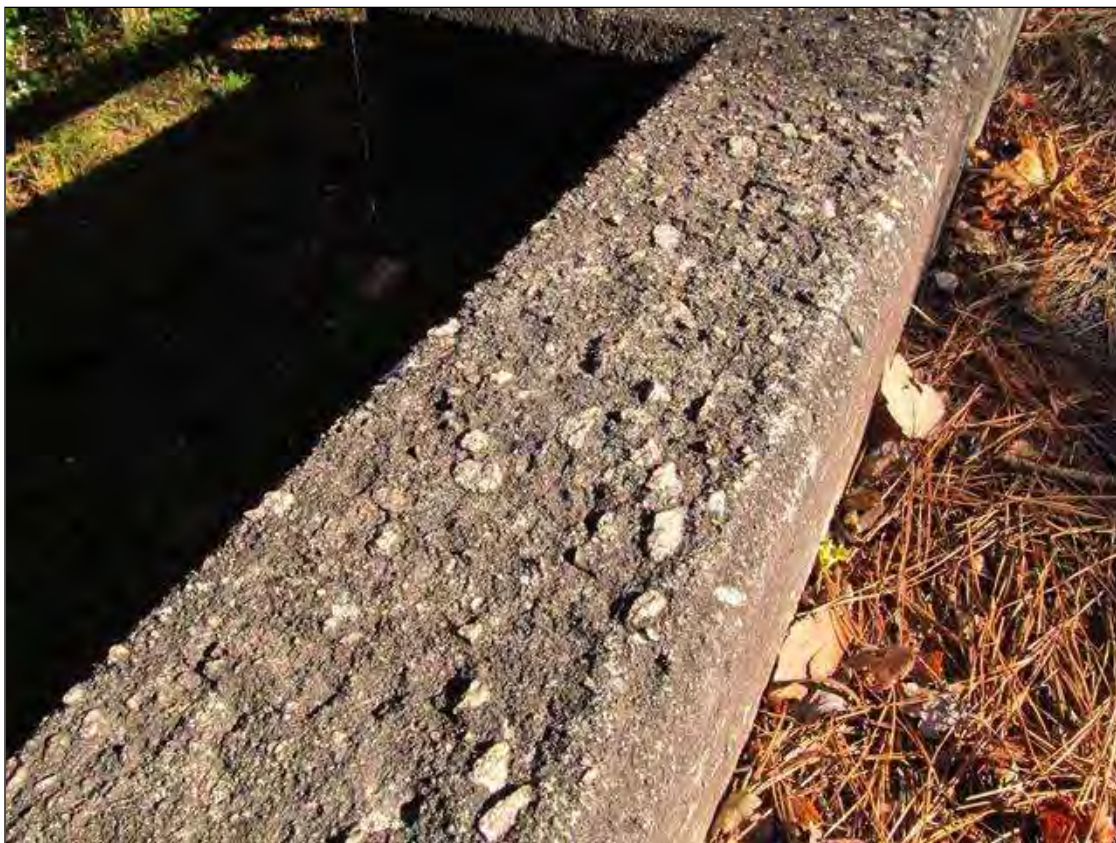
Abrasion with Coarse aggregate exposed along deck curbs
