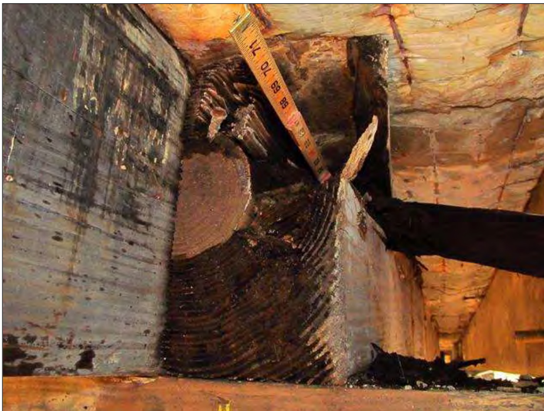
Decay in the end of Joist 18 in Span 5 over Bent 4 - Priority maintenance issued
