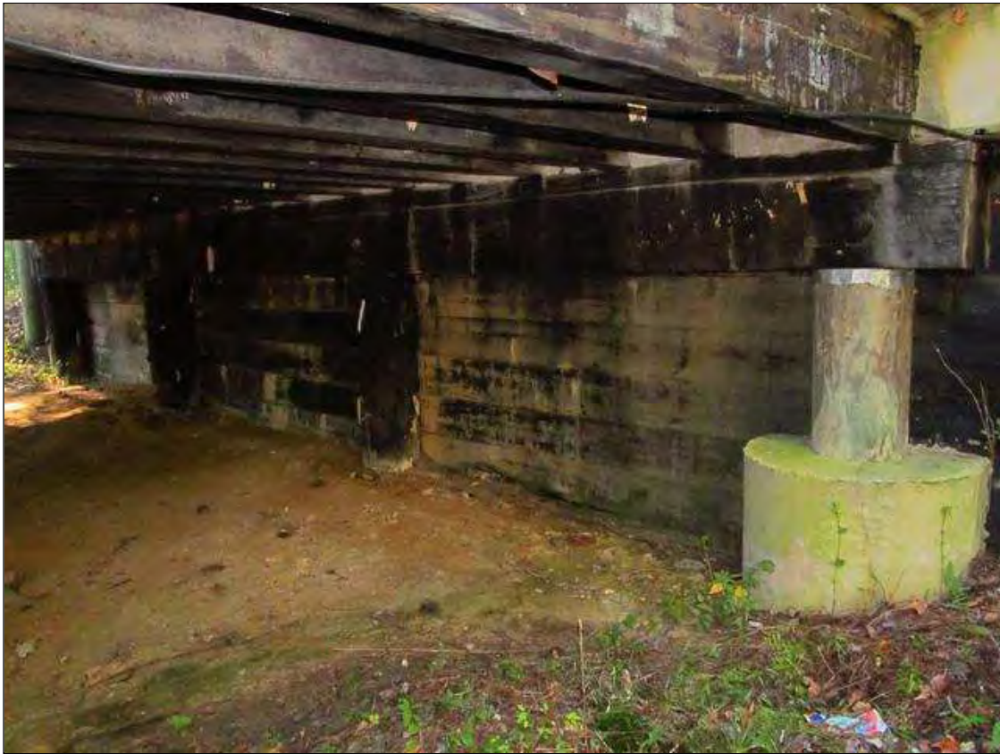
End Bent 1 overview
