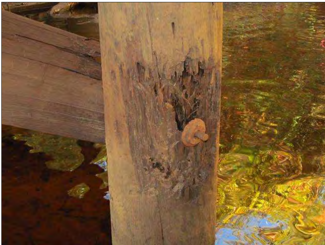
Decay in Span 3 side of Pile 2 at Bent 2 lower crossbrace connection
