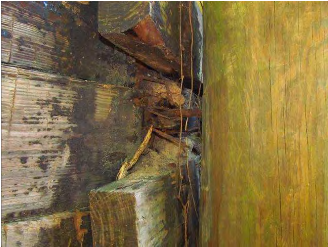
2nd Bulkhead board from top at End Bent 2 decayed and missing from the left end to left end of cap
