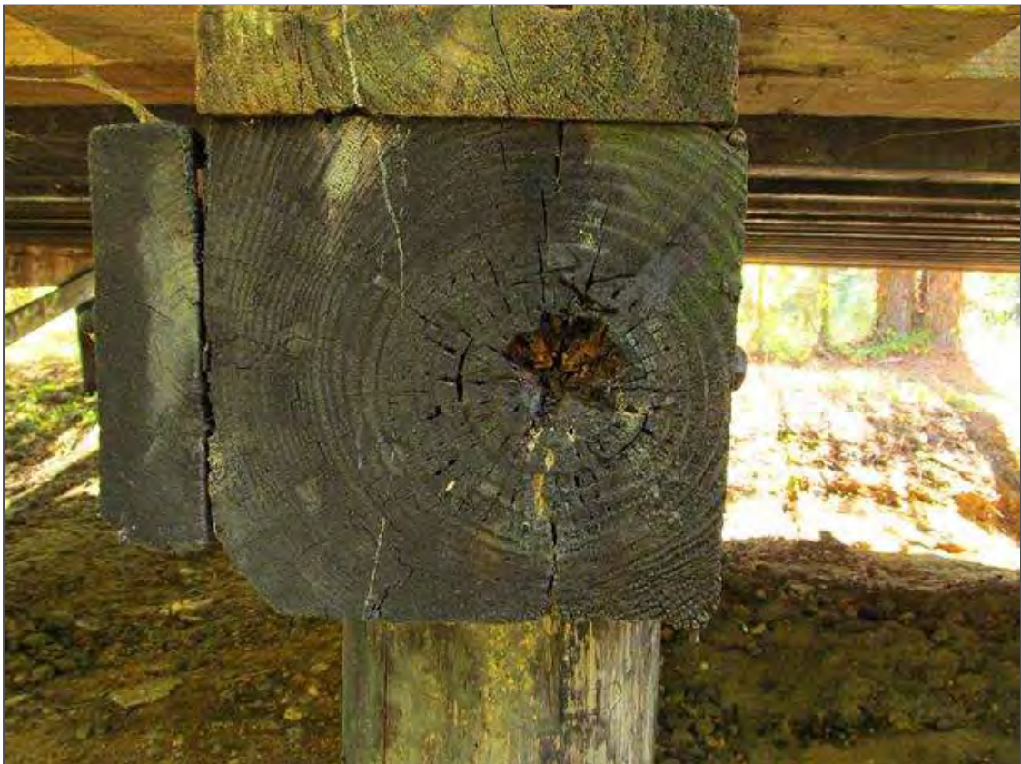
Decay in left End of cap at Bent 5
