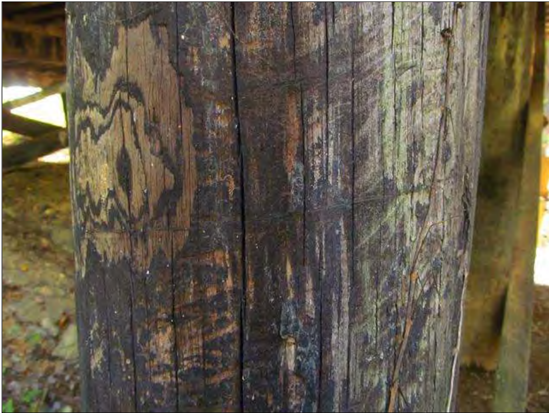
Random vertical checking throughout all timber piles
