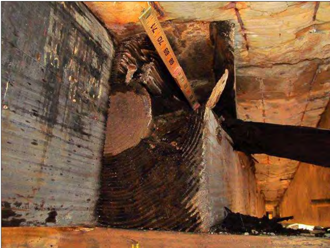
5.5 FT. DEEP DECAY IN THE END OF JOIST 18 IN SPAN 5 OVER BENT 4
