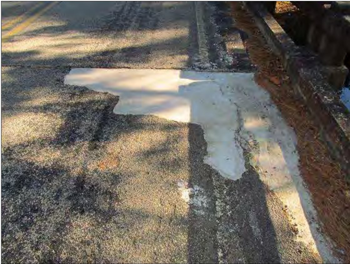
Concrete patch in the Northbound lane and shoulder of Span 1
