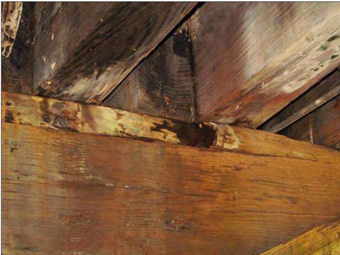
Decay in Bent 3 crownstrip span 4 side at Joist 2
