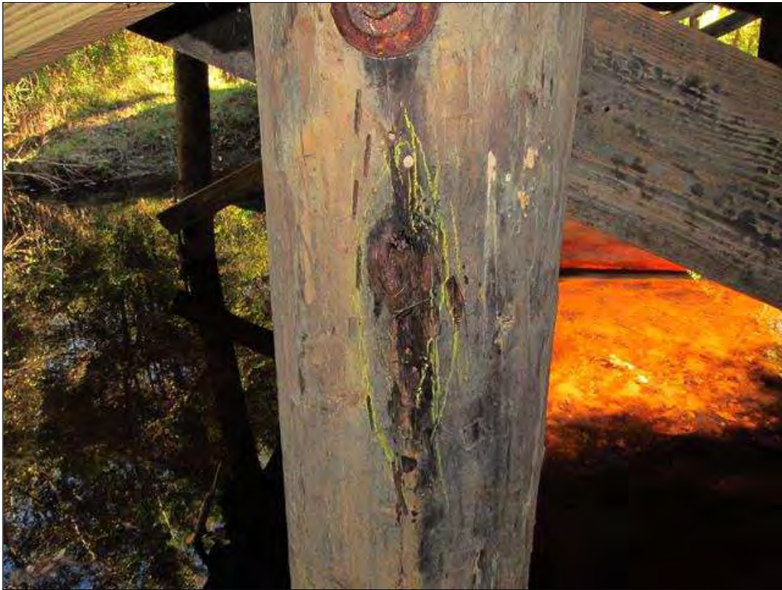
Decay in Span 1 side of Pile 2 at Bent 1
