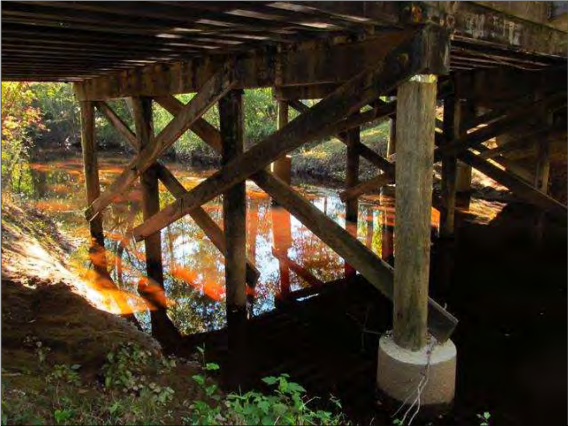
Bent 3 span 4 side
