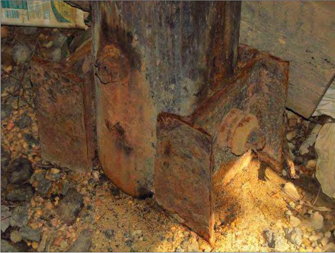
Temporary repair for Pile 3 at Bent 5
