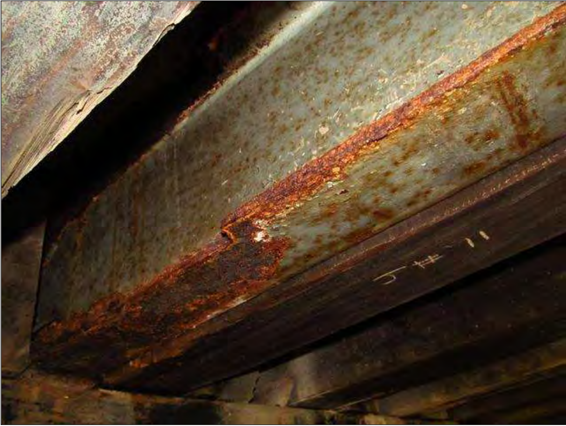
Section loss in the Bottom flange of beam 12 in Span 6 over Bent 5
