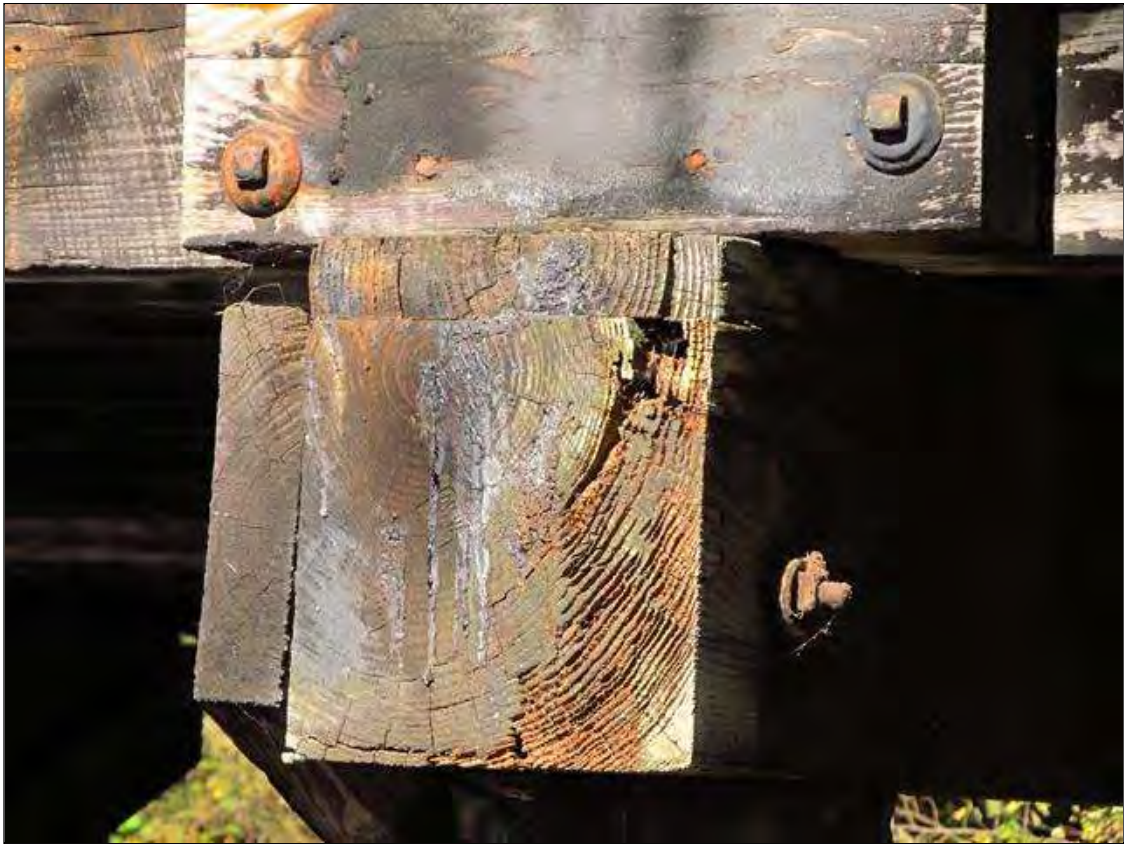
Decay in right End of cap at Bent 3
