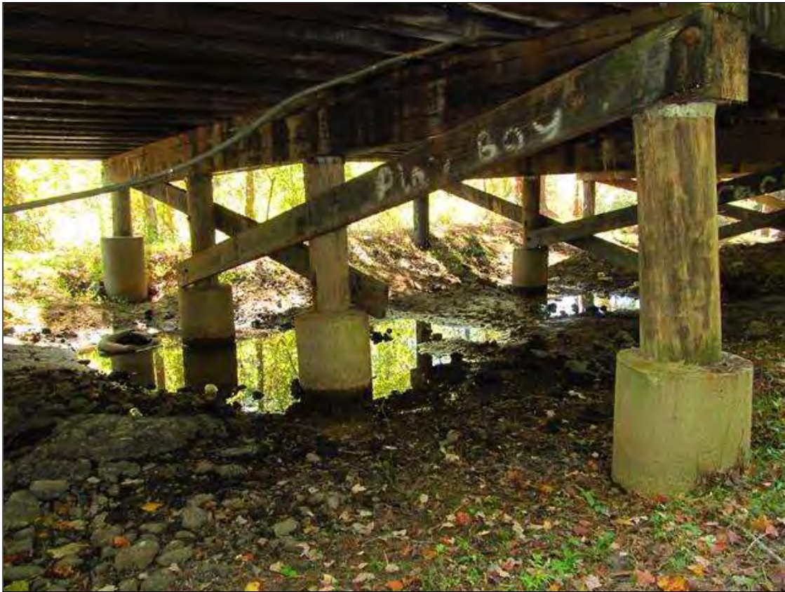
Bent 7 Span 8 side
