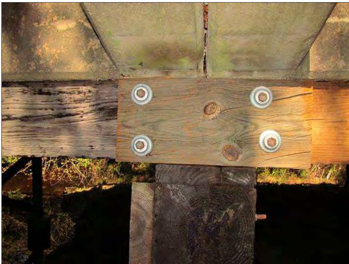
New splice block has been added at the Right side of Bent 4 - Others similar
