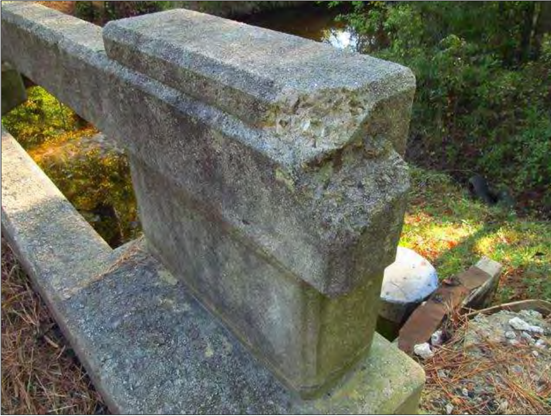
Right guardrail endpost at End Bent 1 spalled
