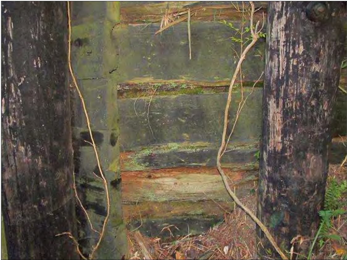
Decay and separation in the Left side Wingwall boards at End Bent 1
