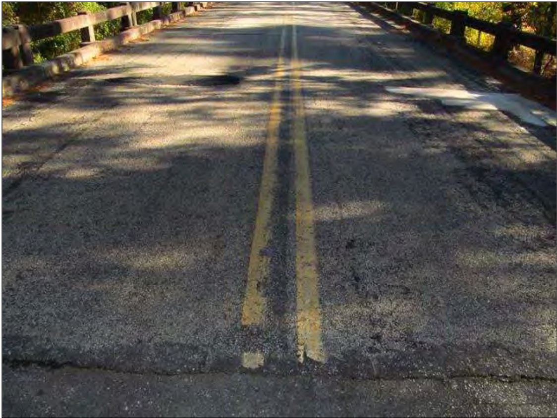
Span 1 overview - Other spans similar
