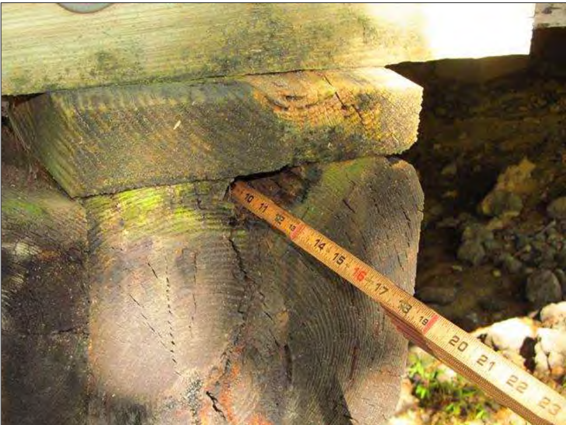
Decay in right End of cap at Bent 7
