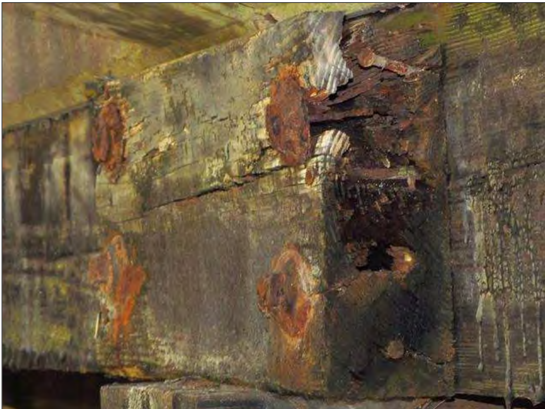
Decay in the Left side splice block at Bent 1 - Others similar
