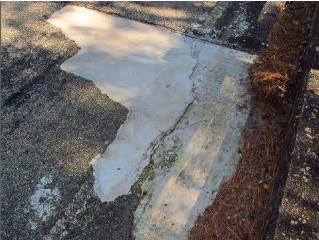
Concrete patch cracked and uneven in the Northbound lane of Span 1
