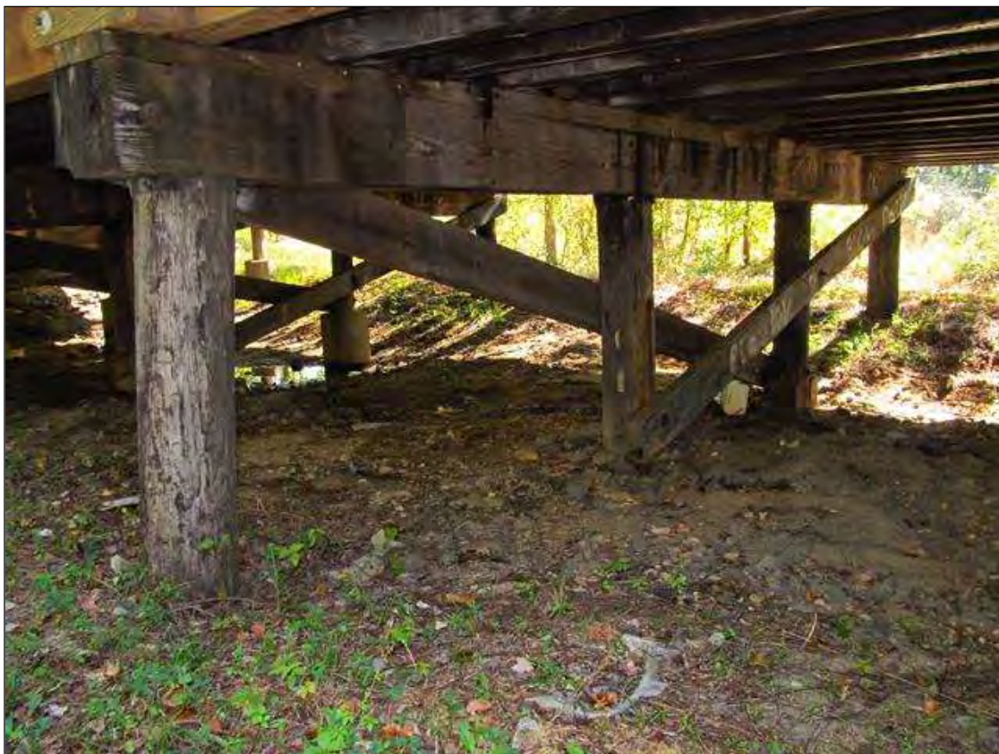
Bent 5 Span 5 side
