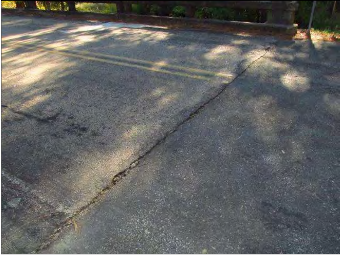
Transverse cracking in Wearing surface over End Bent 1
