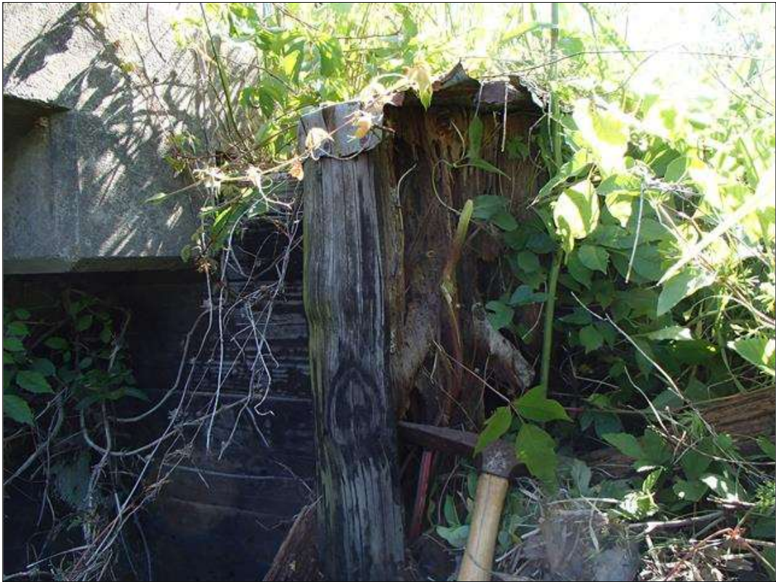
SOUTH EAST RETAINING PILE 100% DECAY
