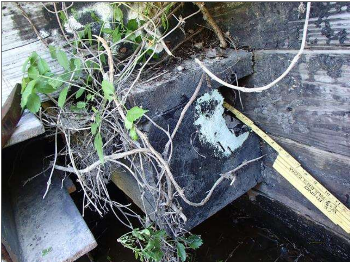
END BENT 2 RIGHT END OF CAP DECAY (BEYOND CRUTCH BENT)
