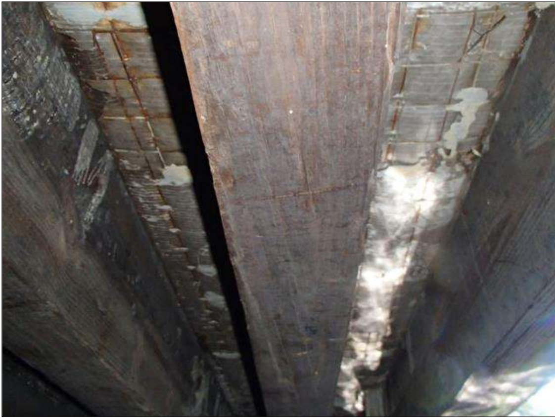
UNDERSIDE OF DECK SPAN 2
