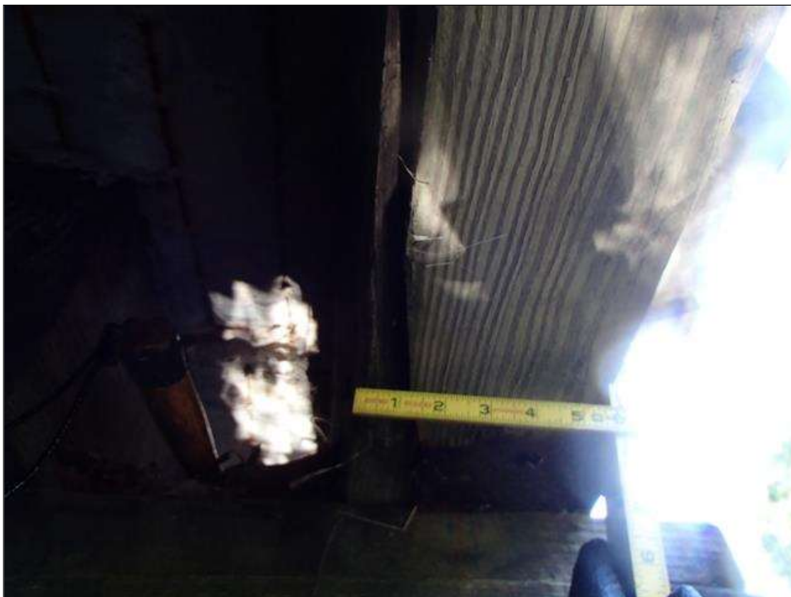
BEAM 19 SPAN 1 - 1" WIDE SPLIT OVER BENT 1 - 2' LONG
