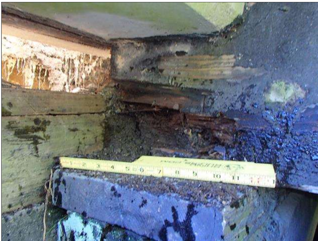
BEAM 1 AT END BENT 2 DECAYED (BEYOND CRUTCH BENT)
