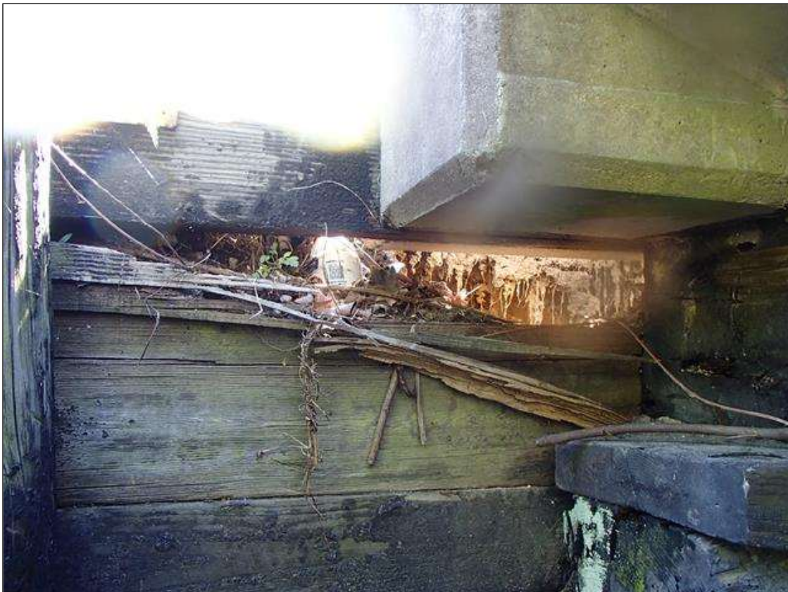
BULKHEAD BOARD 1 LEFT AT END BENT 2 MISSING 3'
