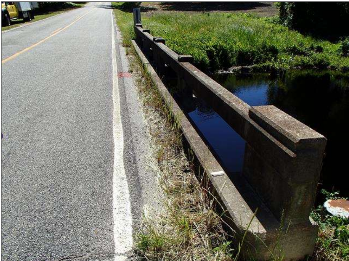
CURB AND RAIL OVERVIEW
