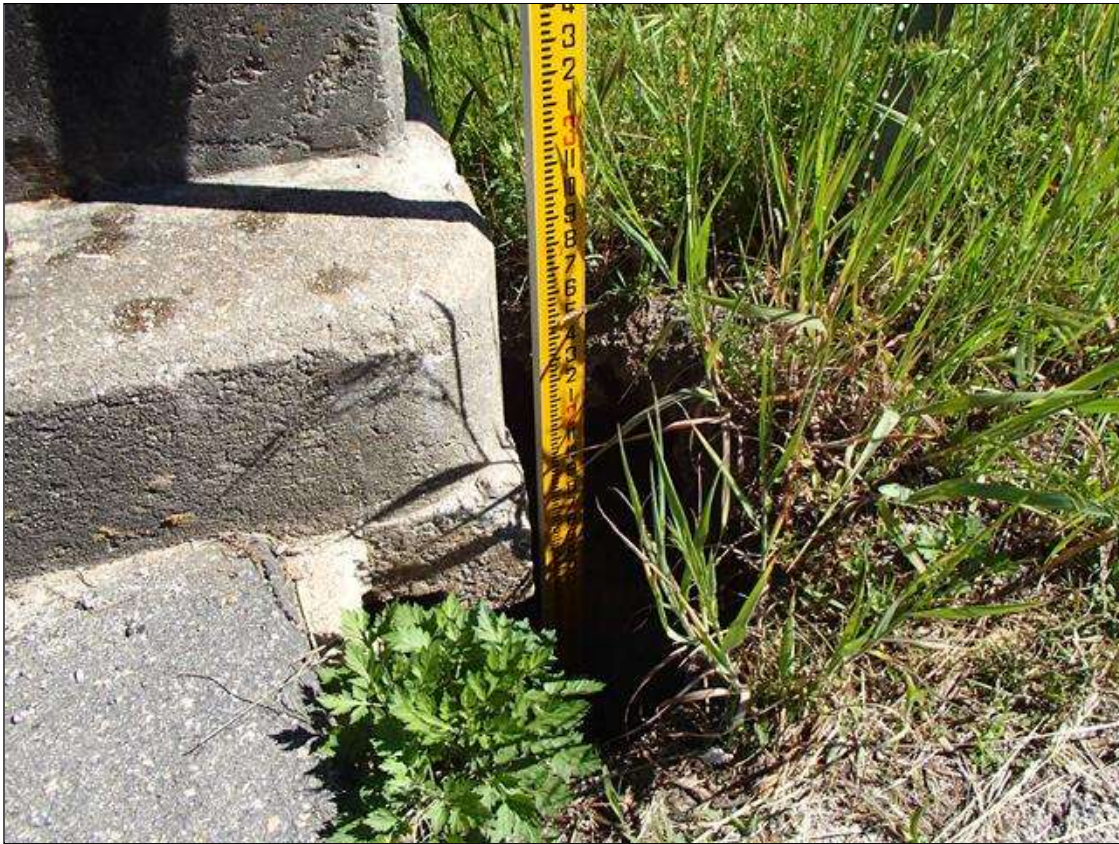
SINKHOLE NEAR NORTH EAST CORNER DOWN TO BULKHEAD BOARD #8
