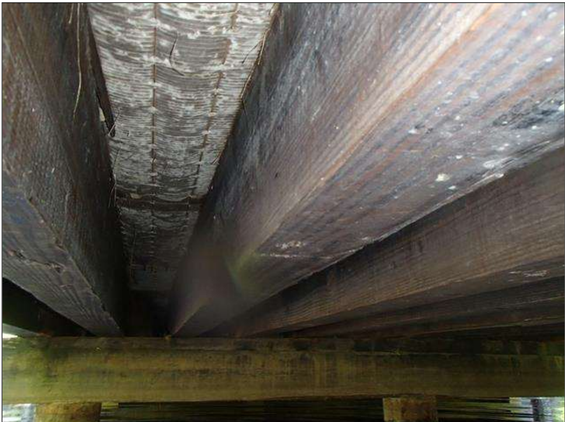
BEAM 3 SPAN 1 SHOWING CHECKS, TYPICAL
