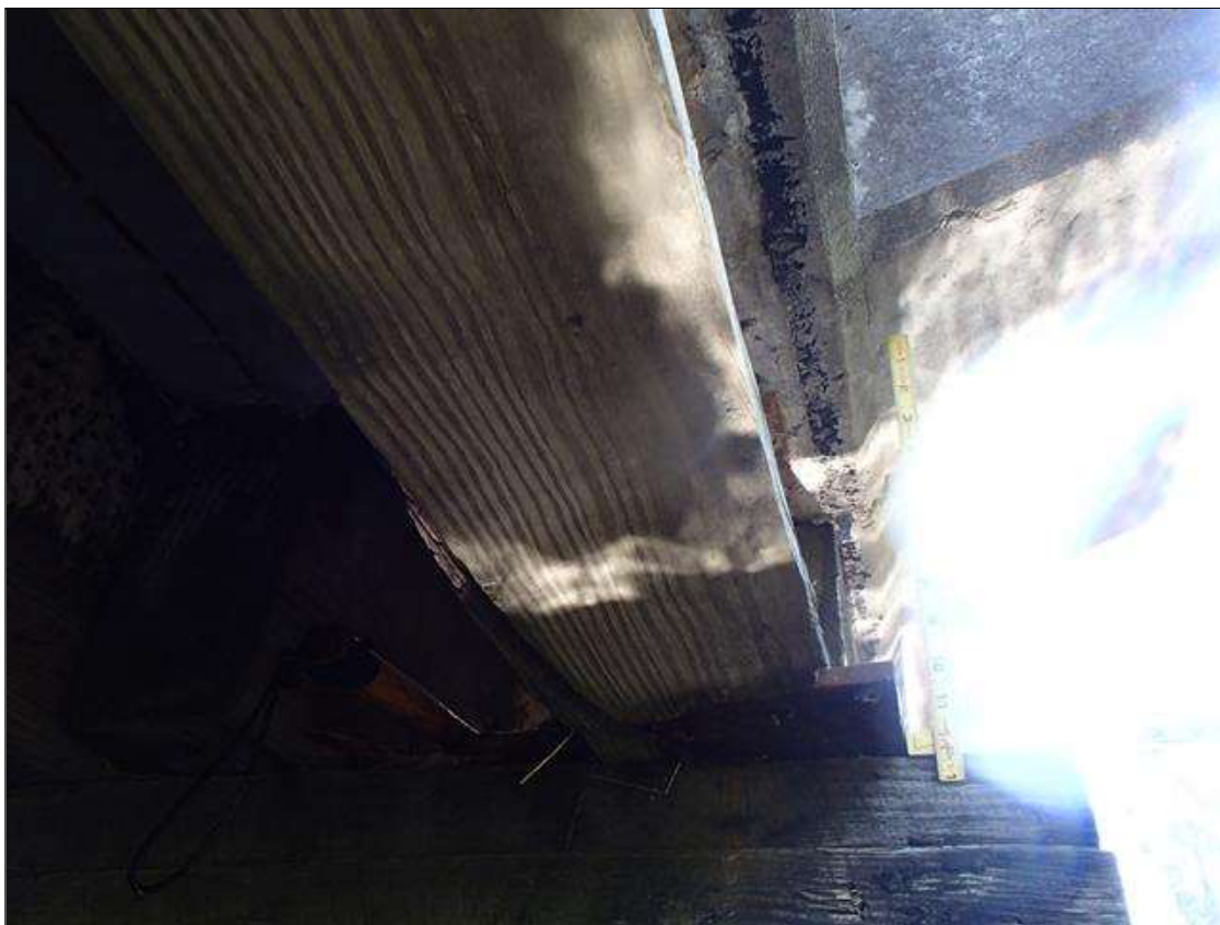
BEAM 19 SPAN 1 ROTATED INWARD 1.5" MIDSPAN BENT 1
