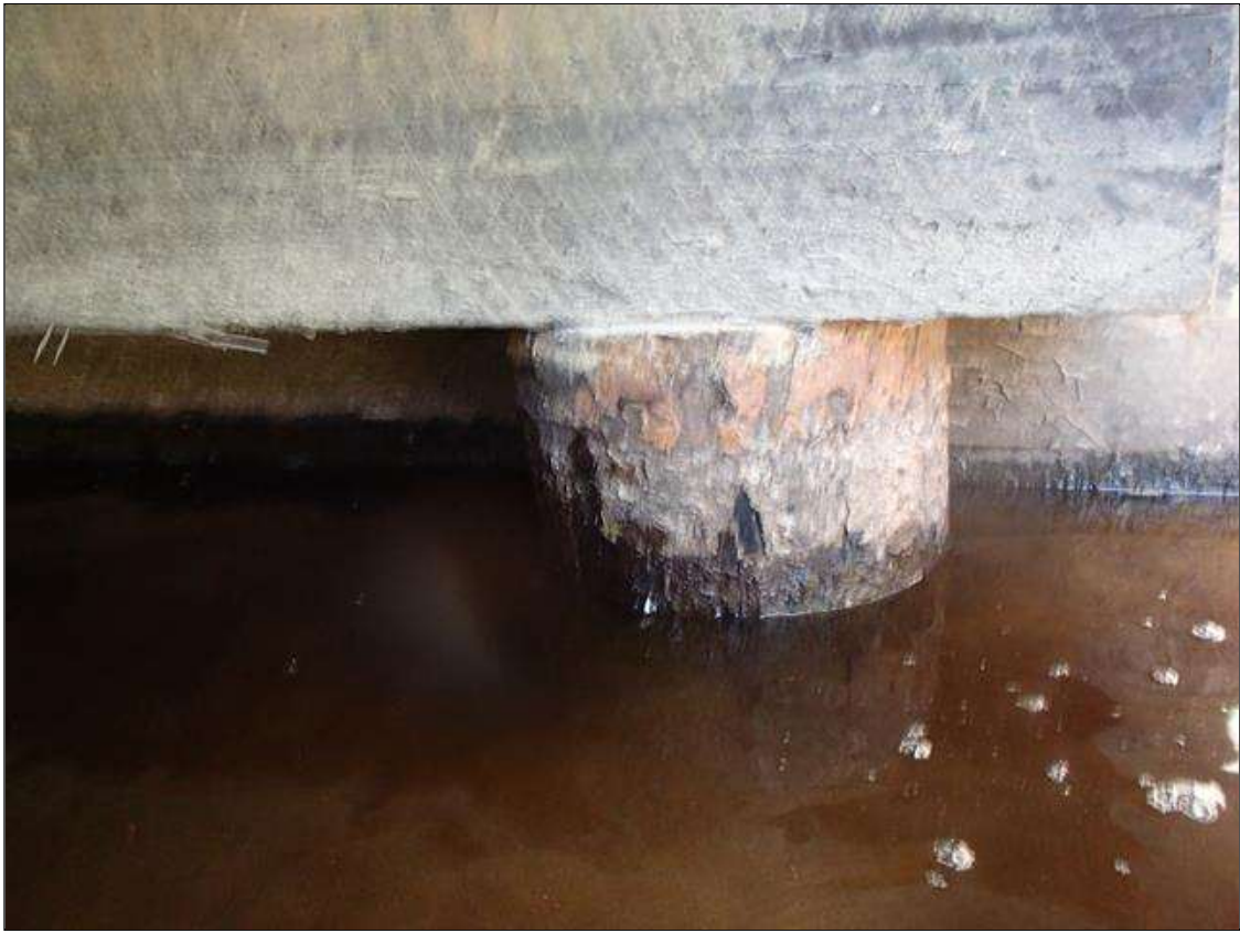
PILE 1 AT BENT 1
