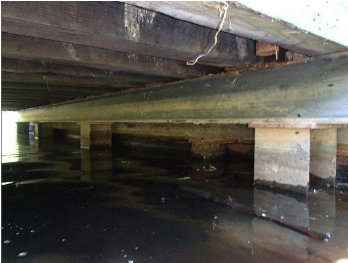
CRUTCH BENT AT END BENT 2
