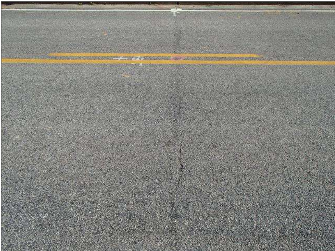
HAIRLINE CRACK IN AWS OVER BENT 1
