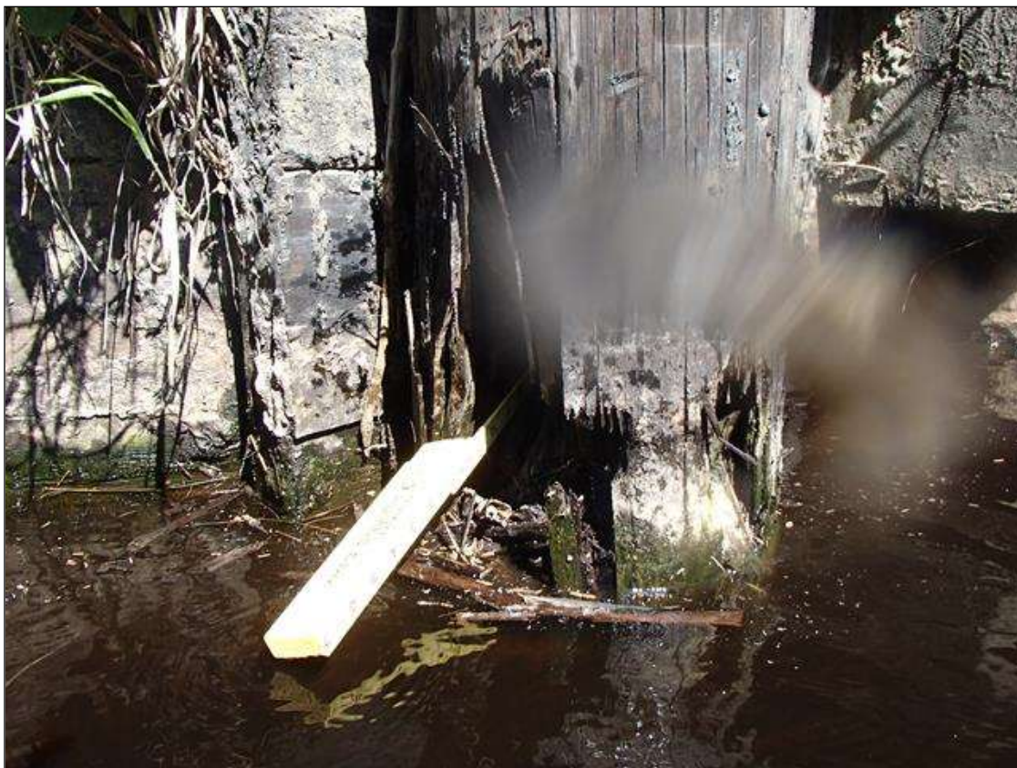
SOUTH WEST RETAINING PILE 100% DECAYED
