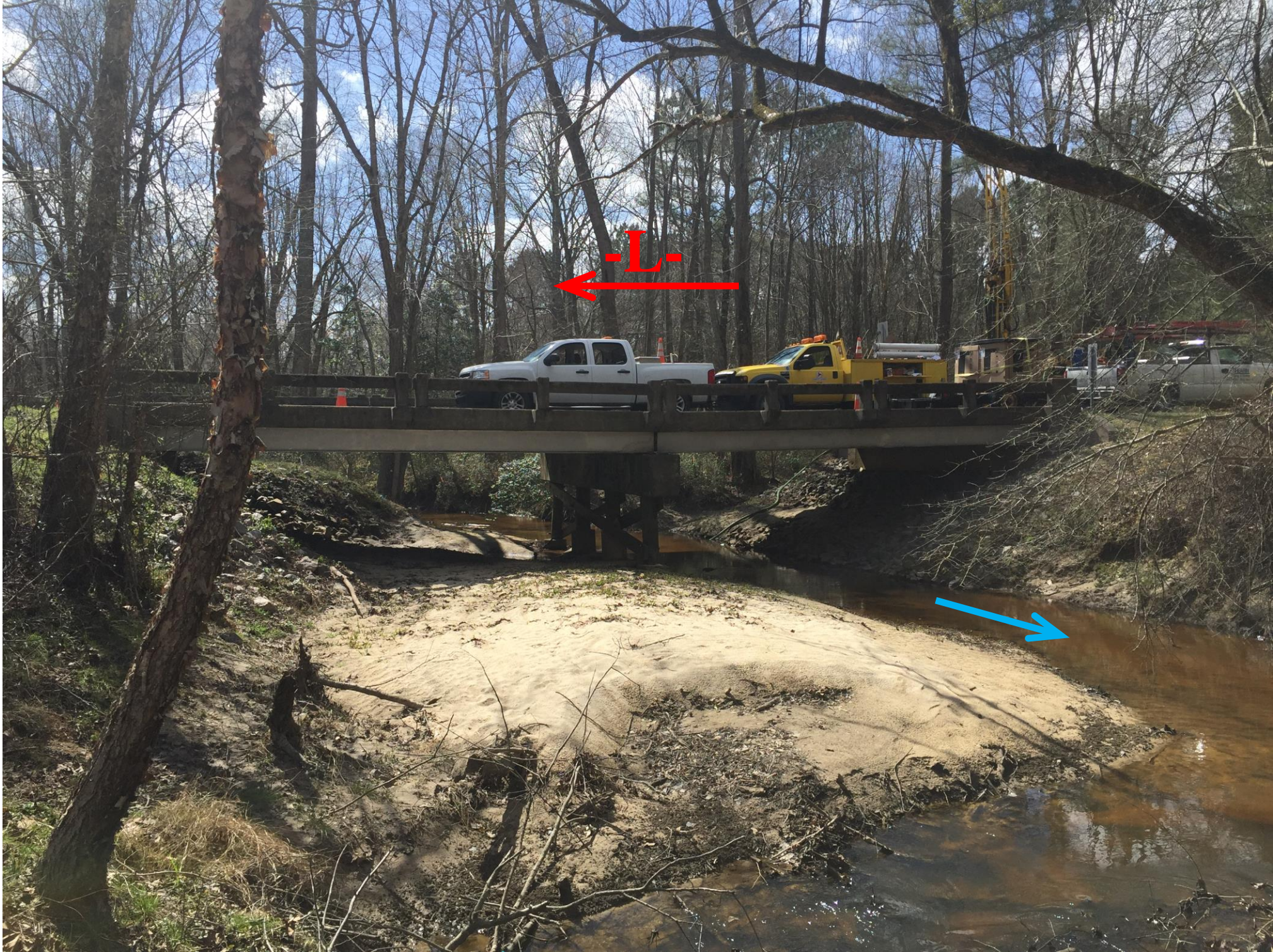
Looking Southwest towards End Bent 1
