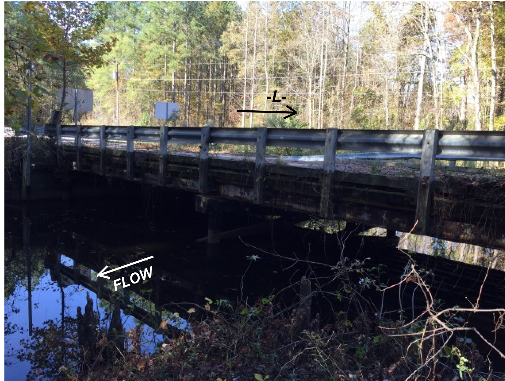
PHOTOGRAPH NO. 1.: VIEW LOOKING WEST
