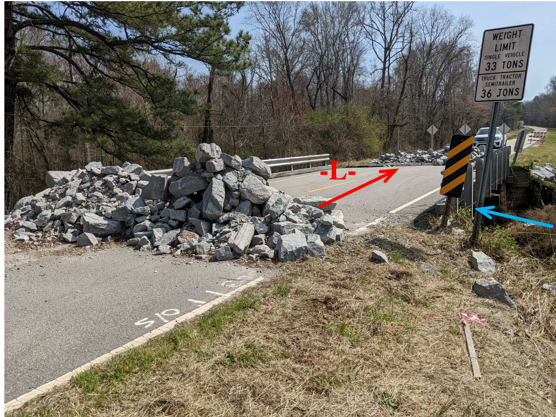
Looking South towards End Bent 2
