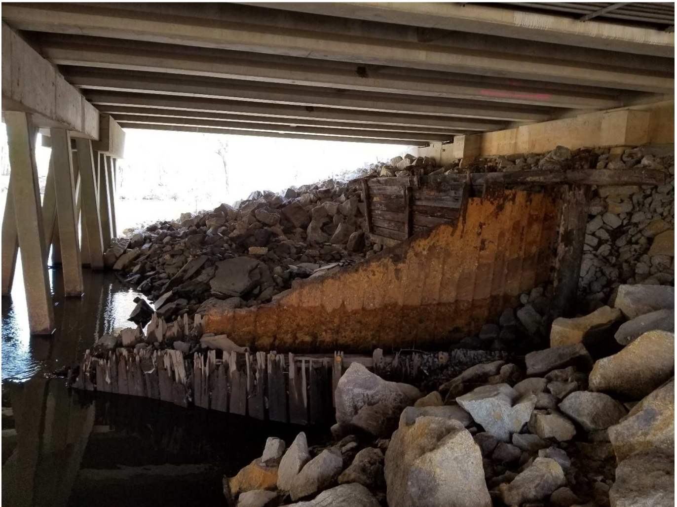
Remnants of old steel sheeting and timber headwall at End Bent 1 to be removed before placing Class II Rip Rap. Lump Sum removal – cutting down as far down as feasible. These remnants contributed to the problem in Hurricane Matthew.
