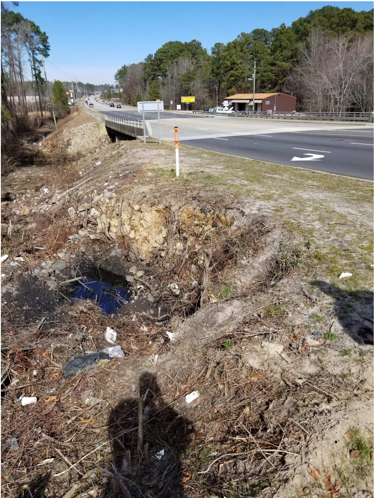
Slope Repair area looking north. Work from this corner for southern end, End Bent 1, work under bridge.
