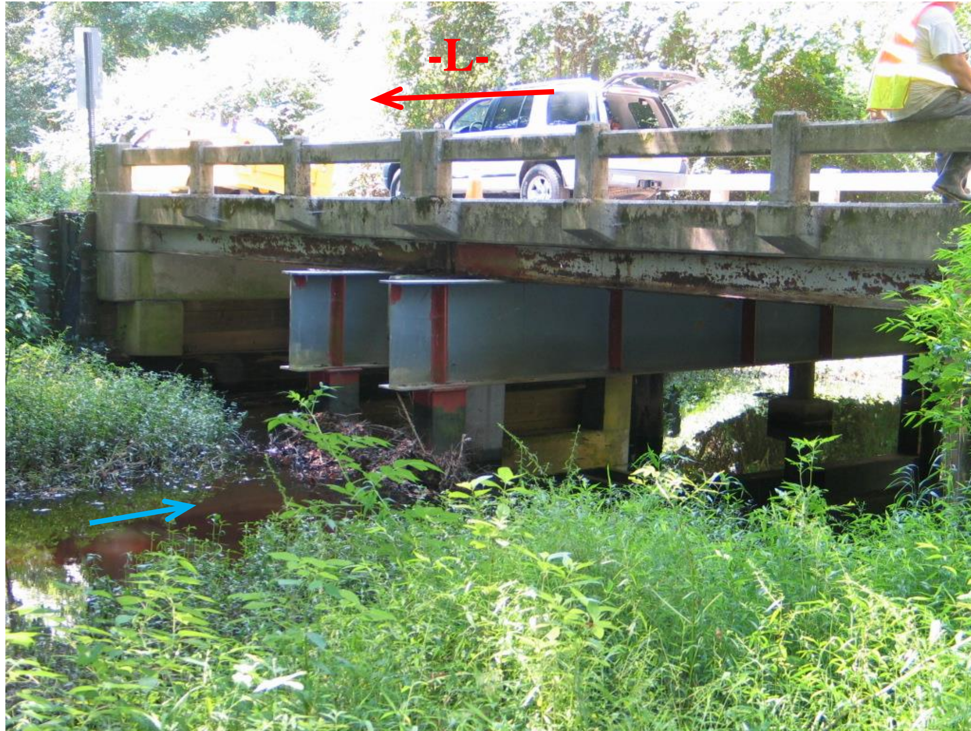
Looking South towards End Bent 2
