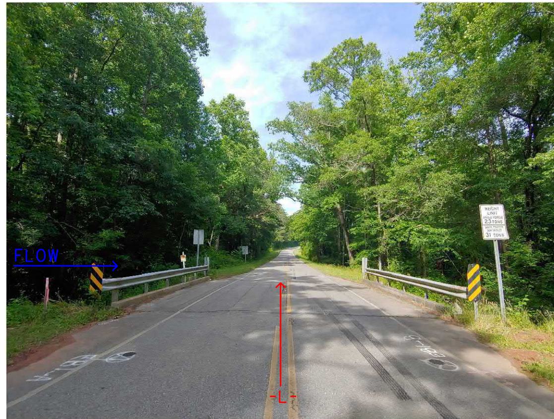
LOOKING EAST FROM END BENT 1 TOWARD END BENT 2
