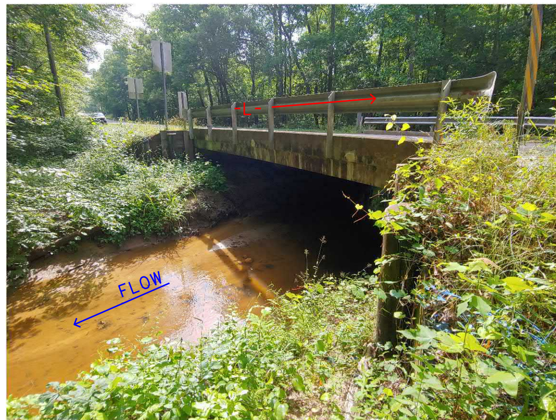
SOUTHEAST OF BRIDGE DOWN STATION TOWARD END BENT 1
