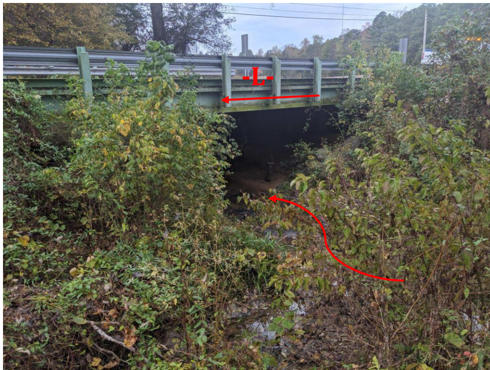
Photograph No. 2: View looking downstream.
