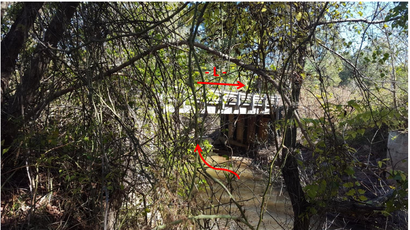
Photograph No. 2: View facing downstream.
