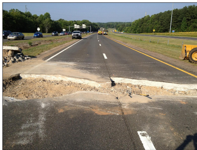
"Pavement buckling" is also known as a blow up or blow out, caused by heat expansion of the concrete slabs. If the joints are not wide enough to accommodate the expansion, the concrete "tents up." It is relatively rare.
