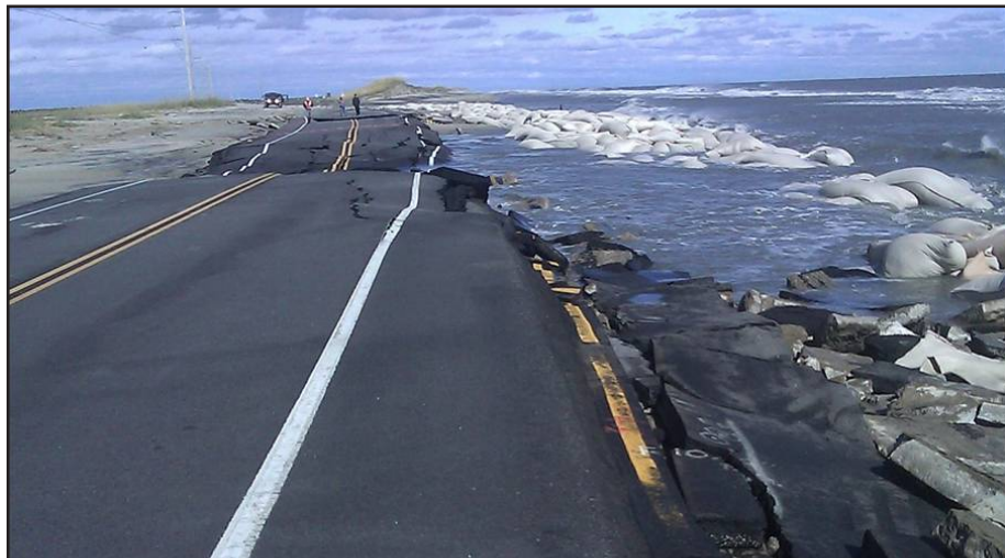
N.C. Highway 12 after Superstorm Sandy wrecked sandbag structures built to protect it. Photo courtesy N.C. Department of Transportation
